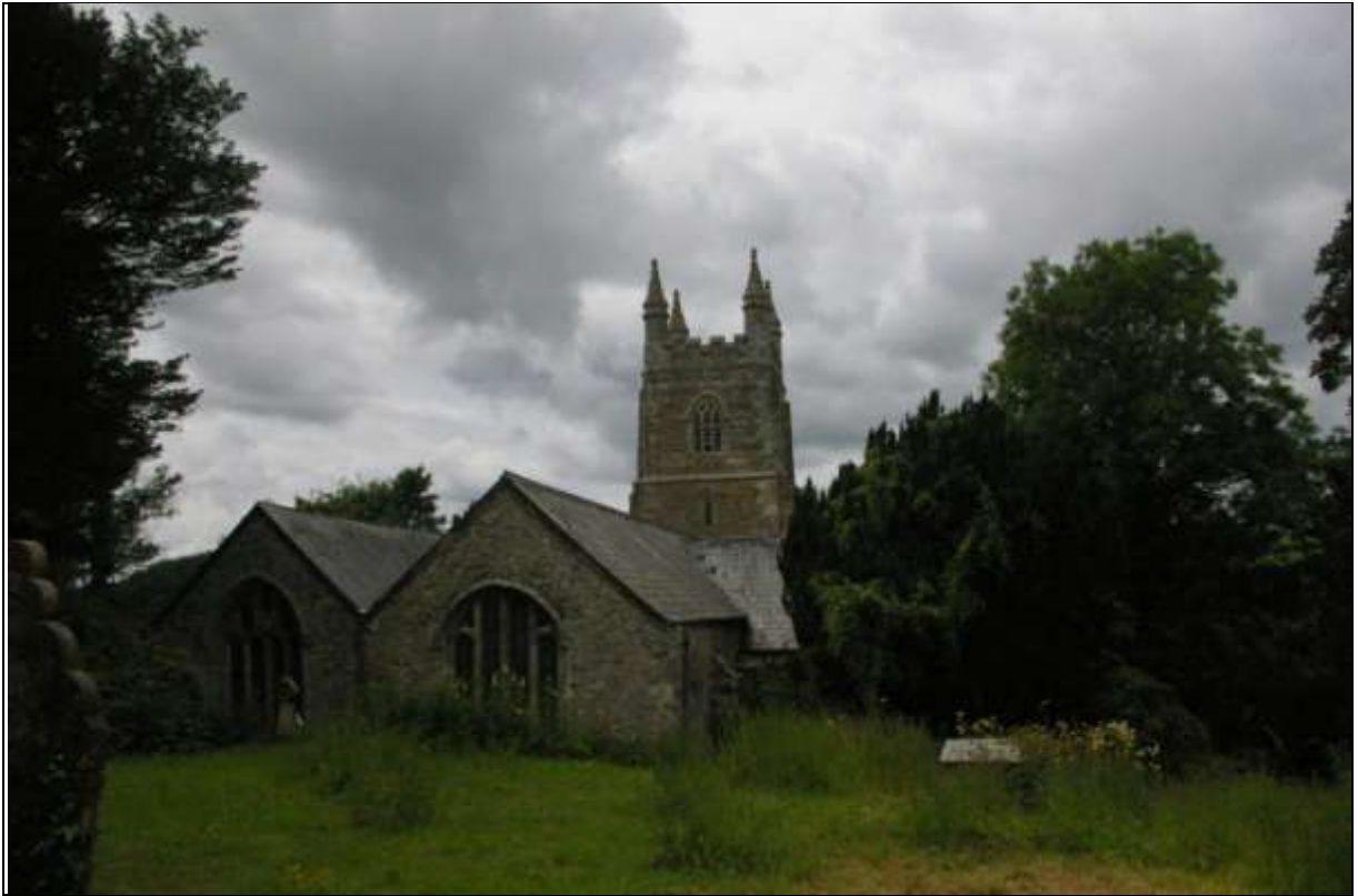
View of St Crida, Creed, within its enclosed churchyard; from the east-north-east.
