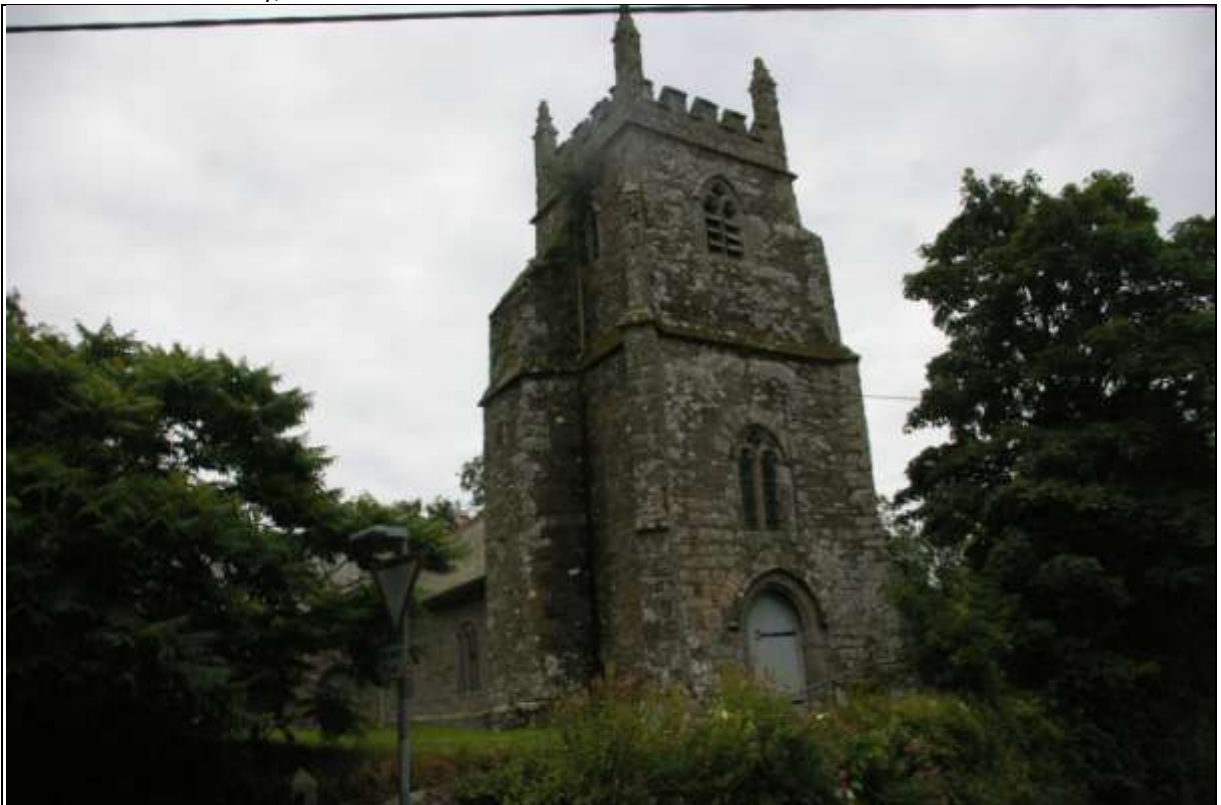
Church of St Cuby in Tregoney; viewed from the north-west.
