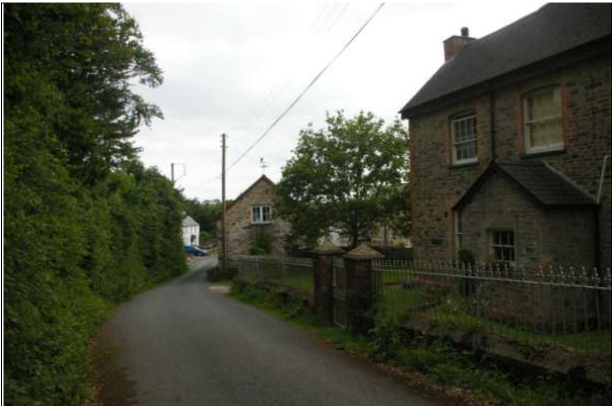
Barns and stables approx 50m south of Westacott House; from the north-north-west.
