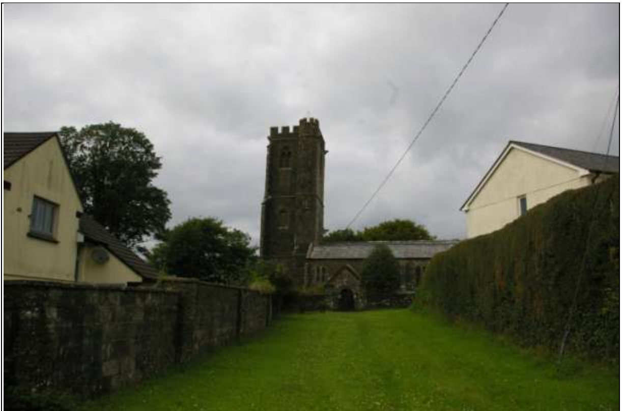
Church of St Bartholomew, Stoke Rivers and archway and gatepiers to churchyard; from the south.
