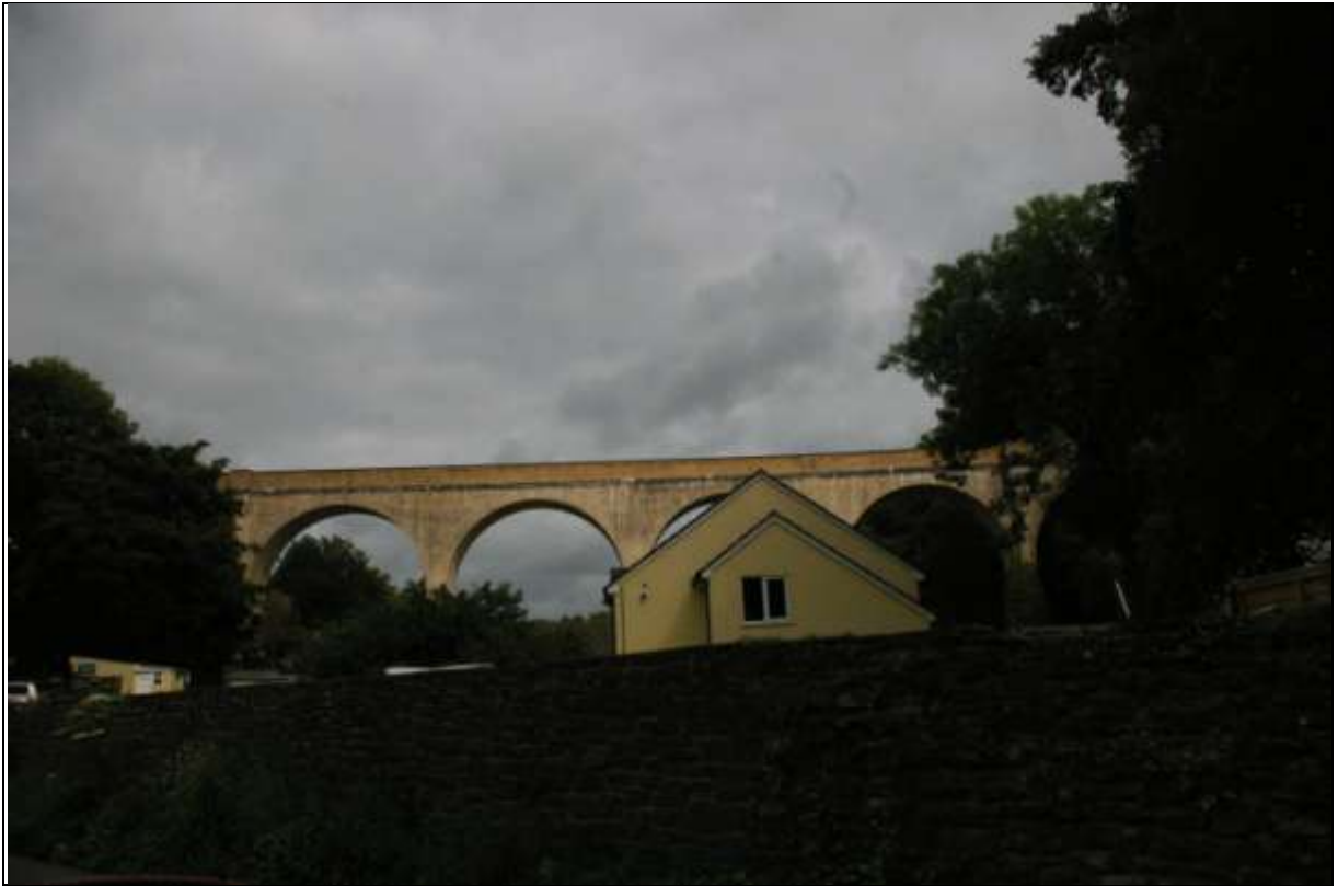
Chelfham Viaduct, Grade II Listed, where a tributary joins the River Yeo valley; from the west-south-west.
