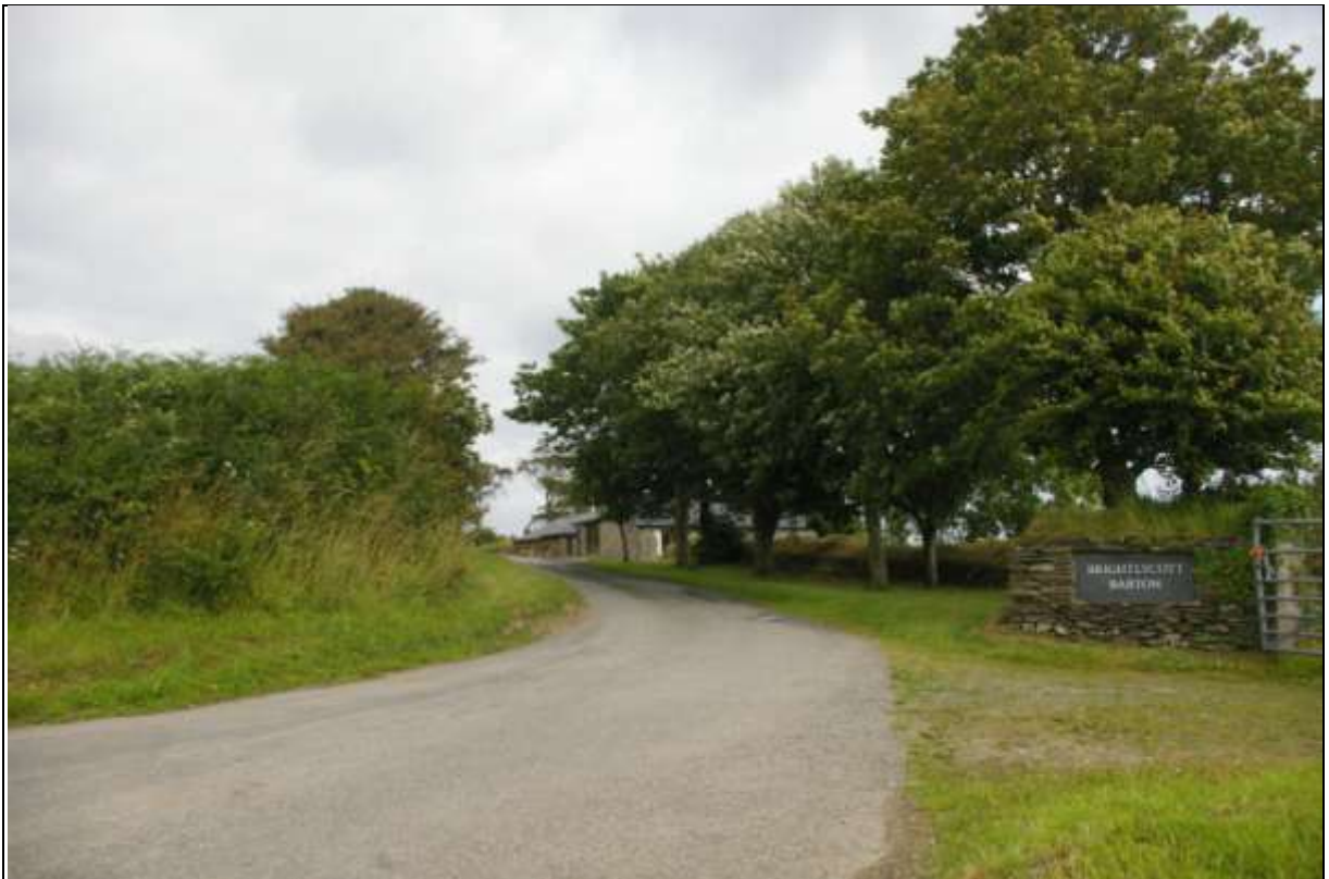
Brightlycott Barton, the closest asset to the proposed turbines, Grade II Listed; from the west.
