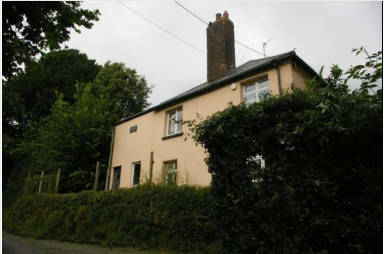
Westacott House, in Westacott, adjacent to Barnstaple; from the south-south-west.
