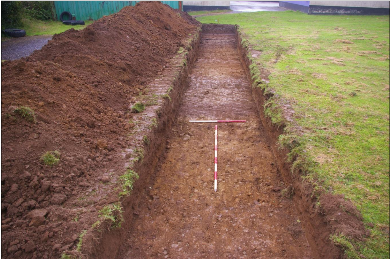
Figure 4: Trench #1, showing ditch [103] pre-excitation; viewed from the north-west (scales 1m and 2m).
