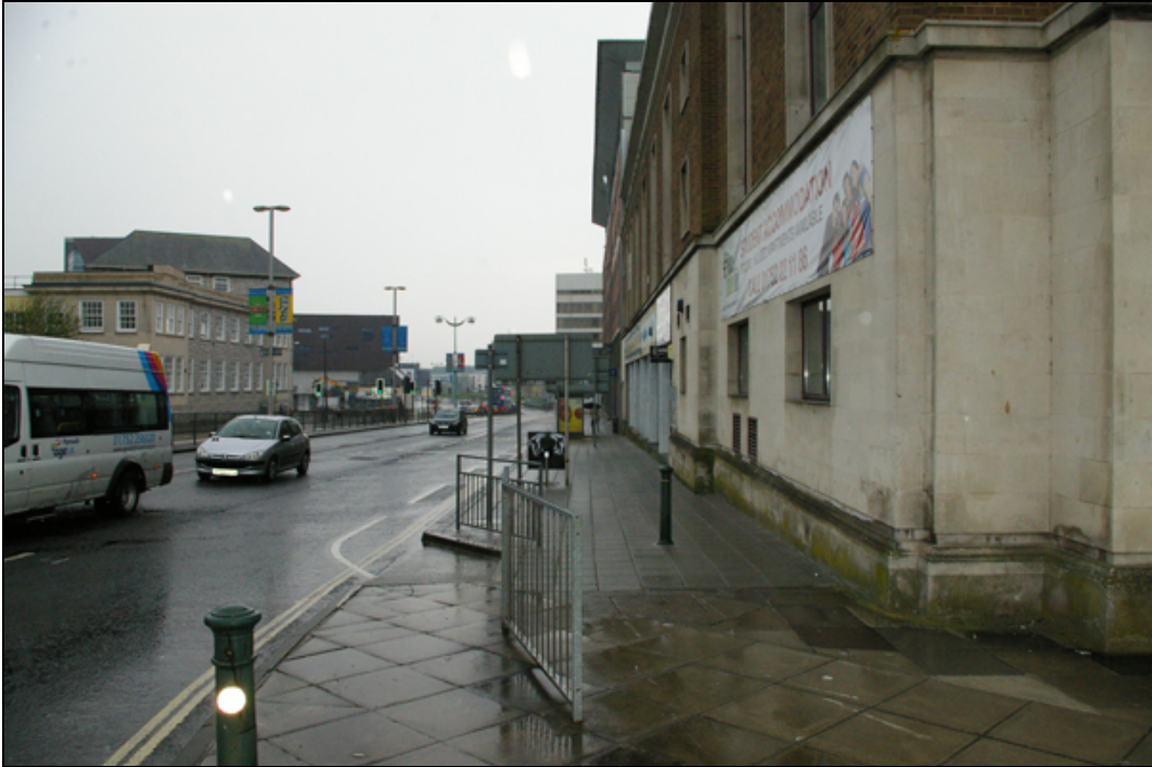
Figure 16: View along Cobourg Street with Beckley Court on the right and Reynolds Building on the left, viewed from the north-west.
