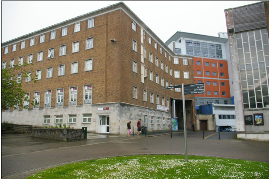
Figure 11: Beckley Court, viewed from the south-west.
