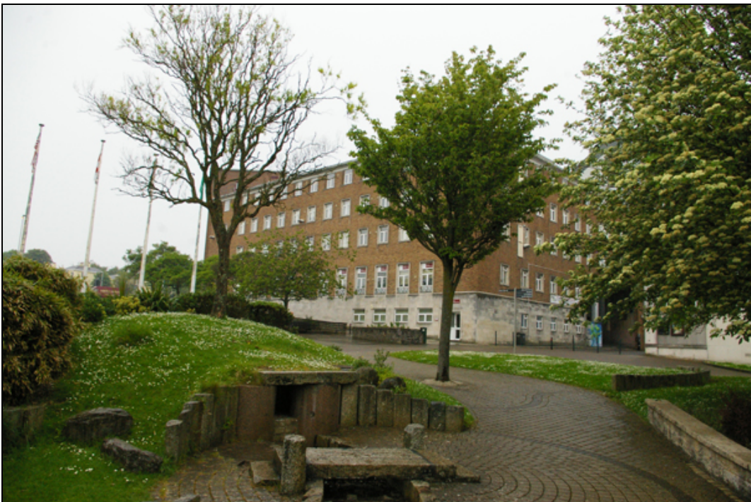
Figure 15: Beckley Court viewed from Armada Way, viewed from south-west.
