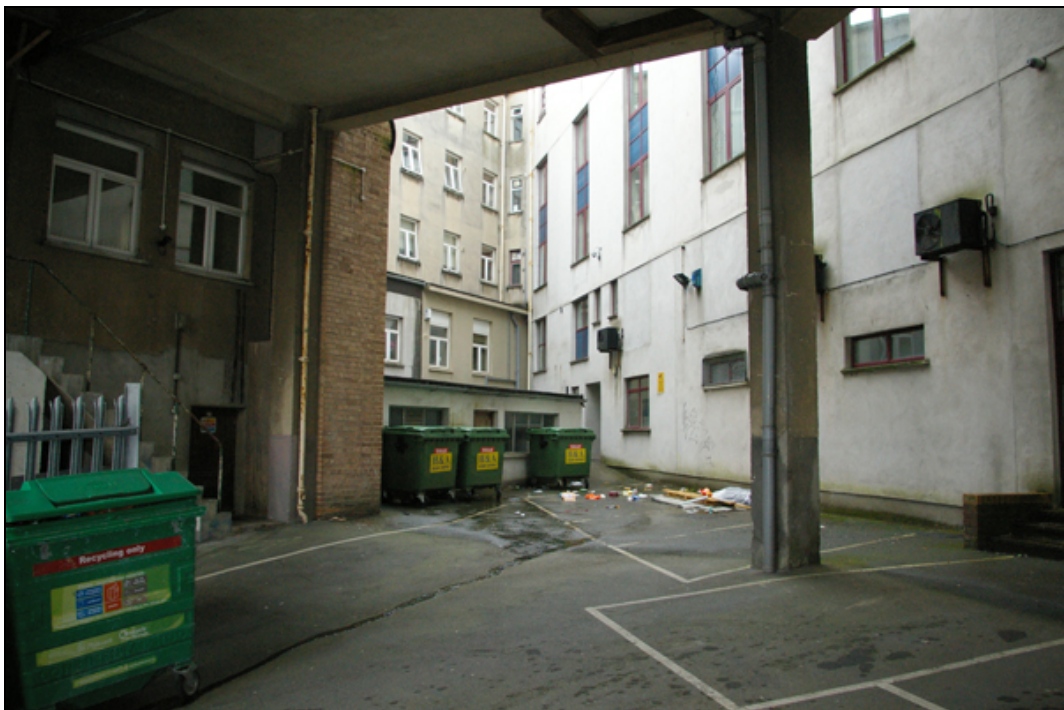
Figure 12: Inner court of Beckley Court, viewed from the south-east.
