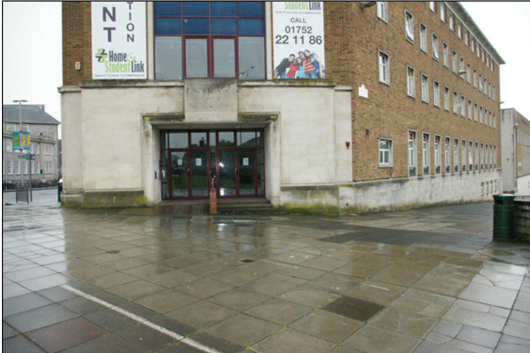
Figure 13: Front of Beckley Court, viewed from the north-west.
