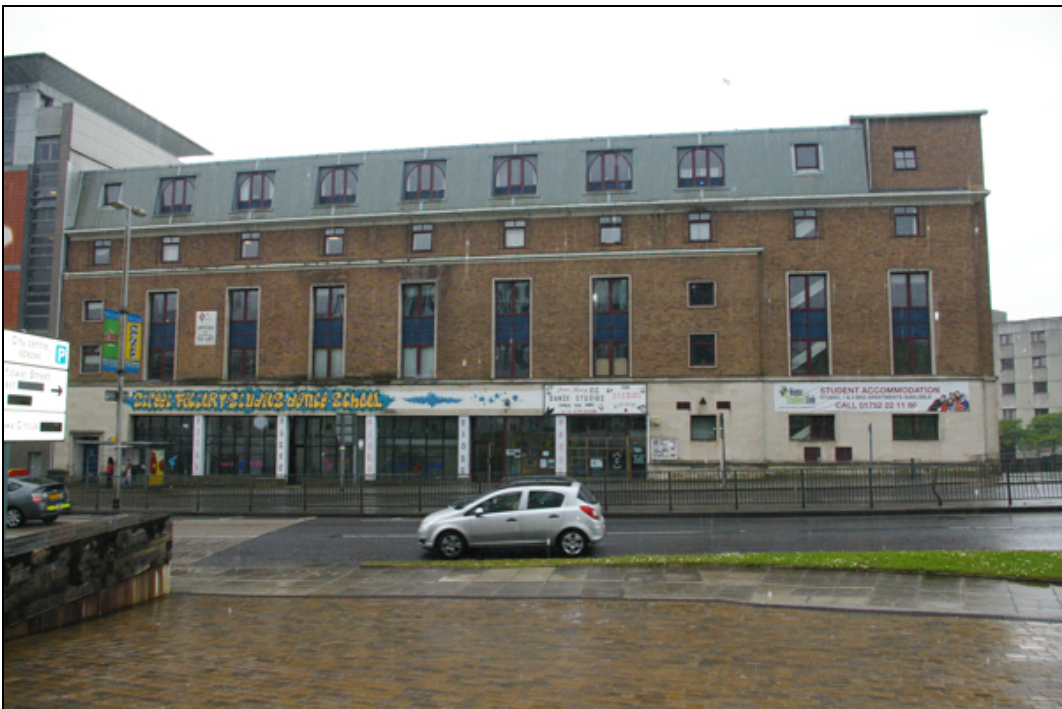
Figure 17: North-east facing elevation of Beckley Court, viewed from the north-east.
