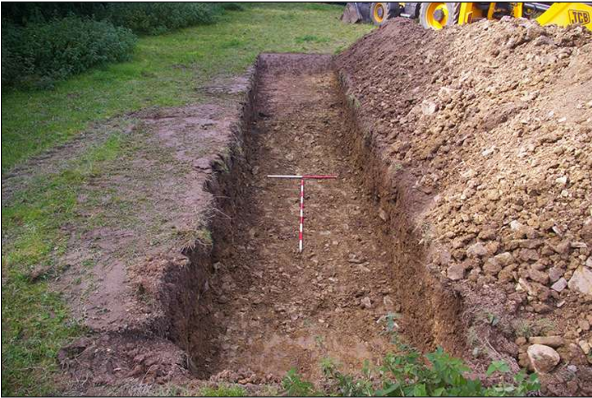
Plan view of Trench #2; viewed from the east (1m and 2m scales).
