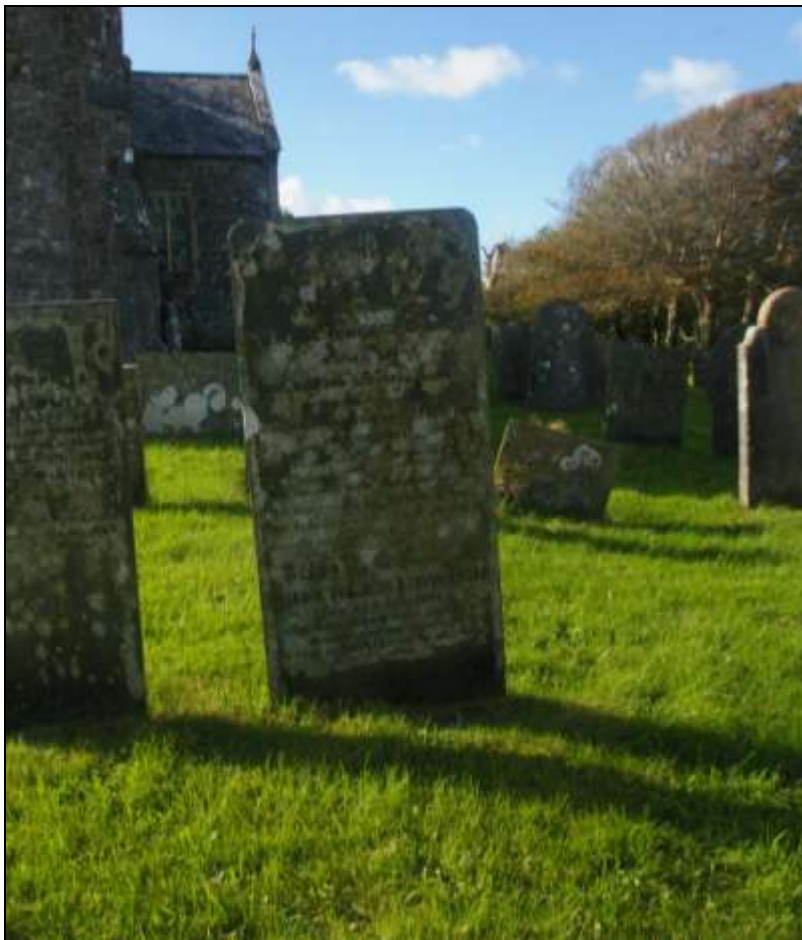
The Galsworthy headstone, a Grade II Listed structure in the churchyard; from the east-south-east.
