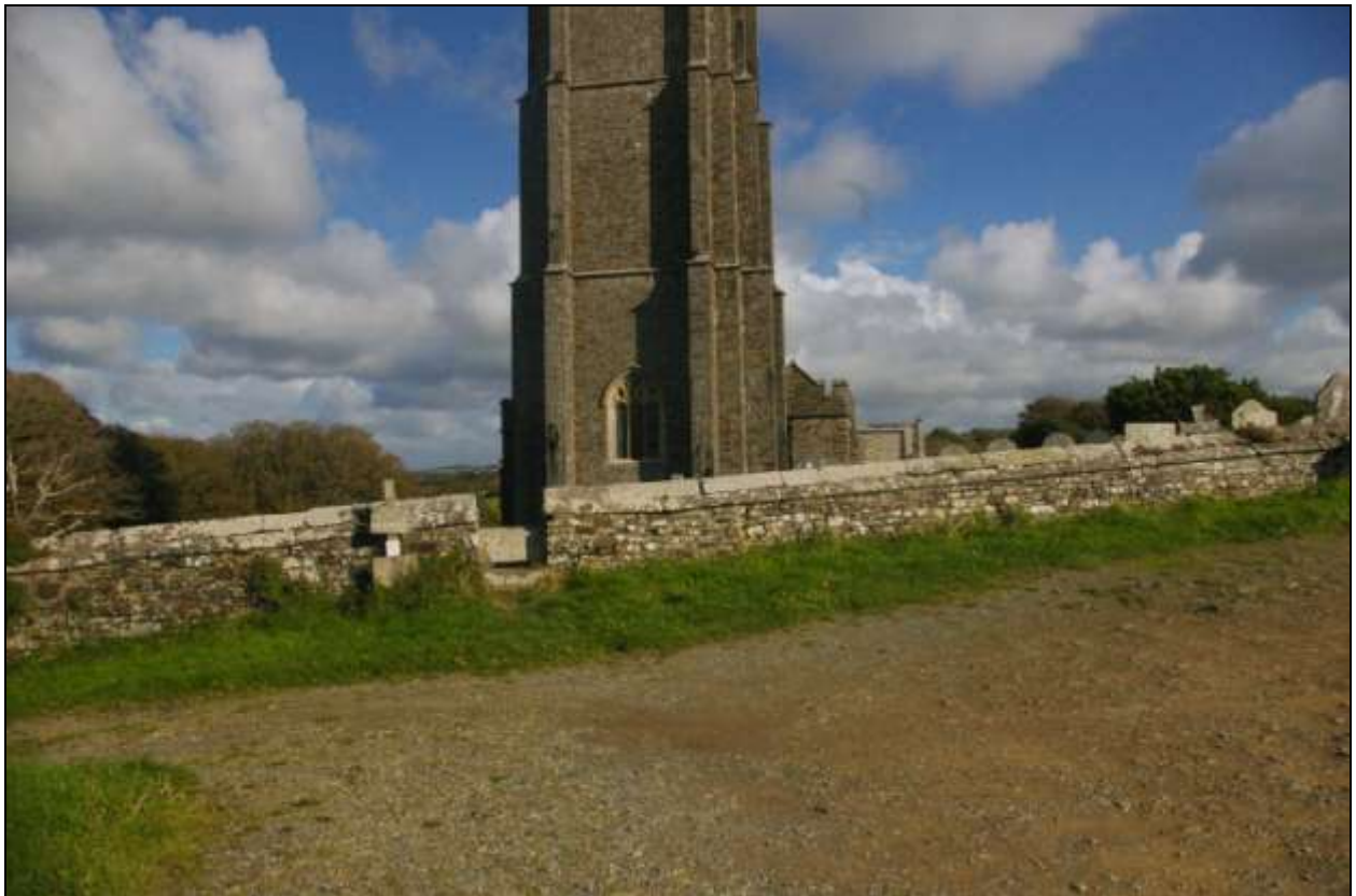
The churchyard wall, with two stiles; viewed from the west.
