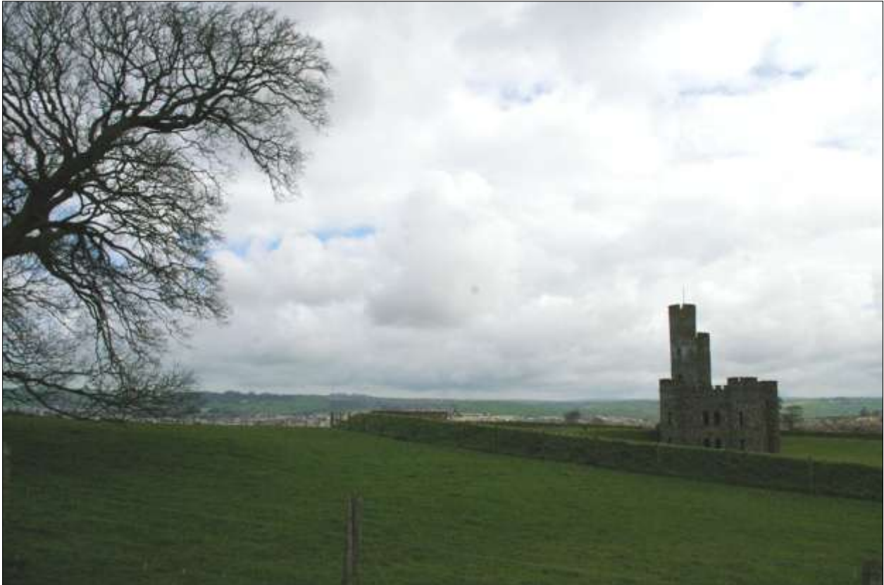
Close up of 'The Tower' from previous report; from the south-west.
