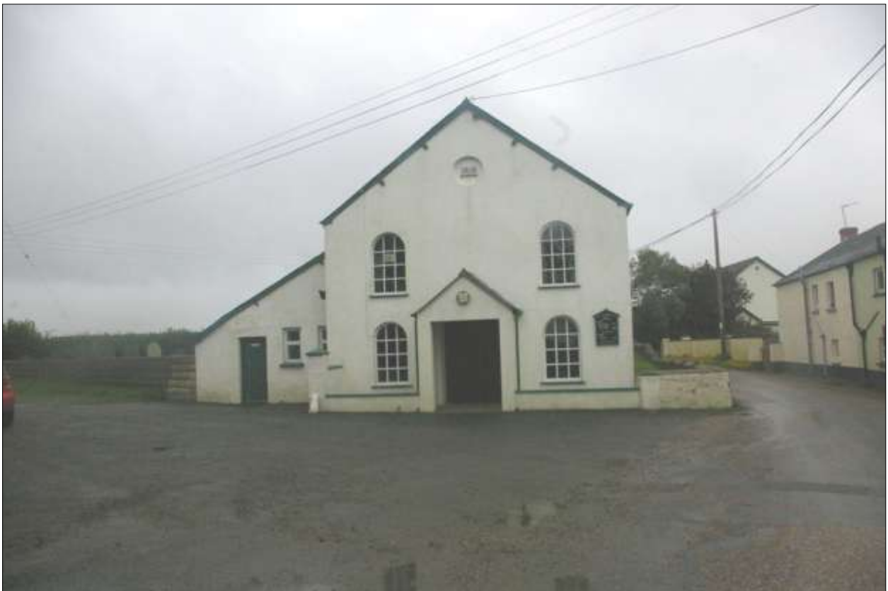
View of the chapel at Eastacombe; from the west-south-west.
