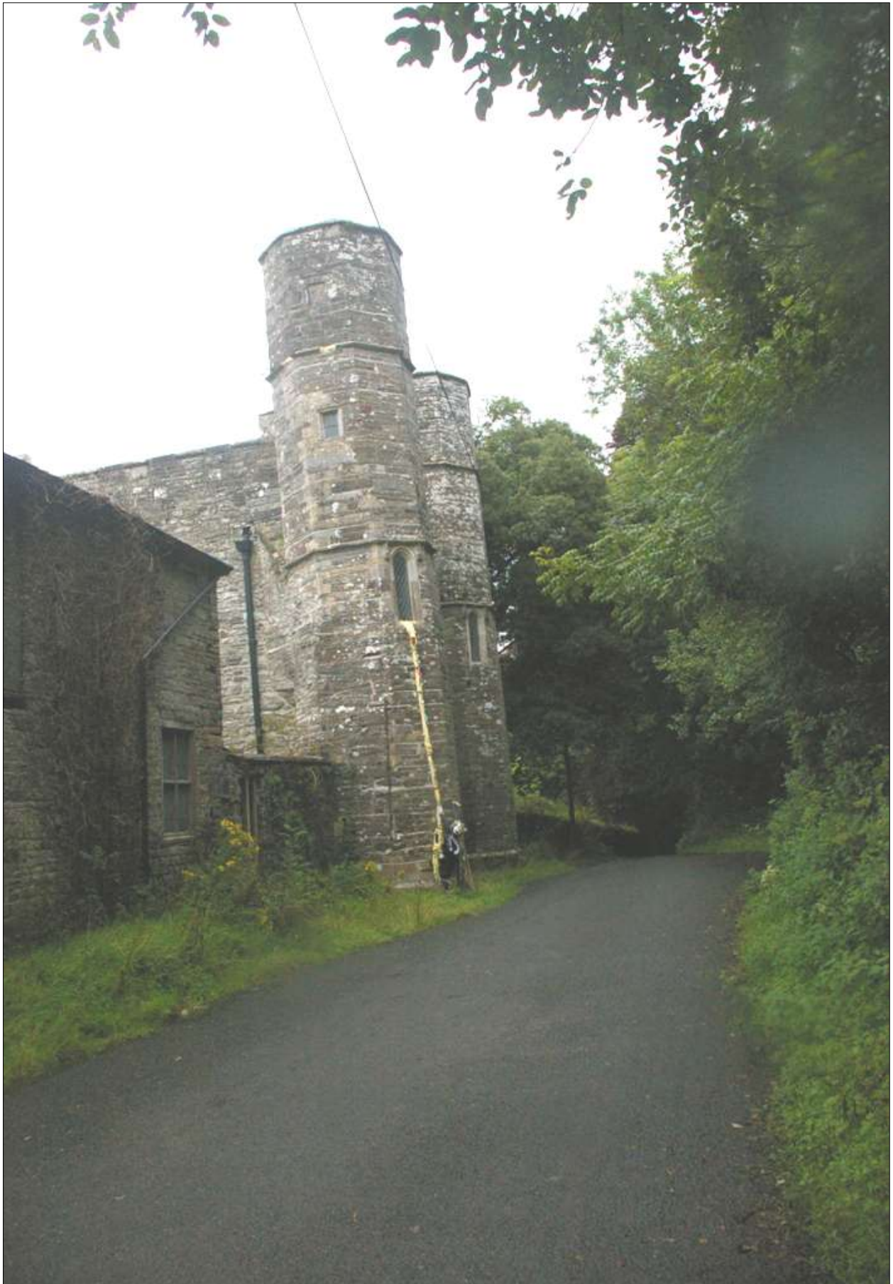
View of Tawstock Court Gatehouse; from the west.
