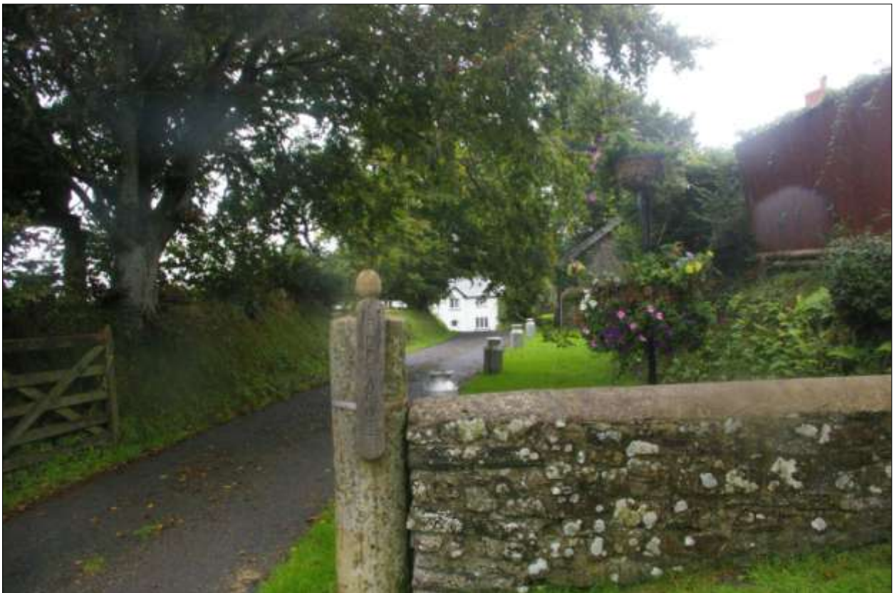
Lower Uppacott, set into the slope, facing west; from the west.
