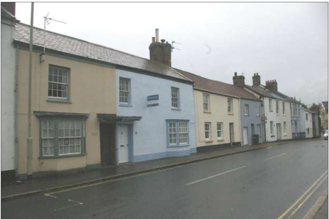
View of GII Listed cottages, along South Street in Newport; from the north-west.
