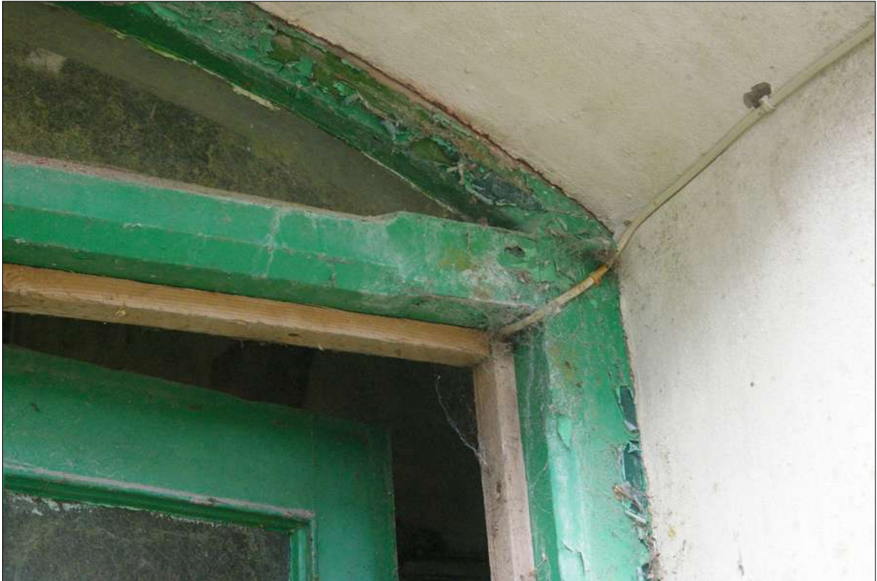
Heavy chamfered frame with arched single pane of glass above; from the south-east.
