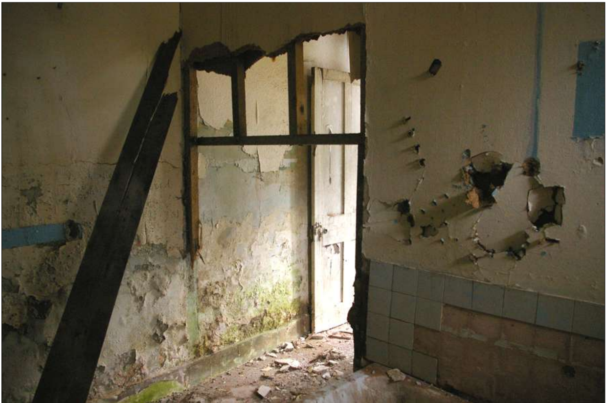
Room 7, the modern timber framed partition; from the south-west.
