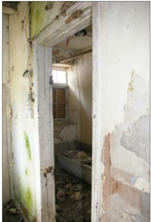
Left: Room 2, a secondary part of the lobby, showing doorways 3 and 4 and surviving skirting boards; from the south. Right: The bathrooms of Room 7. The modern partition cuts the transom timber window, which is the same as that Rooms 4 and 6; from the north-east.
