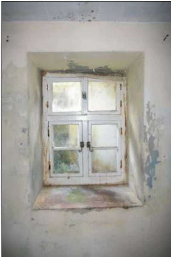
Left: The window in Room 9. A heavy timber transom, with fixed single-pane opening casements above and two-pane opening casements below. The window has brass locks and coiled latches; from the south.
