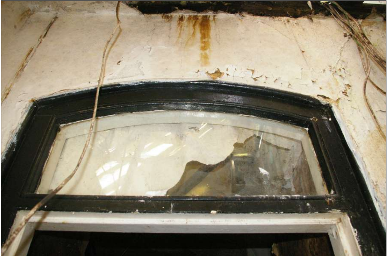
Detail of door between Rooms 14 and 15, with its narrow beaded frames instead of the chamfered frames seen elsewhere in the building; from the west.
