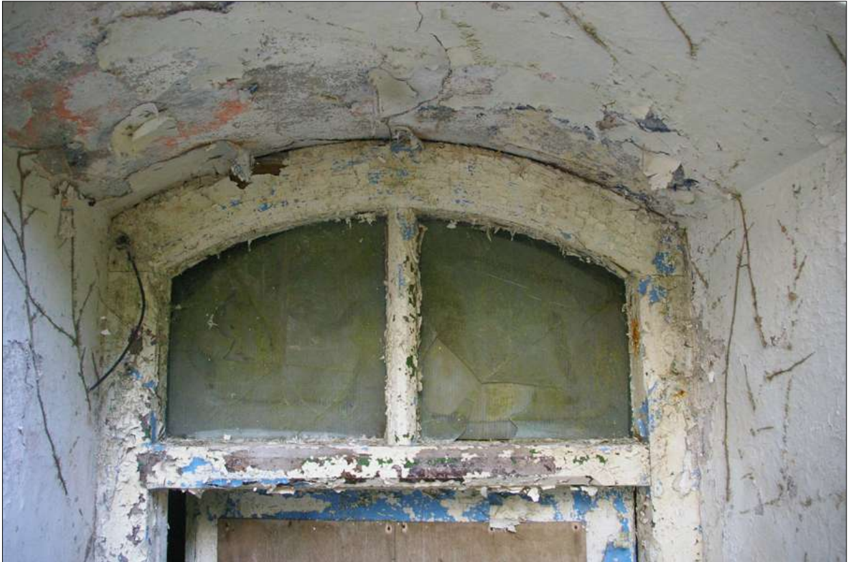
Heavy chamfered frame with two-pane mullioned arched light above; from the west.
