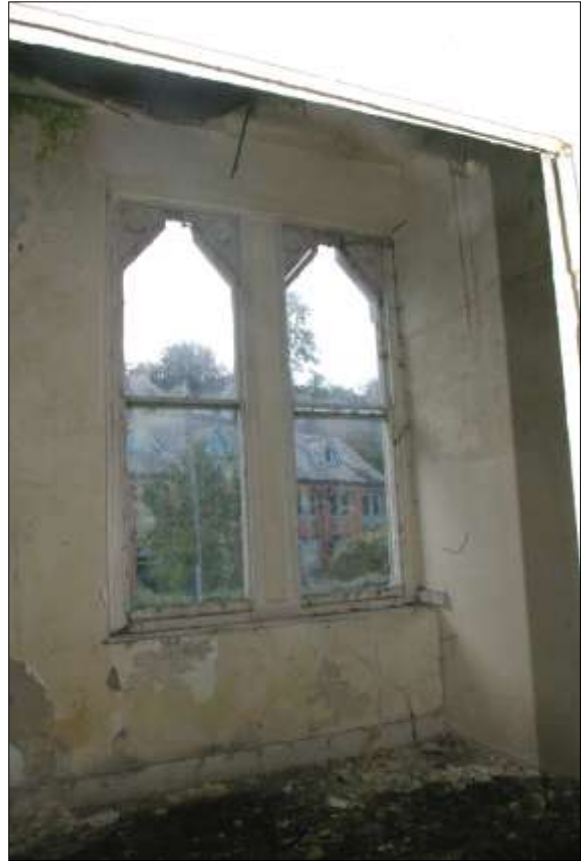
Right: Room 20, showing a modern partition cutting the three-light sash window; from the north-east.
