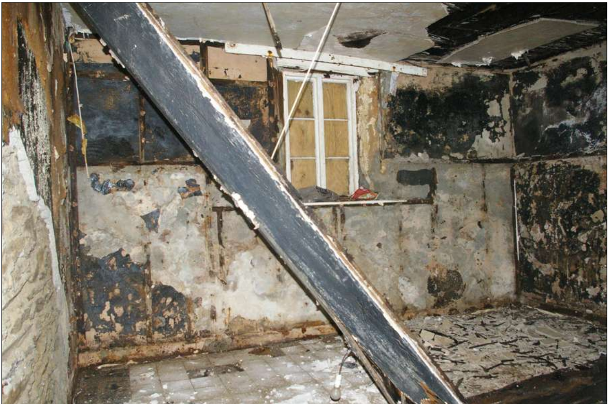
Room 14, showing excessive water ingress and damage; from the south-west.
