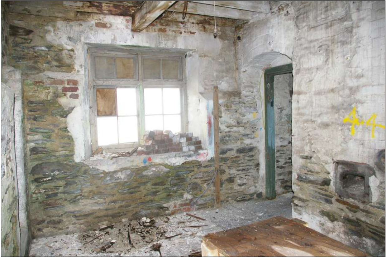
Room 6, the former coal chute and boiler room, with a further timber transom window, as in Room 4, and exposed stone walls; from the north-east.
