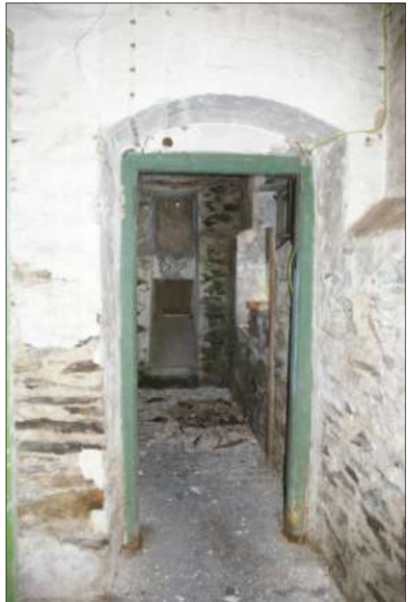
Right: Brick segmental arch; to Room 6, the former coal chute and boiler room; from the west.
