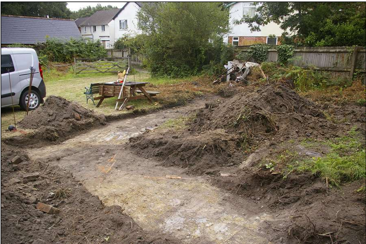
FIGURE 3: GARAGE FOOTING AREA; VIEWED FROM THE NORTH-WEST (NO SCALE).
