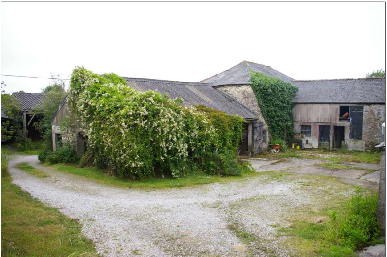
B4 and B5, viewed from the north-west.
