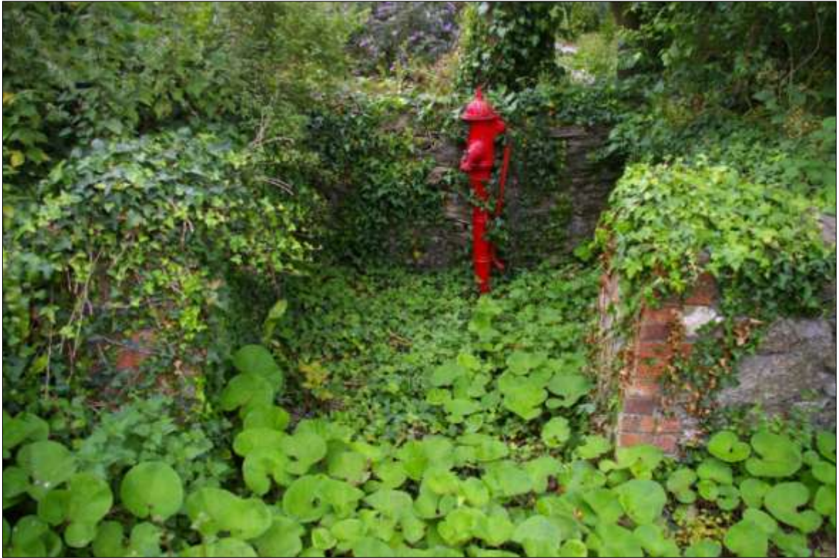
Figure 17: The walled pump at the southern end of the site; viewed from the west.
