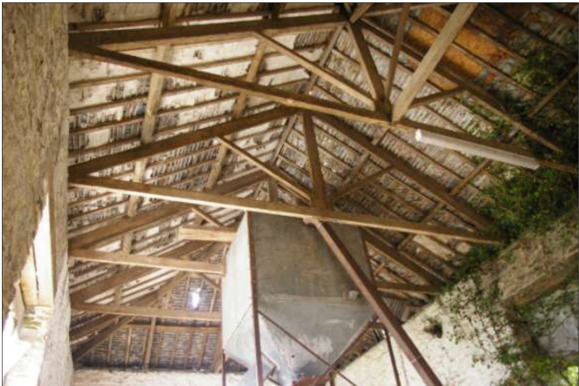
Figure 15: The interior of B4, showing the kingpost with queen-strut roof.
