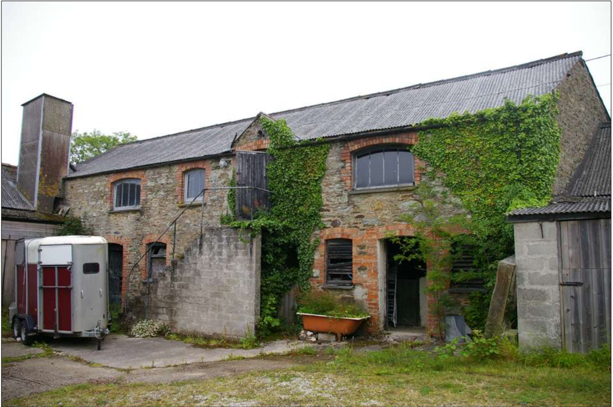
Detail of the east elevation of B2; viewed from the north-east.
