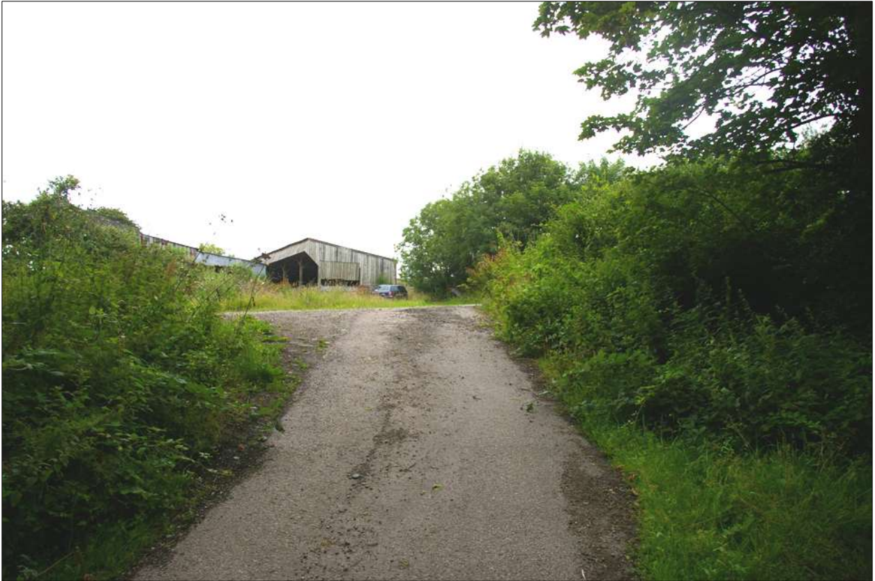
View up one of the new access drives, showing B9; viewed from the south.
