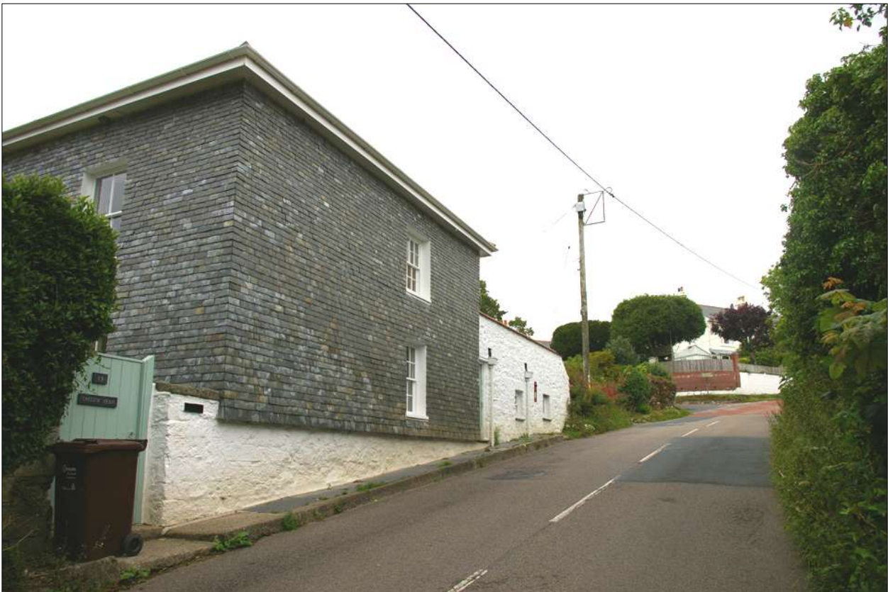
No. 19 Tregew Road, the roadside elevation viewed from the south-east.
