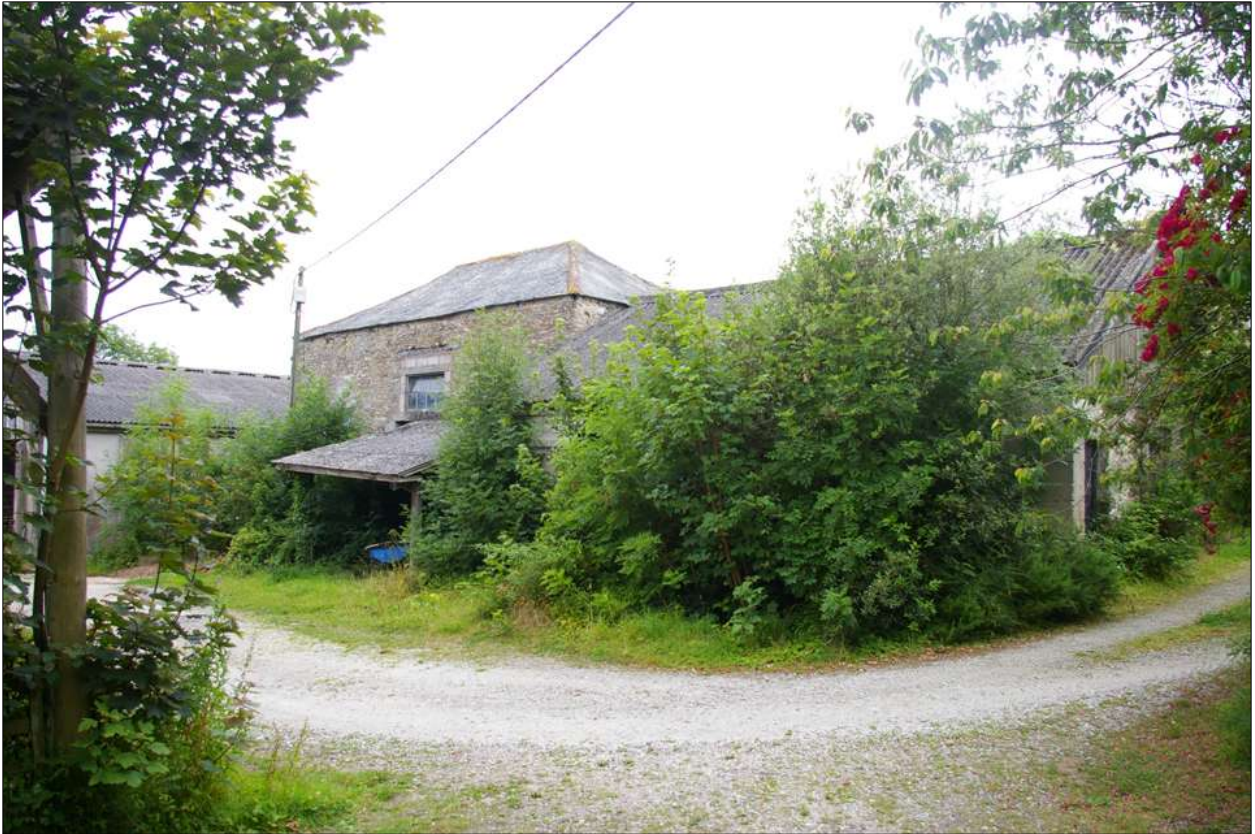
The east elevation of B4 and B5, viewed from the north-east.
