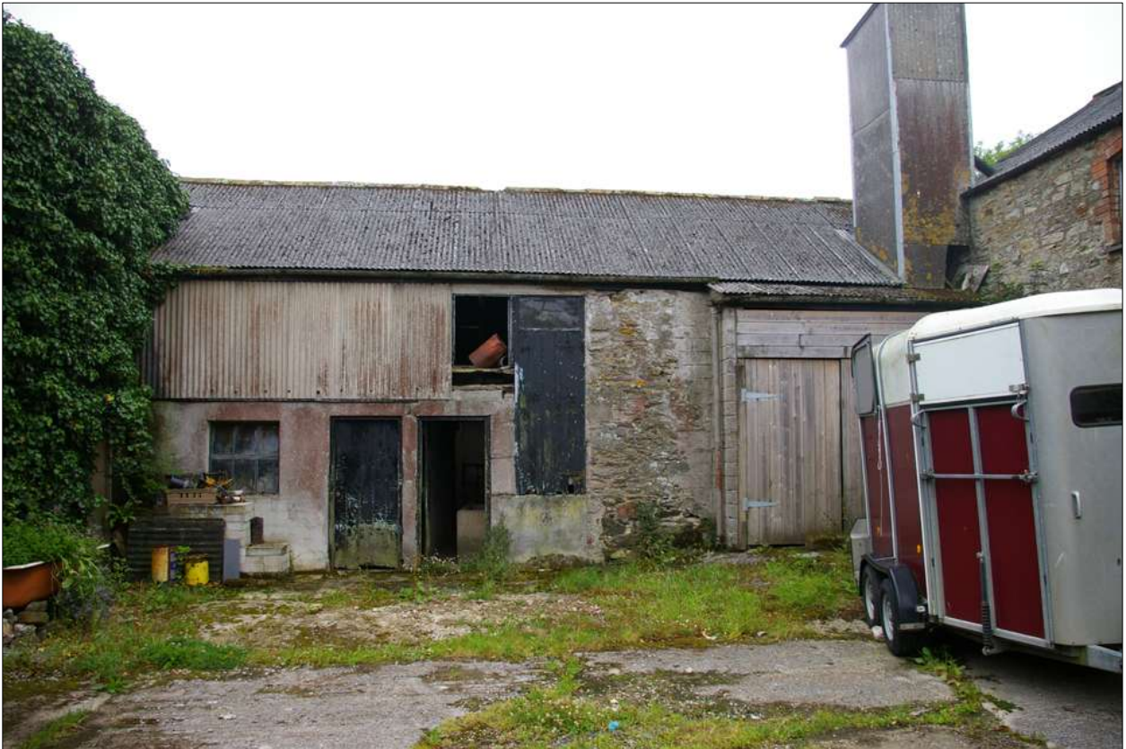
Detail of the north elevation of B3; viewed from the north.
