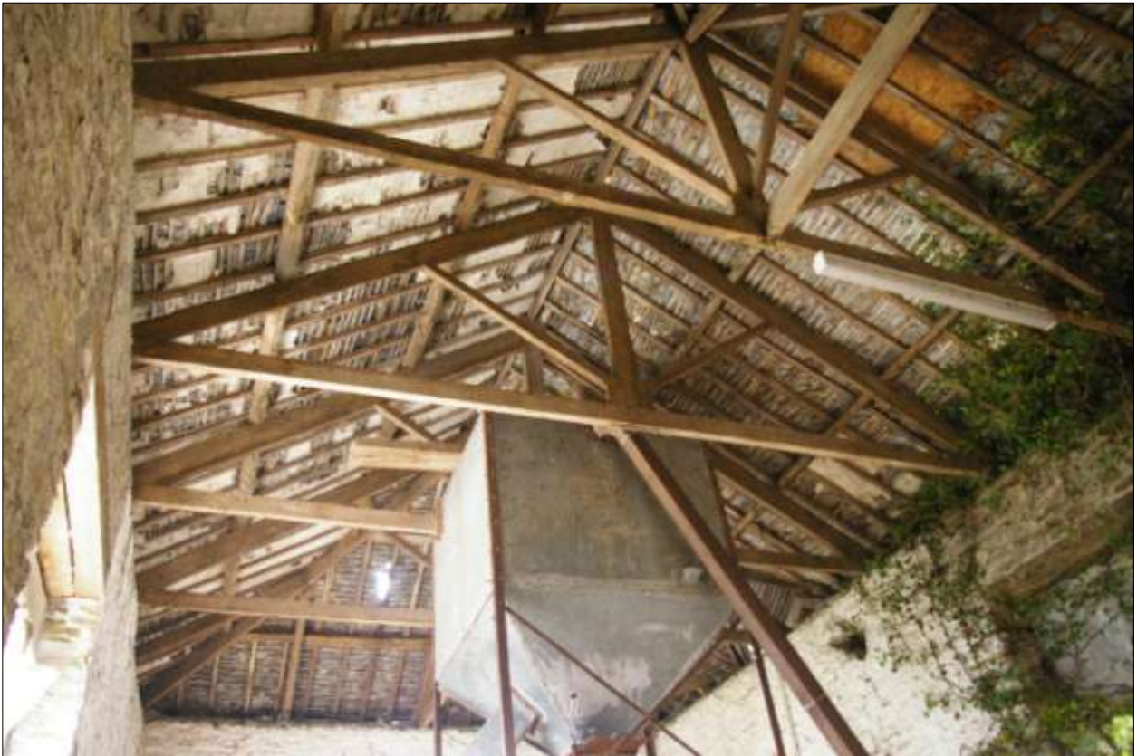
The interior of B4, showing the kingpost with queen-strut roof.
