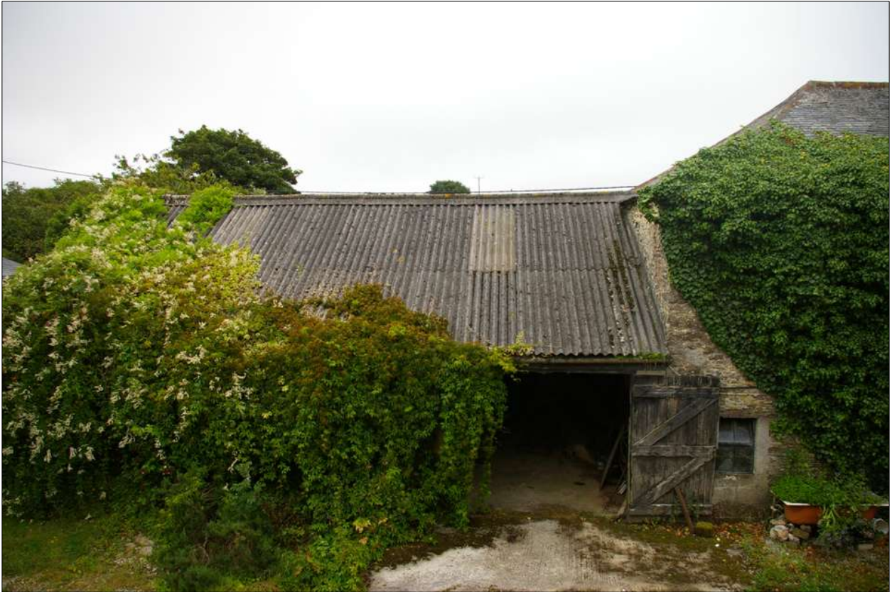
Detail of the west elevation of B5; viewed from the west.
