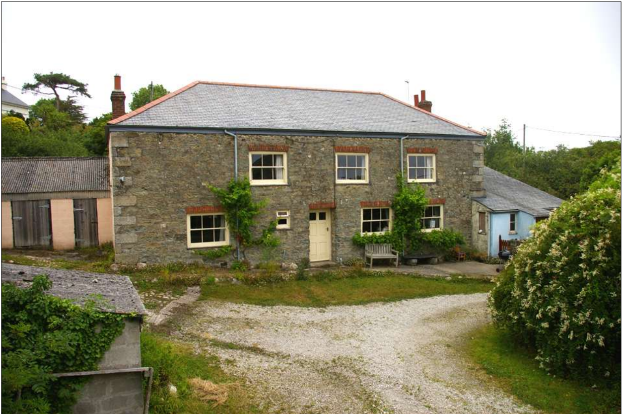
The south elevation of the farmhouse, viewed from the top of the steps outside of B2; viewed from the south-west.
