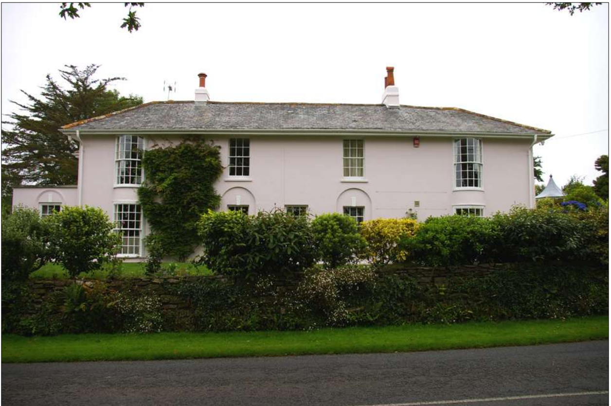
As above; viewed from the south-east.
