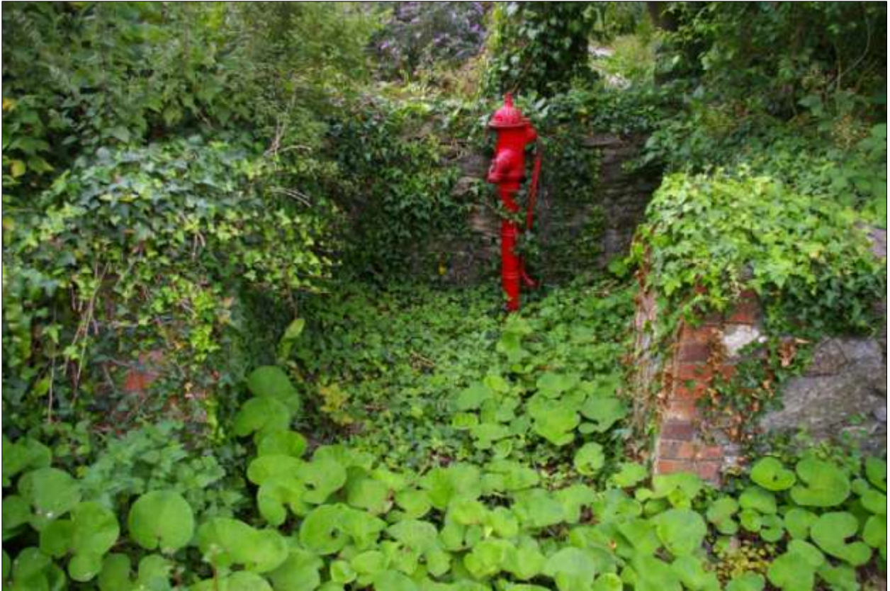
The walled pump at the southern end of the site; viewed from the west.
