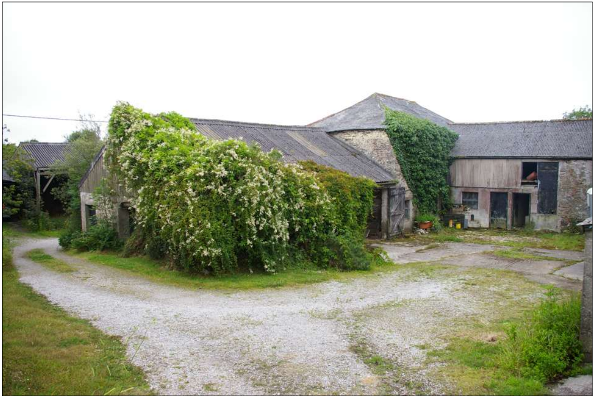
Figure 14: B5 (centre) and B4 (right), viewed from the north-west.
