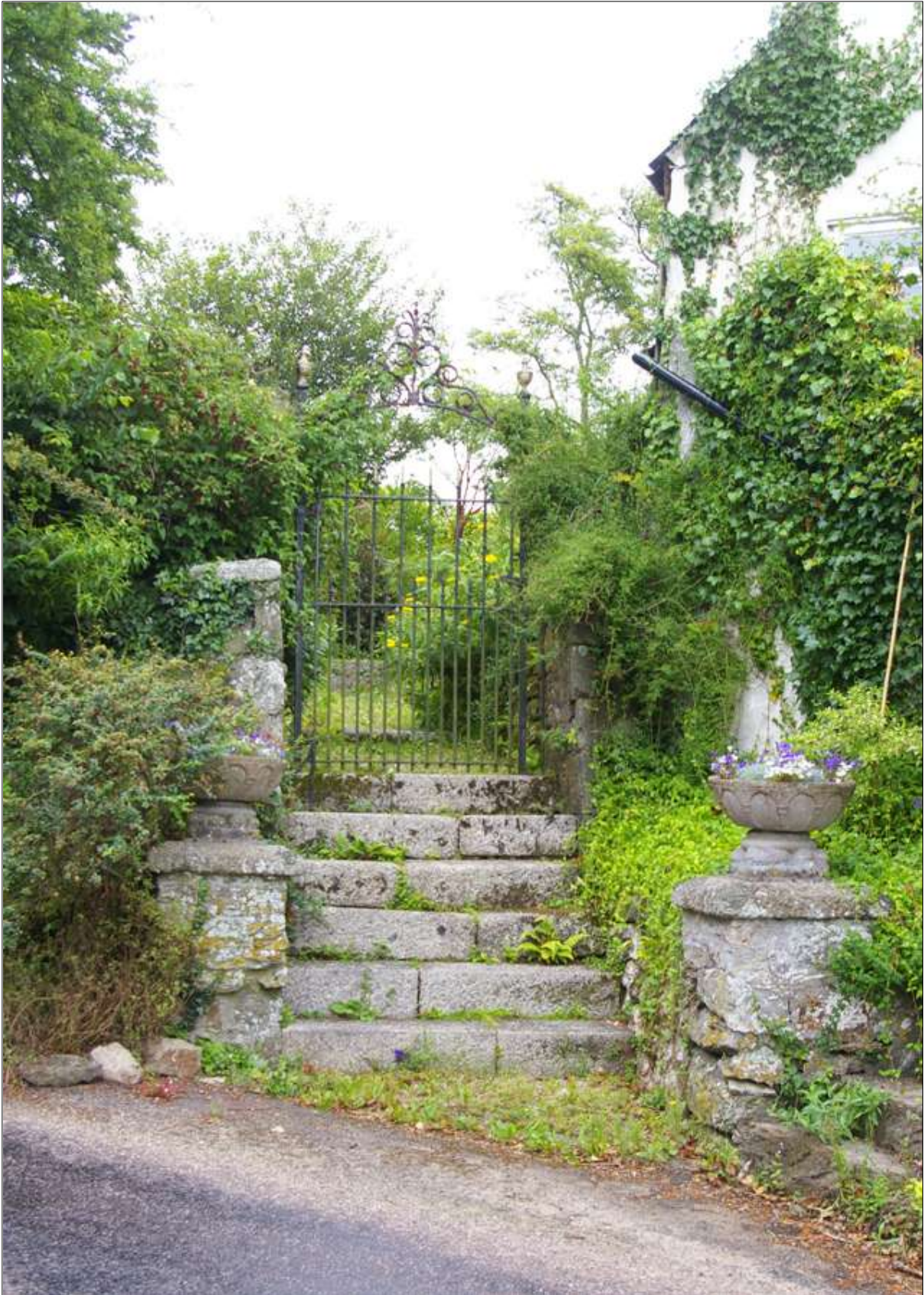
The GII steps/gate piers to Tregew House; viewed from the south.
