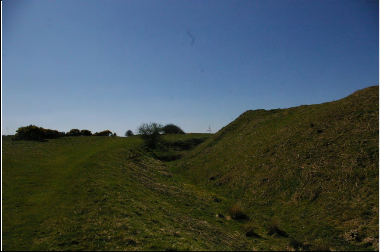
Shot across the outer ramparts at Warbstow to the Tredarrup turbine to the south-west; viewed from the east.
