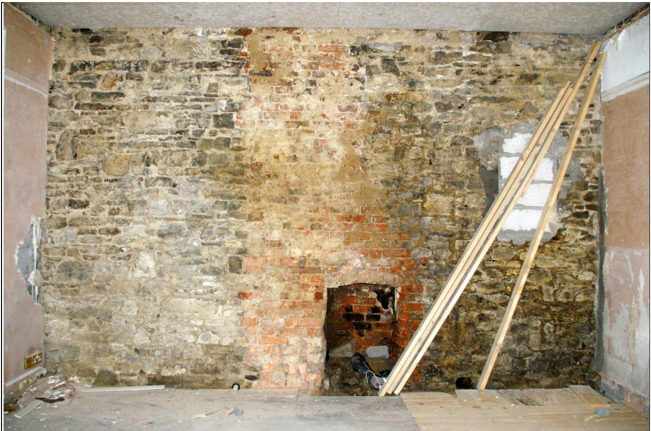
The small fireplace and blocked window or alcove in the west wall in the front bedroom to the left in the Manor House; from the east.
