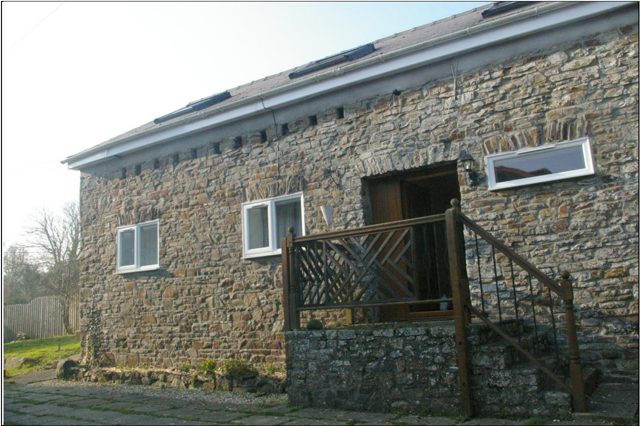
The outbuilding to the north of the Manor House; from the south-east.
