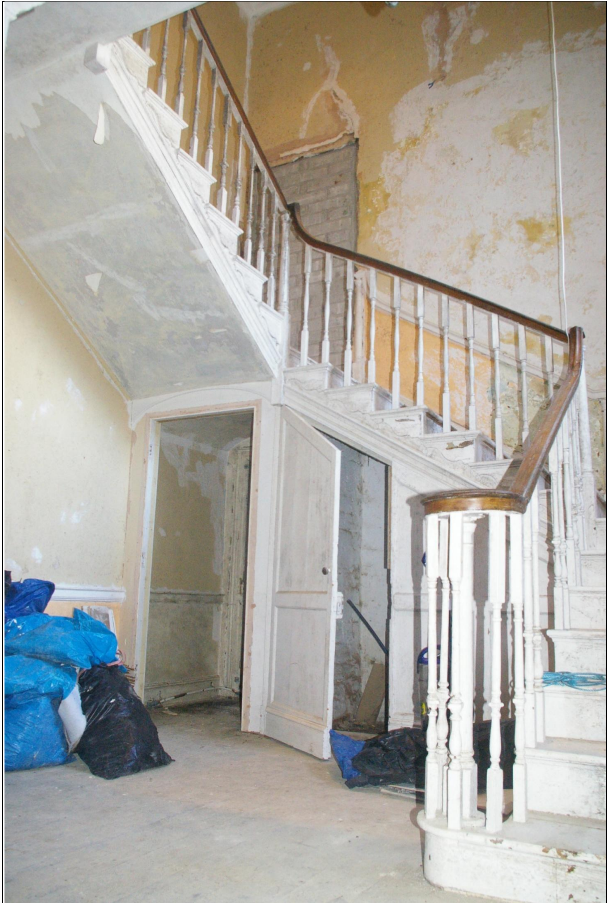
The stair in the Manor House; from the south-east.
