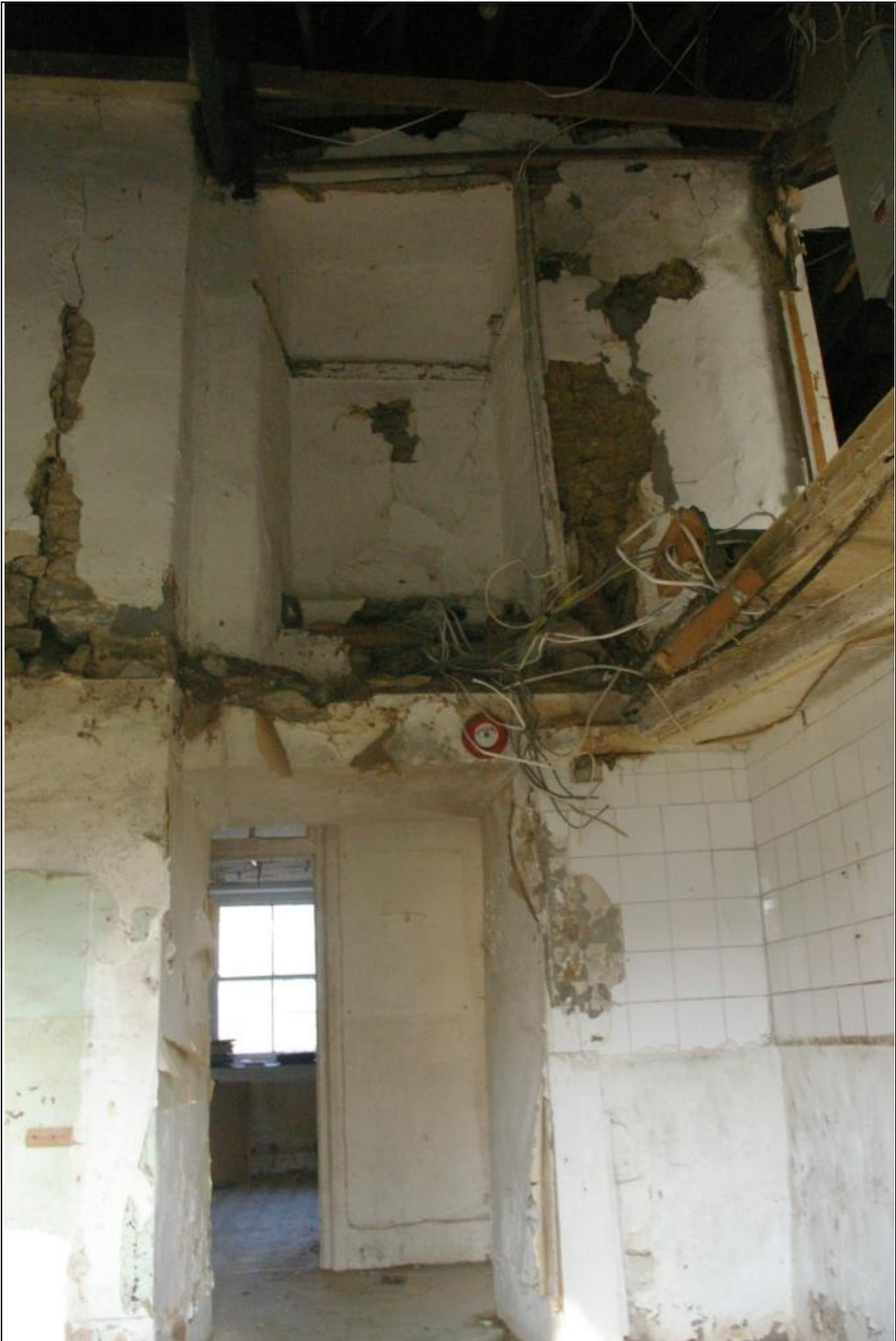
Two doorways within the lean-to, one to the former cross-passage on the ground floor, the other on the first floor to the former porch; from the west.
