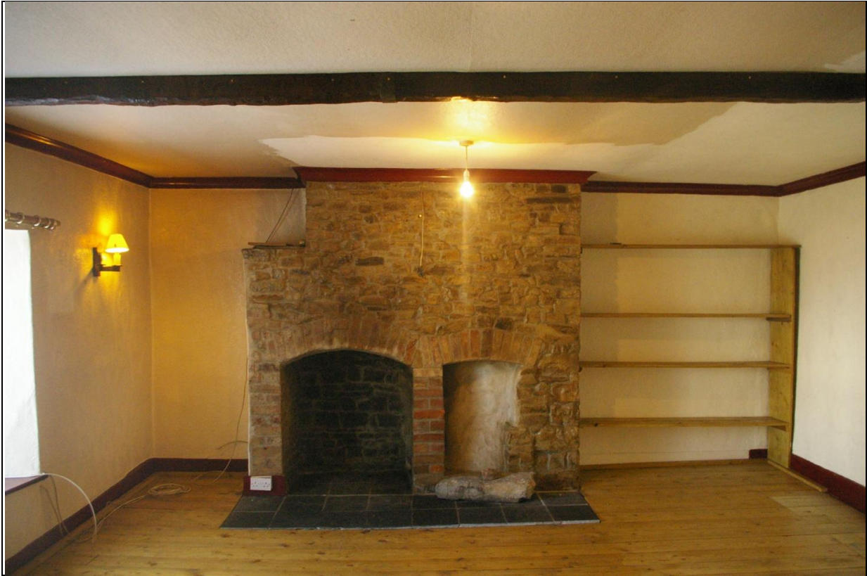
The first floor stone stack with two hearths in the 19 th century infill building; from the west.
