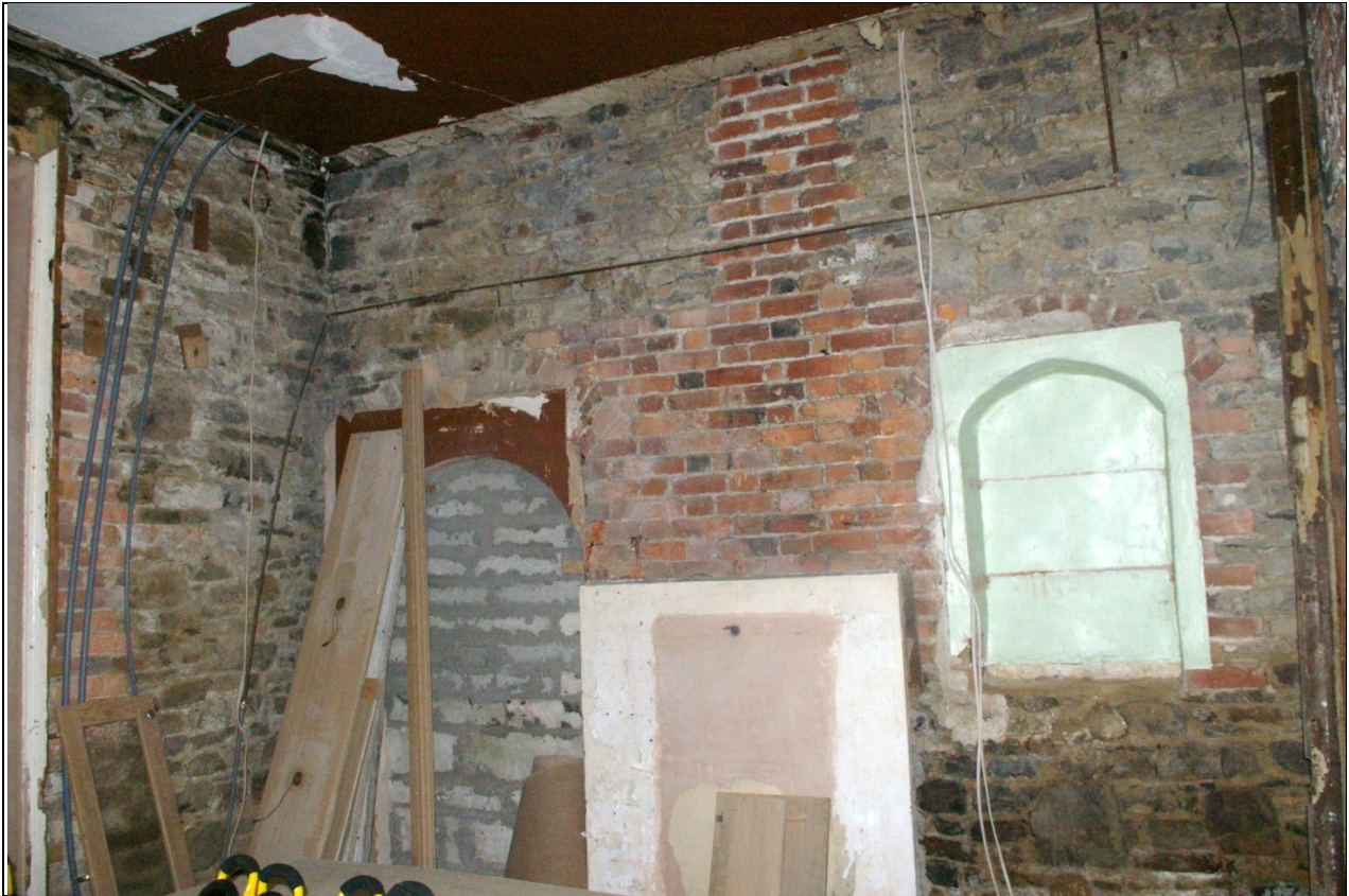
The alcove, blocked fireplace and blocked doorway in the north wall of the morning room, in the Manor House; from the east, south-east.
