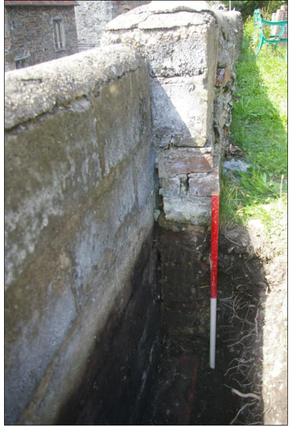
Figure 5: South-east facing section of Area #2; viewed from the south-east (scale 1m).
