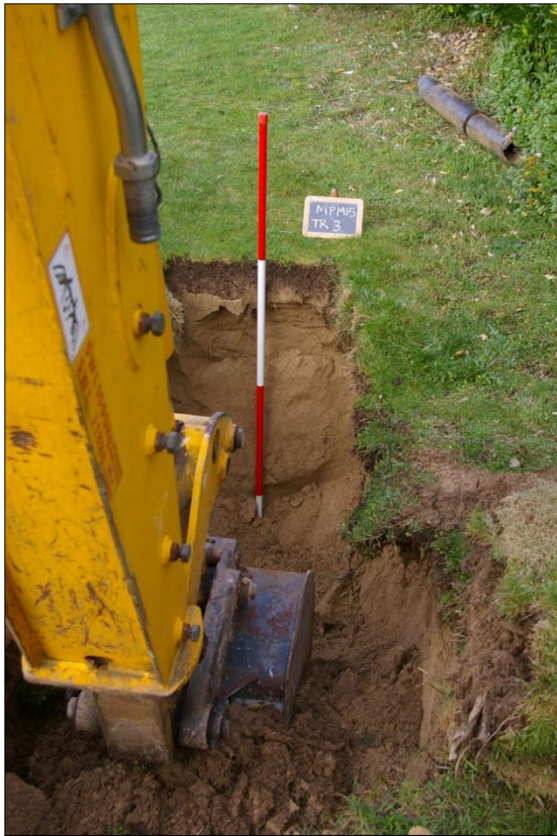
Trench #3 under excavation, the sides were too unstable to remove the digger bucket; viewed from the east (2m scale).
