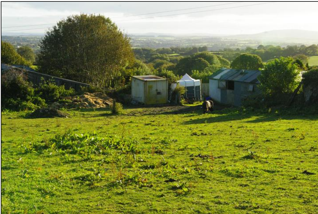
Figure 14: View towards the eastern corner of the site, looking east.
