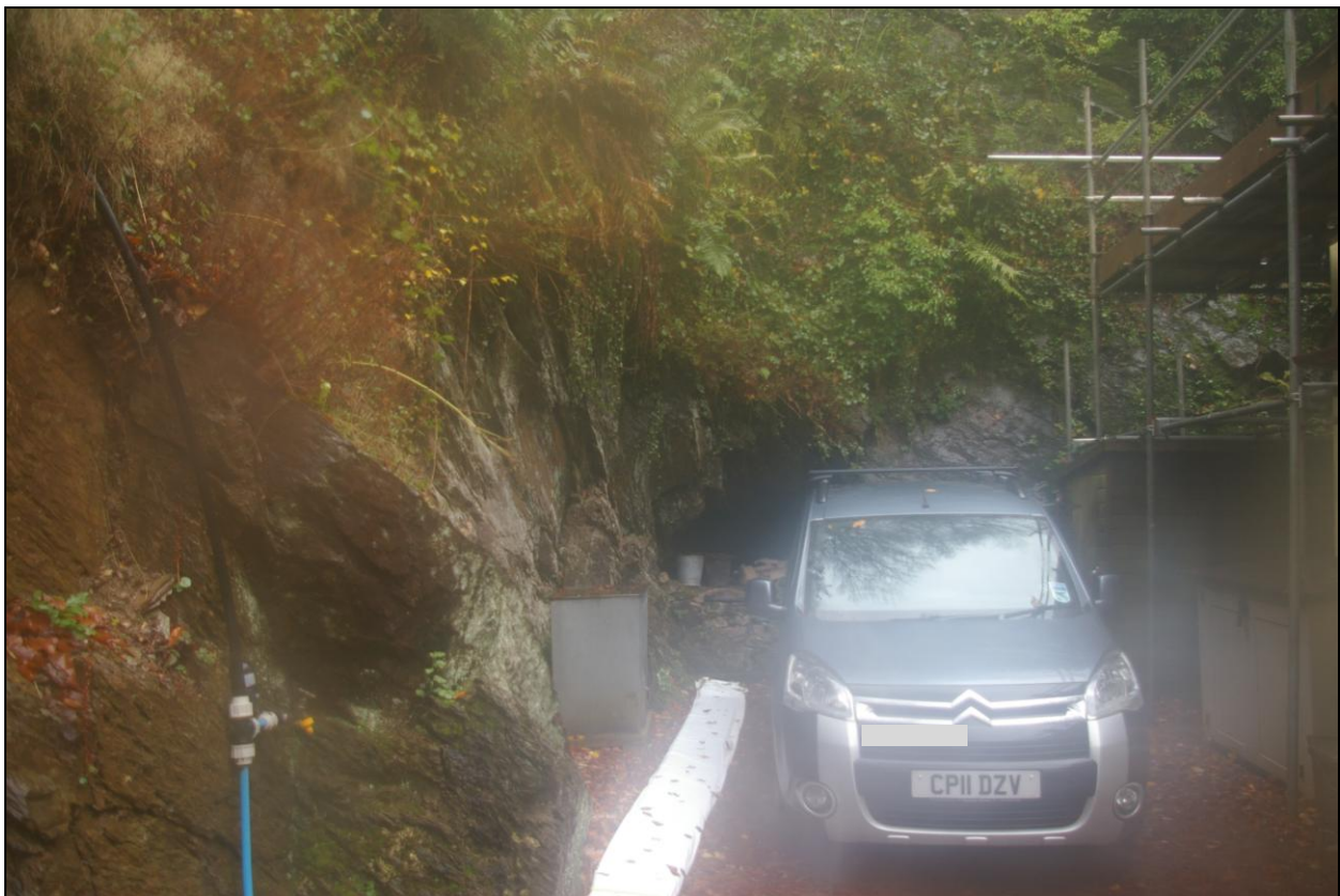
2. View along the northern site boundary, showing the quarry face and the rock-cut adit entrance in the north-east corner; from the west.
