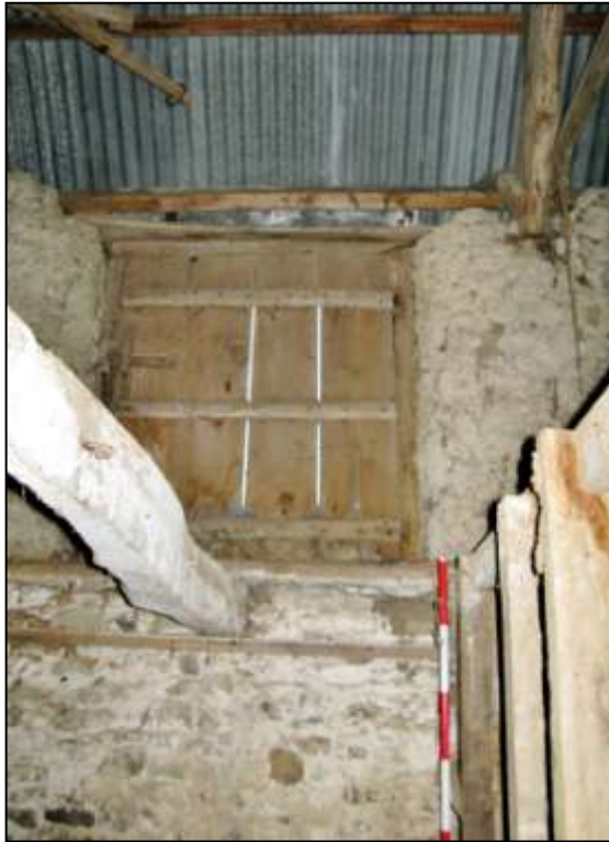
Rear of first floor loading door in east wall (2m scale).
