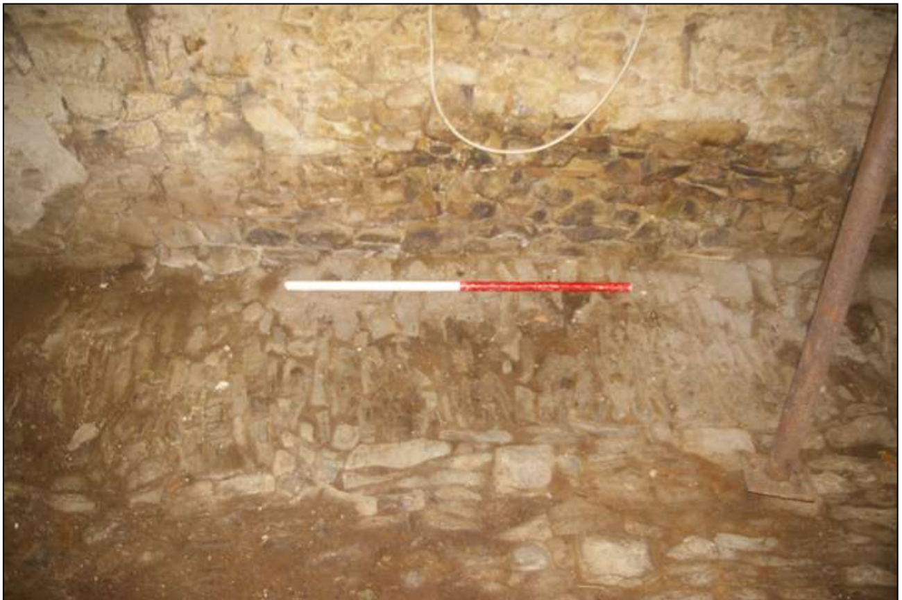
Detail of floor beneath north window; viewed from the west (1m scale).
