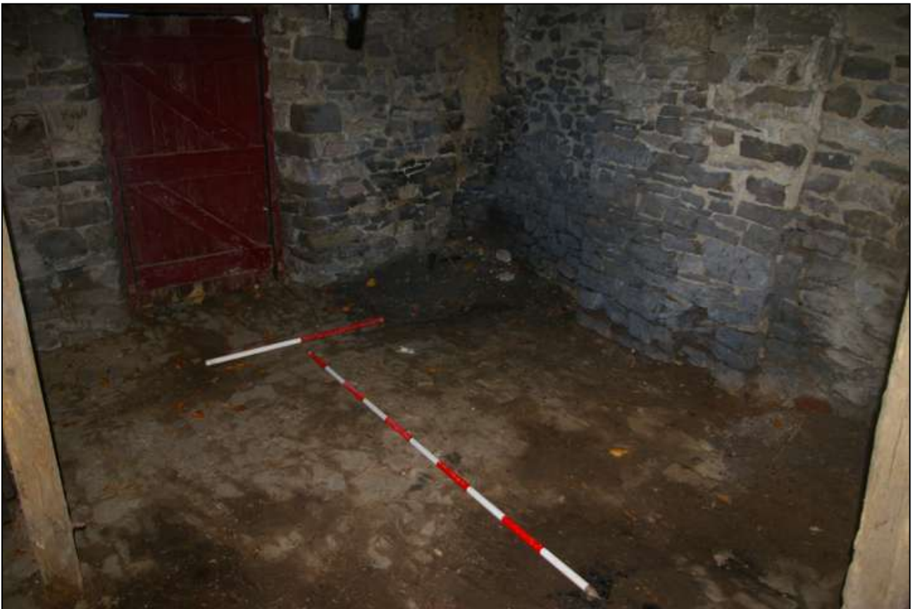
View to southeast corner; viewed from the northwest (1m and 2m scales).
