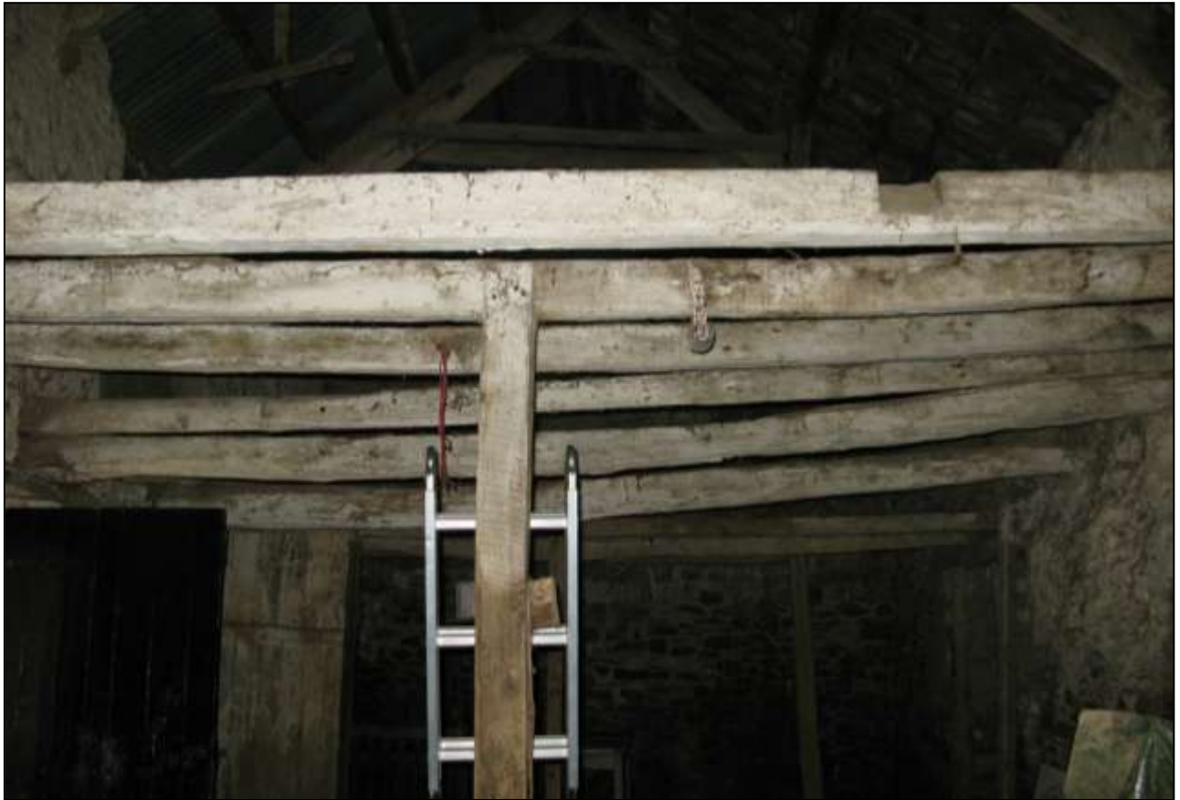
Remains of first floor joists (no scale).
