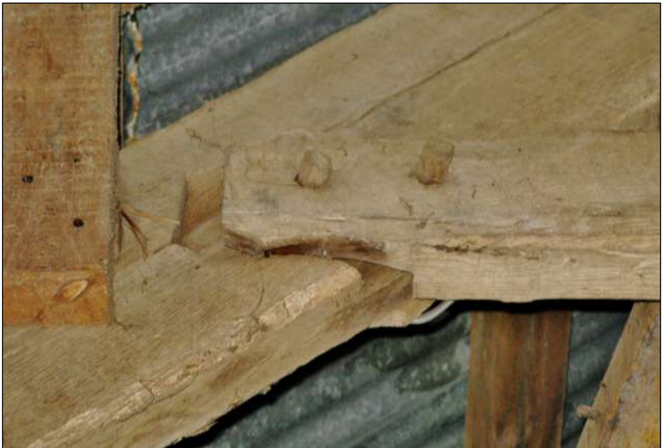
As above, detail of collar joint.
