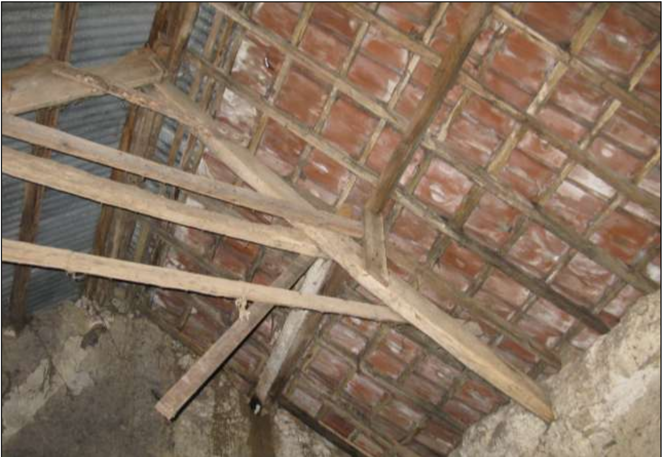
The most southerly truss showing the setting in the west wall (no scale).
