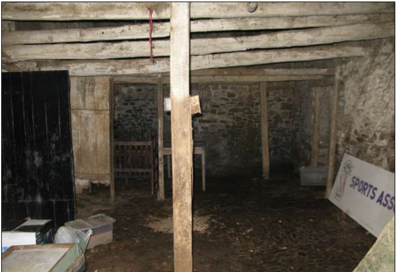
View of the south end of the barn (no scale).
