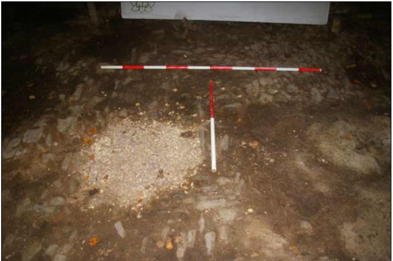
Cobble floor in centre of barn showing backfilled damaged area; viewed from the east (1m and 2m scales).
