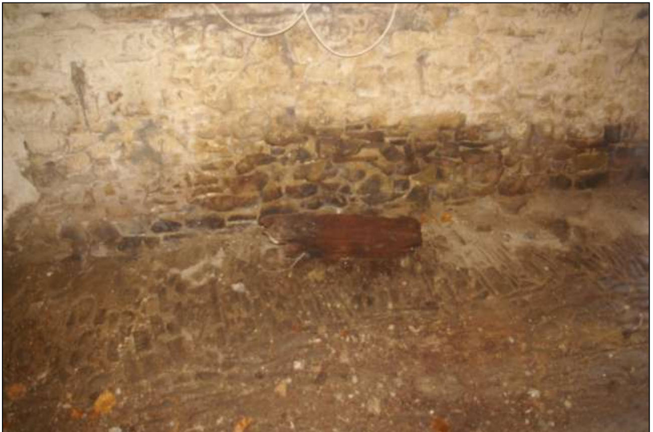
Detail of the base of the former post, removed from the floor; viewed from the west (no scale).
