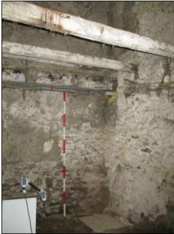
Eastern part of north wall with possible blocked opening (2m scale).
