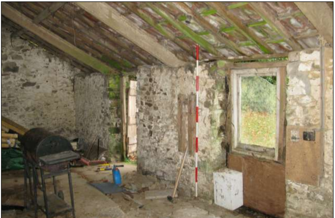
The southern end of the west wall of the lean-to.
