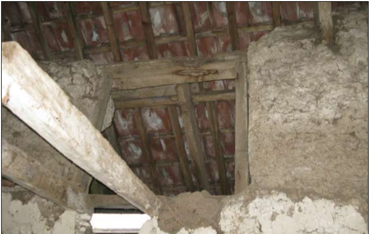
Rear of first floor loading door in west wall (no scale).
