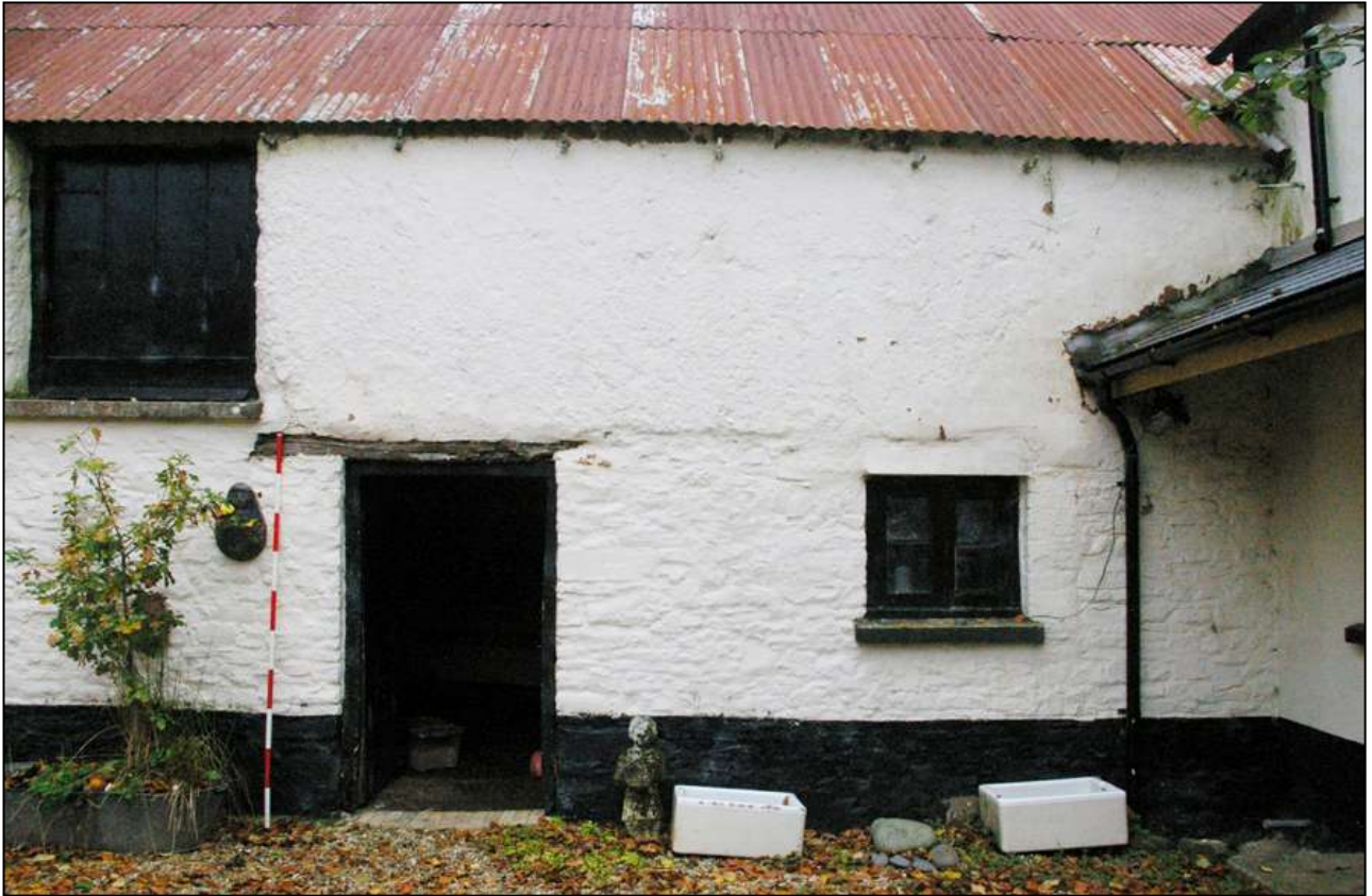
The north end of the east facing elevation (2m scale).
