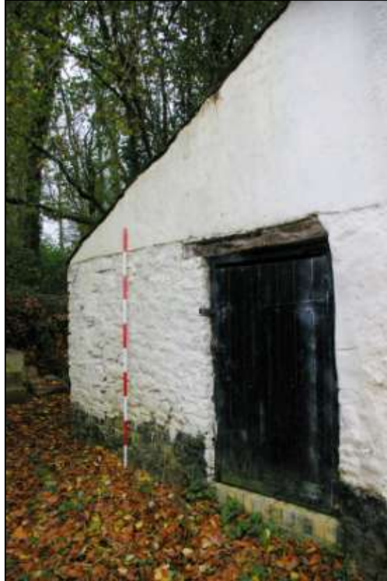
The lean-to added to the southern end of the barn (2m scale).
