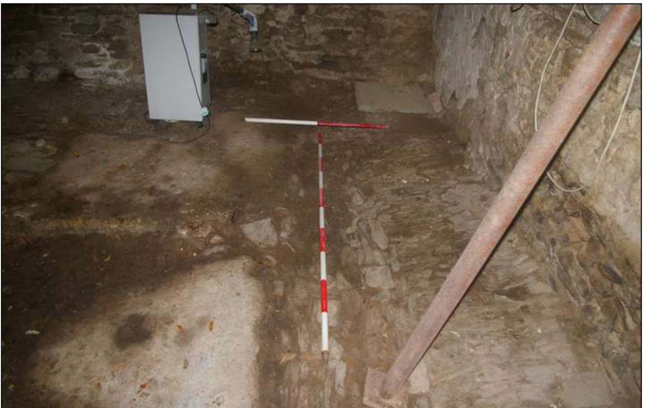
View to northeast corner from doorway; viewed from the south (1m and 2m scales).
