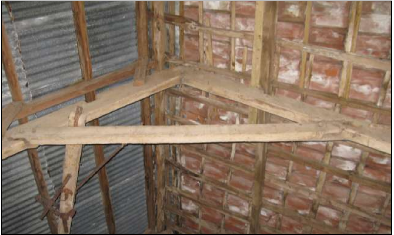
The most northerly truss viewed from the north (no scale).
