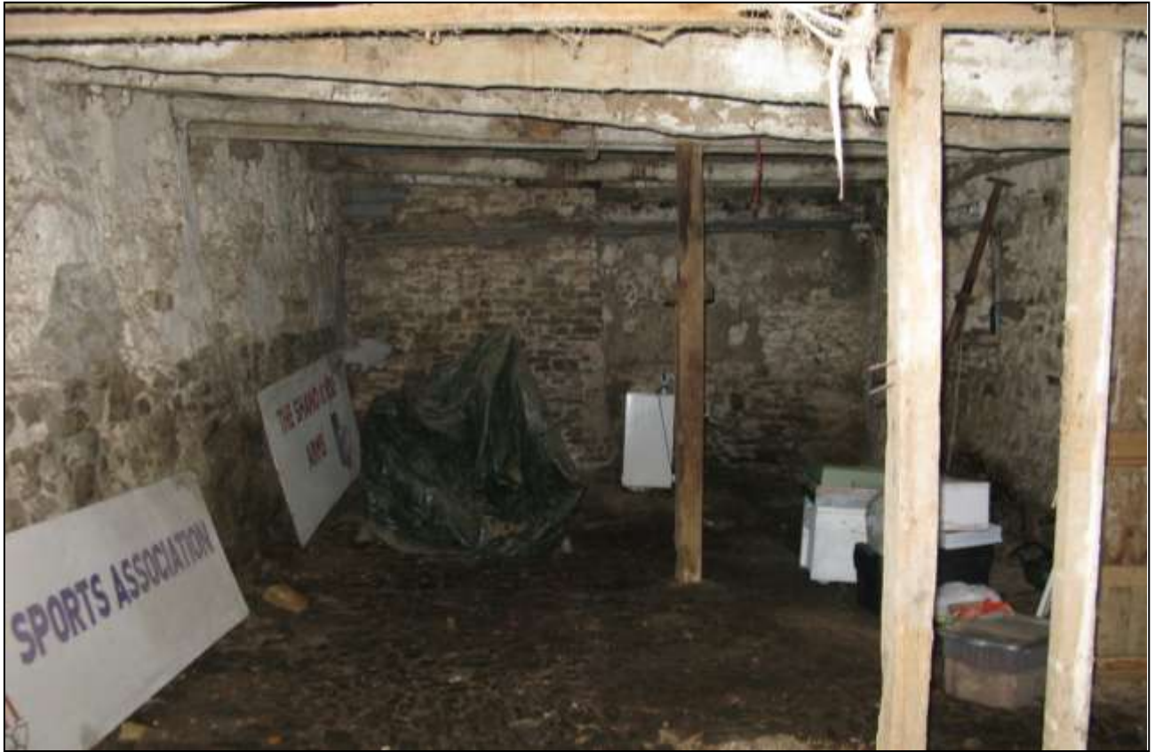
View of the north end of the barn (no scale).
