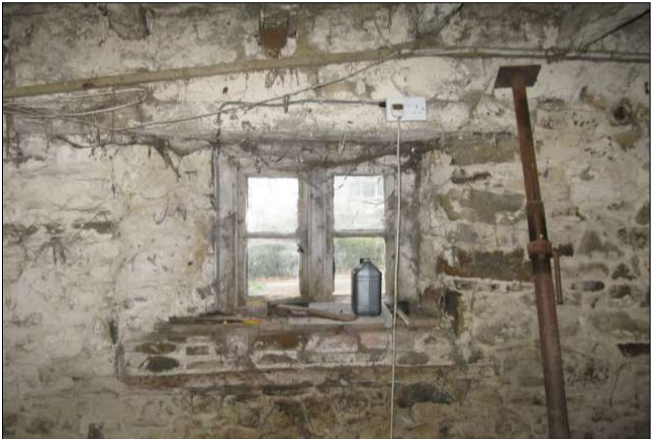
The window set in a reduced opening in the north end of the east wall (no scale).
