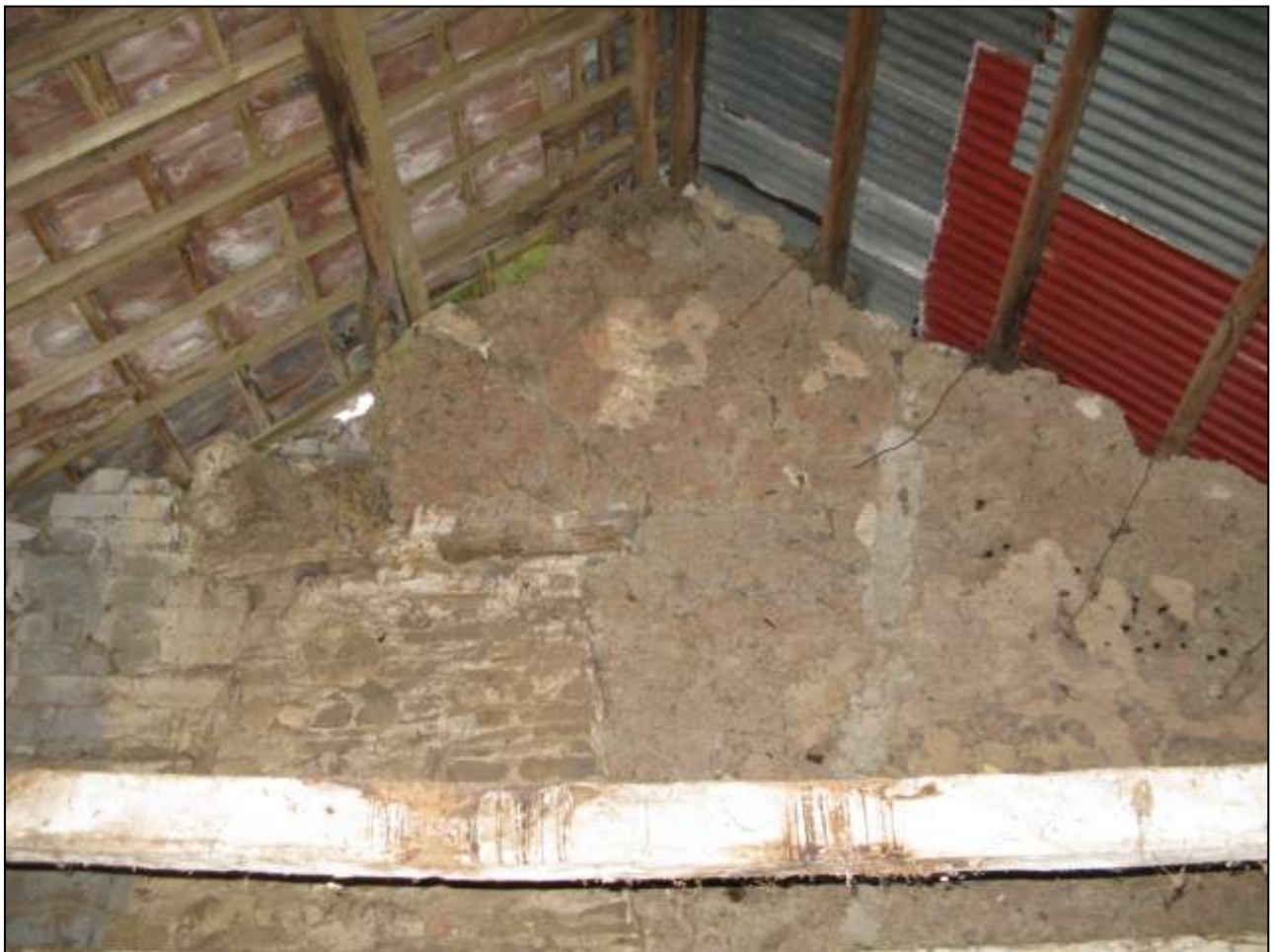
Upper gable of north wall (no scale).
