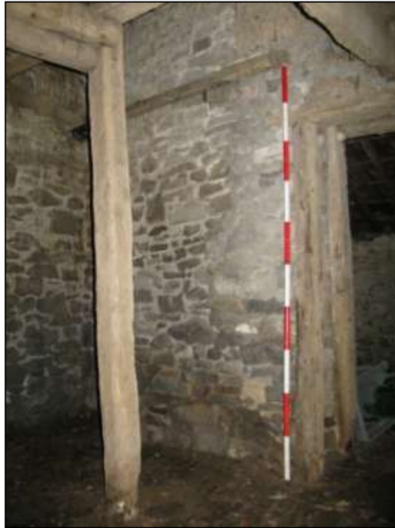
The corner of the south and west walls (2m scale).
