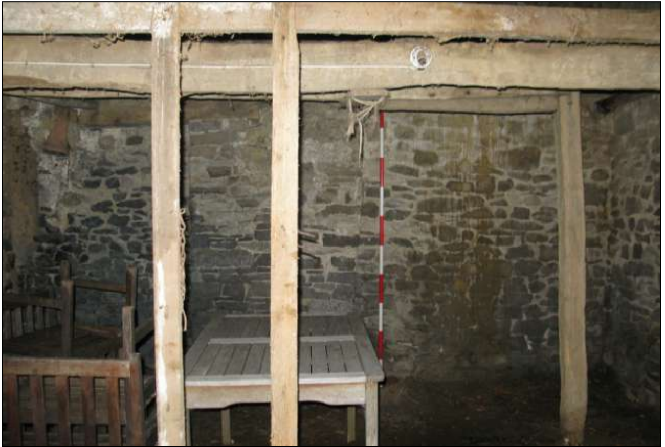
The central section of the south wall (2m scale).
