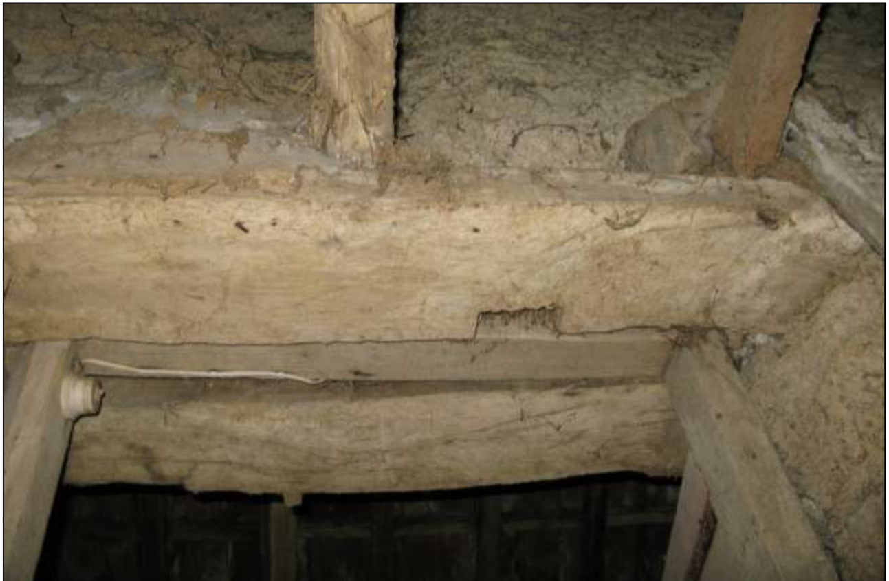
As above showing re-used timber lintel; a possible truss blade (no scale).
