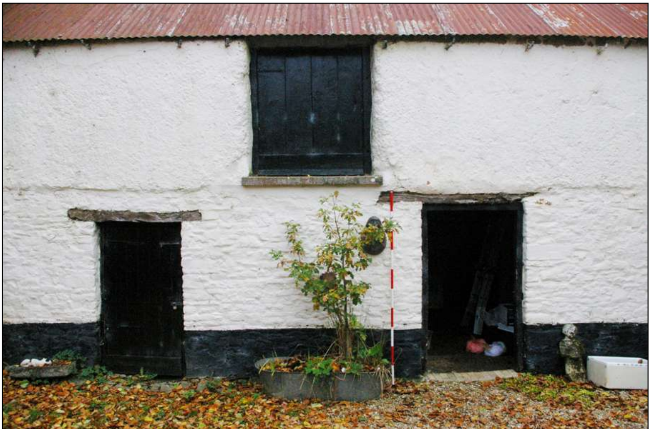
The central part of the east facing elevation (2m scale).
