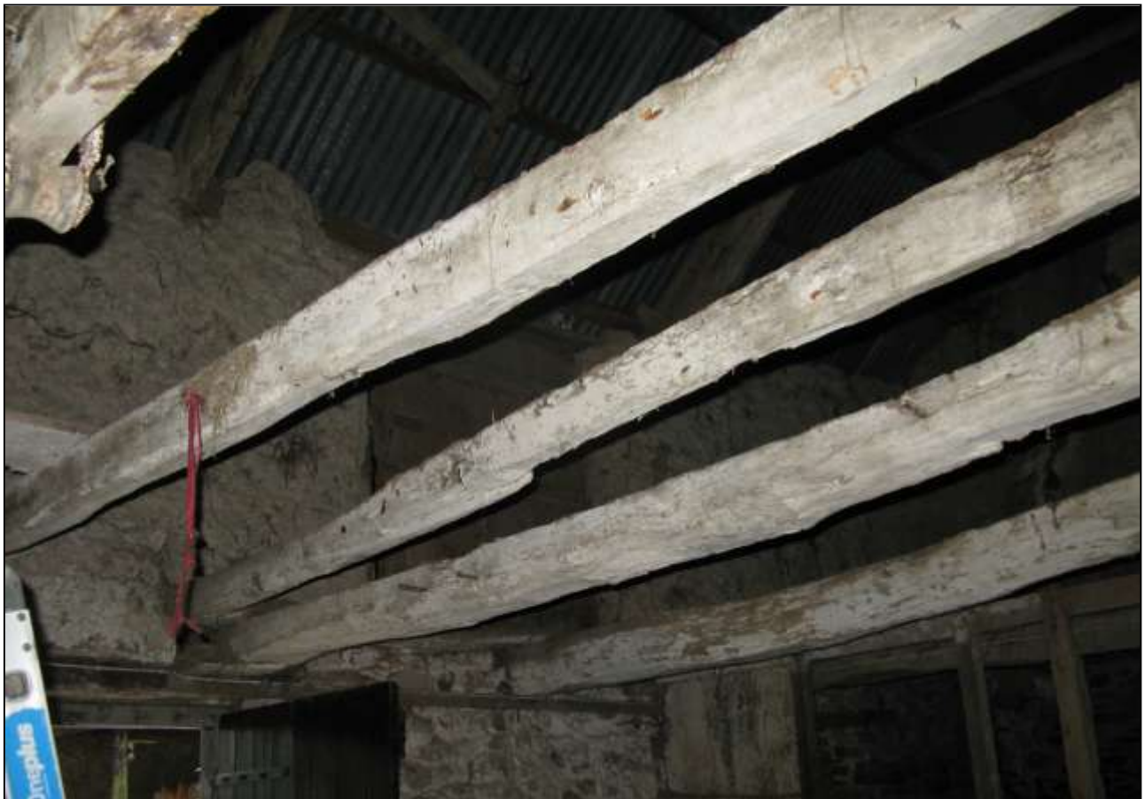
Remains of first floor joists (no scale).
