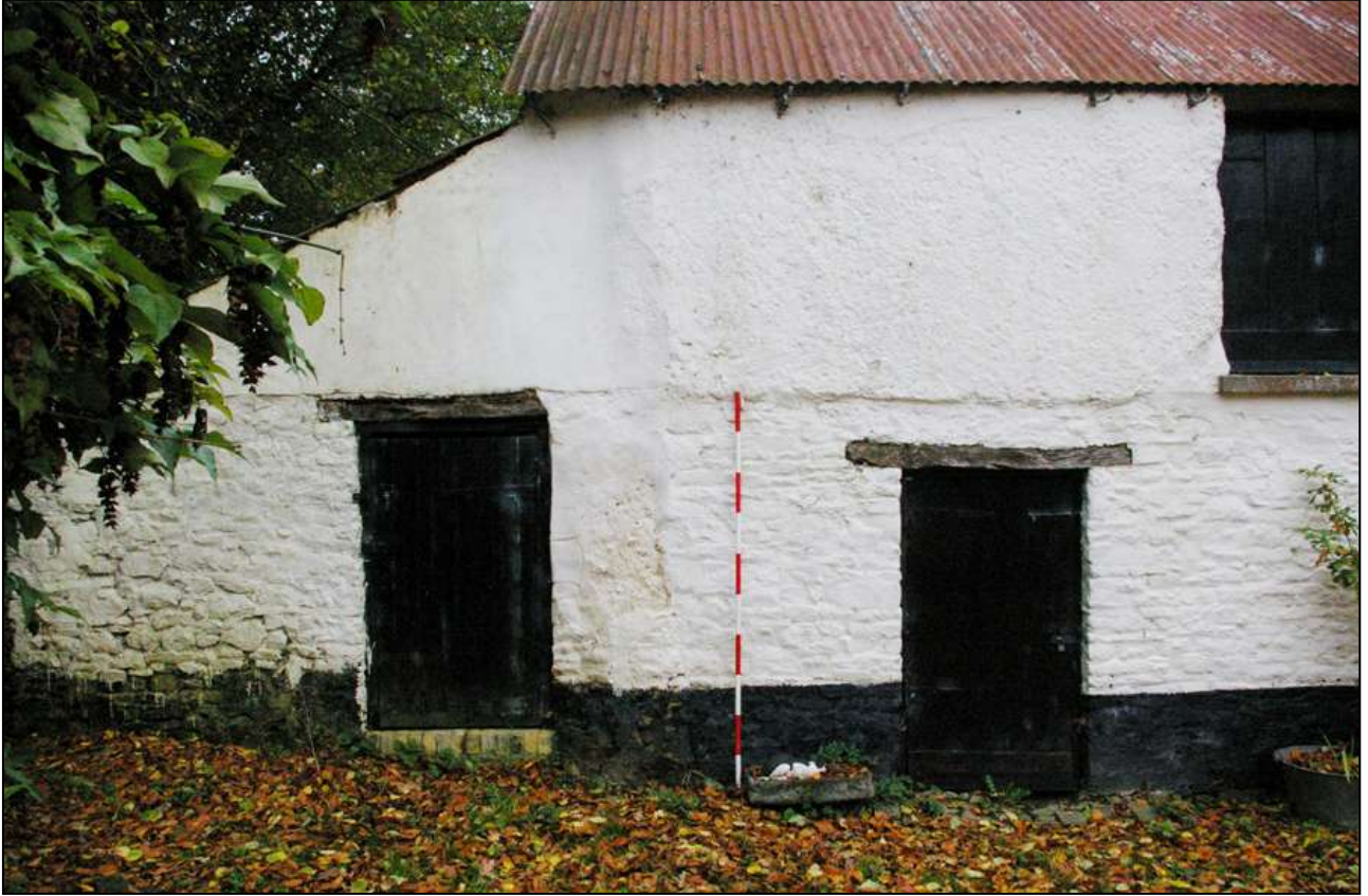
The southern part of the east facing elevation (2m scale).
