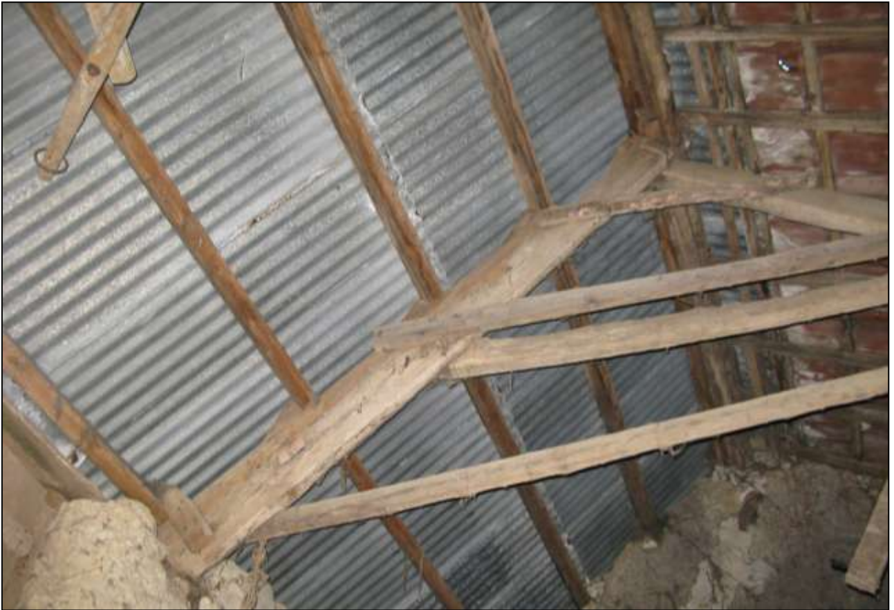
The most southerly truss showing the setting in the east wall (no scale).
