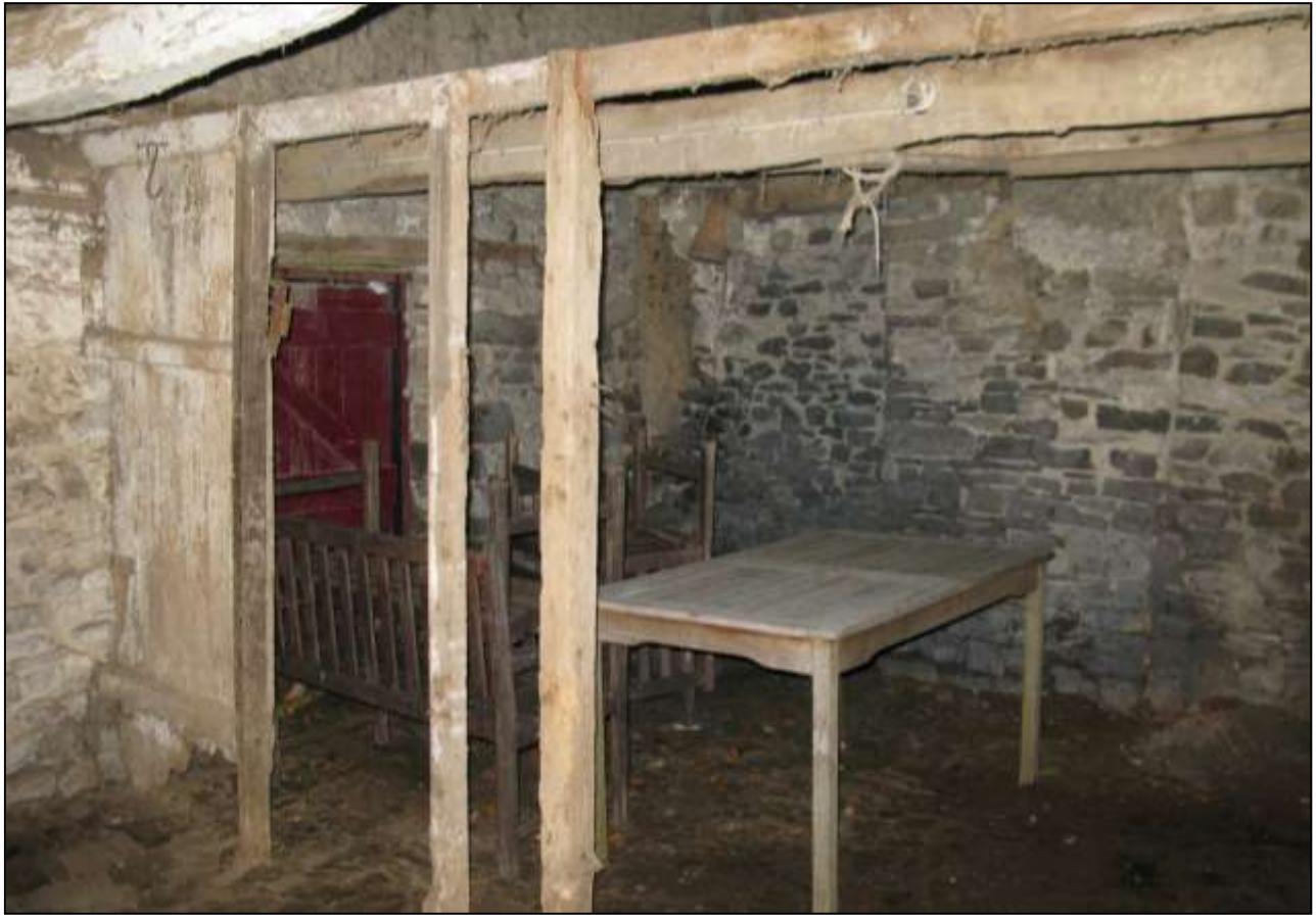
The southern end of the east wall showing the doorway and remains of the partition (no scale).
