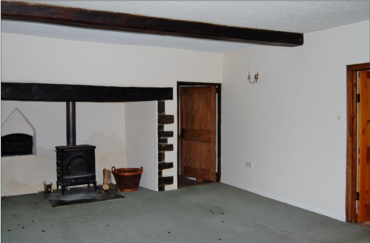
Figure 6: Room D, showing the fireplace; from the north (from the 2015 survey).
