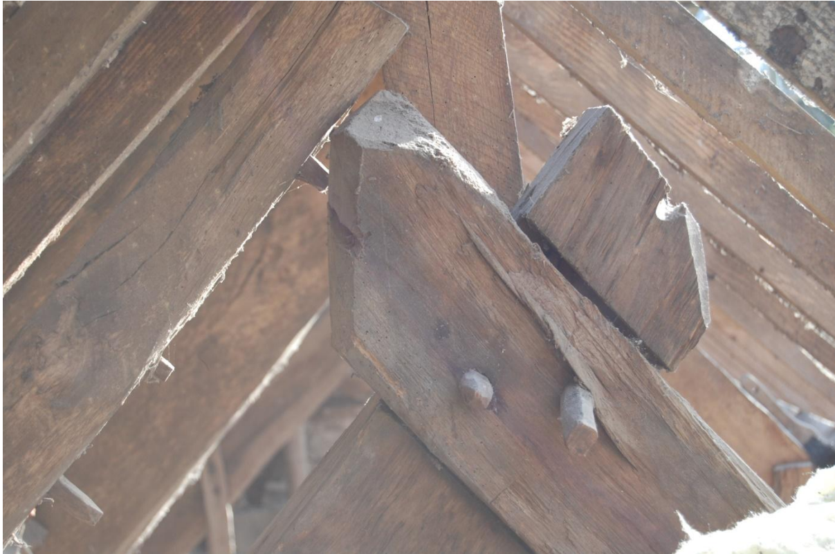
Figure 10: Internal Roof Structure showing apex of truss 3.
