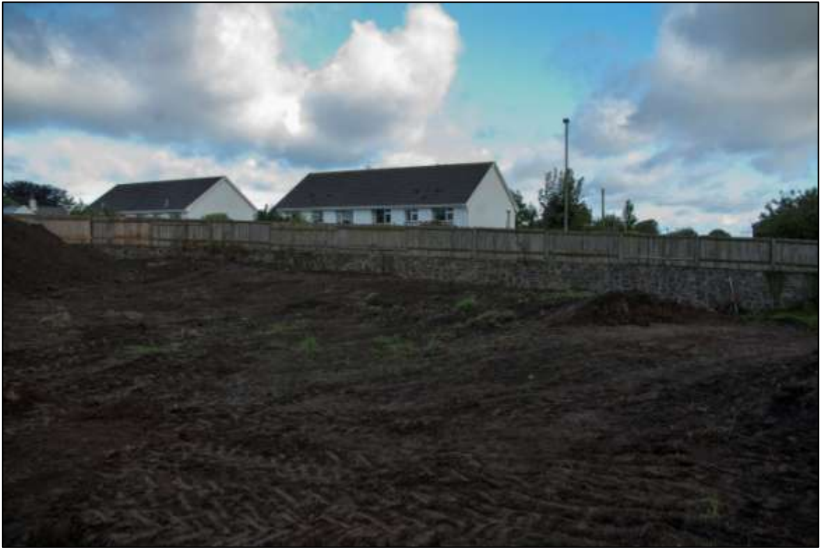
Pre-excitation view of bank <404>/<504>; looking north-west.
