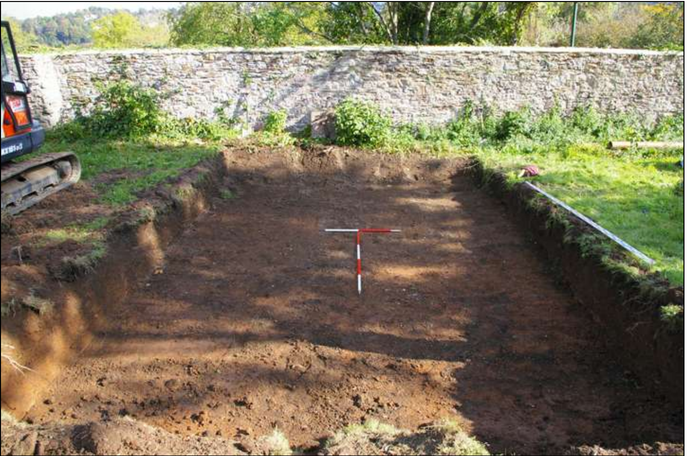
Figure 1: South end of excavation area, showing the eastern retaining wall; looking east (1m & 2m scale).
