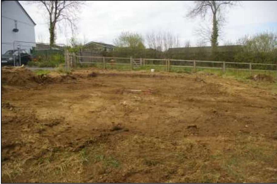
FIGURE 3: PLOTS 1 AND 2; MID EXCAVATION , PRE-FOOTINGS.
