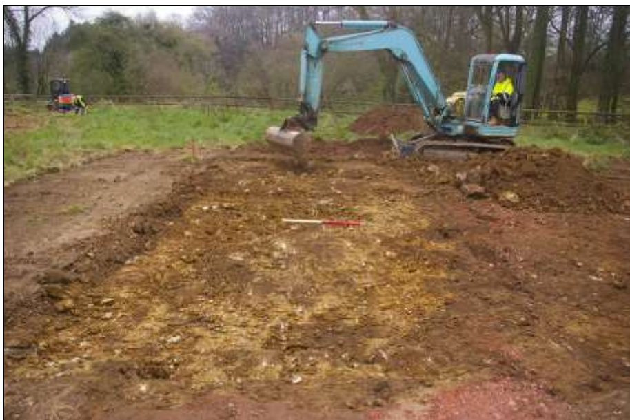
FIGURE 5: PLOT 3 AND 4; MID EXCAVATION, PRE-FOOTINGS.
