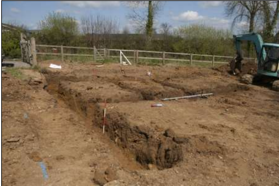
FIGURE 4: PLOT 1 AND 2 FOOTINGS; MID EXCAVATION.
