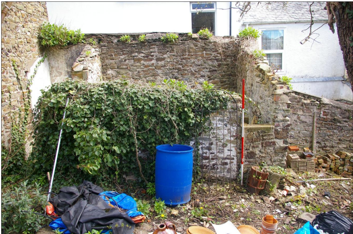
WEST ELEVATION OF THE OUTBUILDING; VIEWED FROM THE WEST (2M SCALE).
