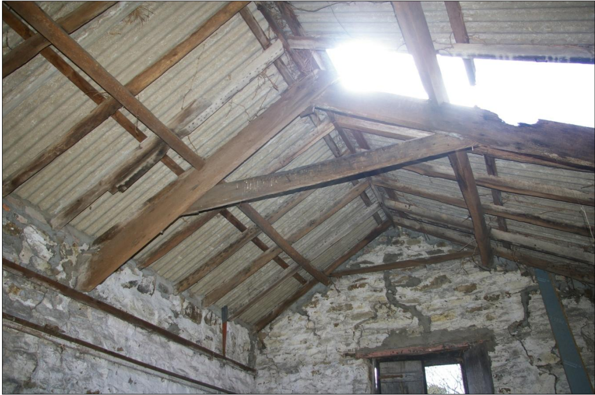
DETAIL OF THE 'A'-FRAME WITHIN THE 20 TH CENTURY ROOF STRUCTURE OF THE BARN; VIEWED FROM THE NORTH-WEST (NO SCALE).
