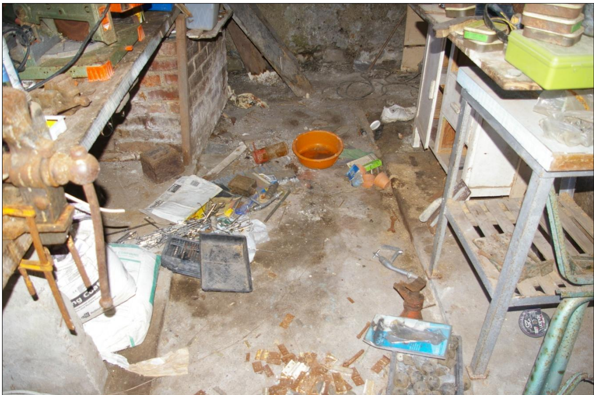
DETAIL OF THE MAIN SURVIVING CONCRETE FLOOR WITHIN THE BARN, SHOWING THE RAISED PLATFORMS AGAINST EACH SIDE WALL; VIEWED FROM THE SOUTH (NO SCALE).
