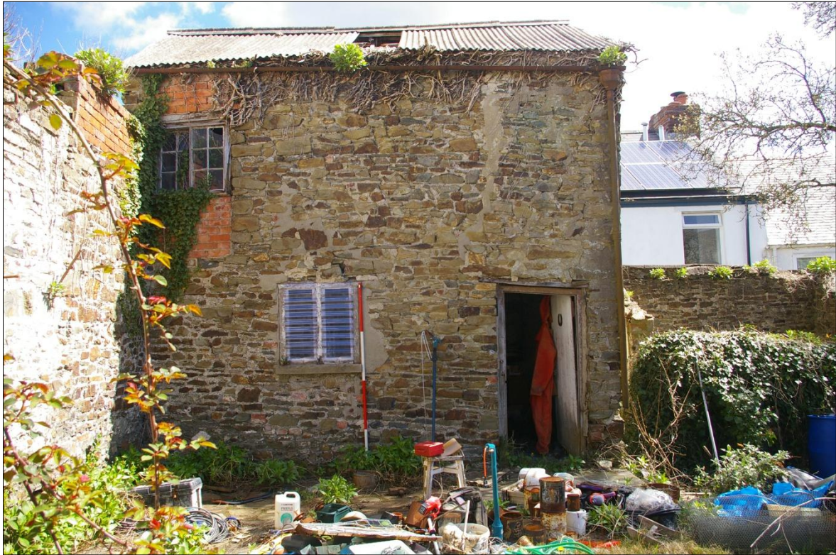
WEST ELEVATION OF THE BARN; VIEWED FROM THE WEST (2M SCALE).
