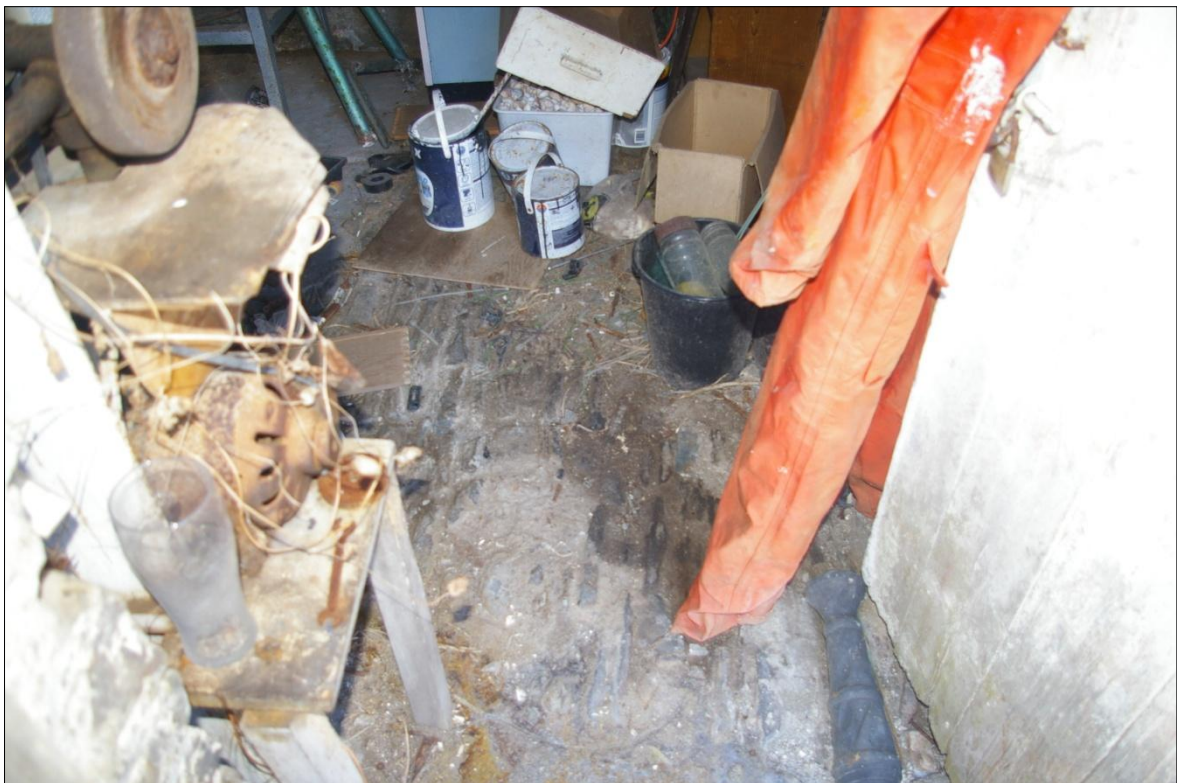
DETAIL OF THE SURVIVING COBBLE FLOOR IN THE EXISTING DOORWAY TO THE BARN; VIEWED FROM THE WEST (NO SCALE).
