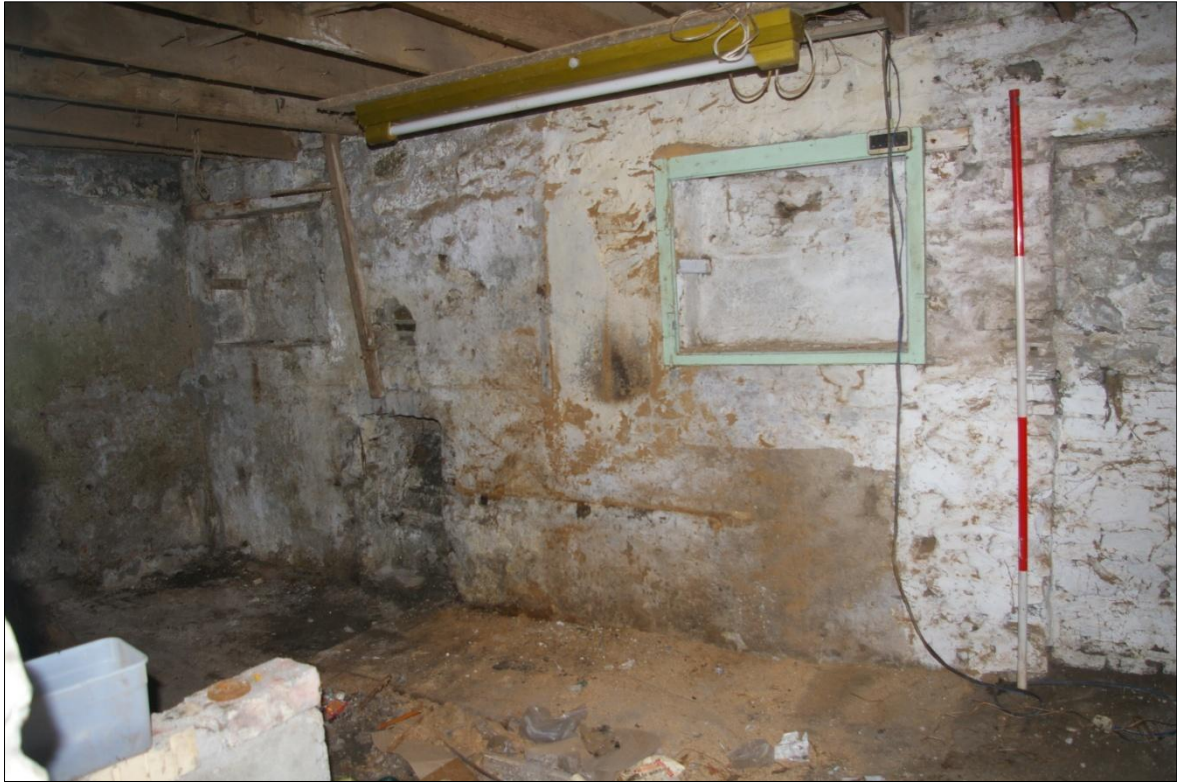
INTERIOR OF THE BARN, SHOWING THE INTERNAL FACE OF THE EAST BURGAGE PLOT WALL WITH DETAILS OF THE BLOCKED DOOR, WINDOWS AND FIREPLACE; VIEWED FROM THE WEST (2M SCALE).
