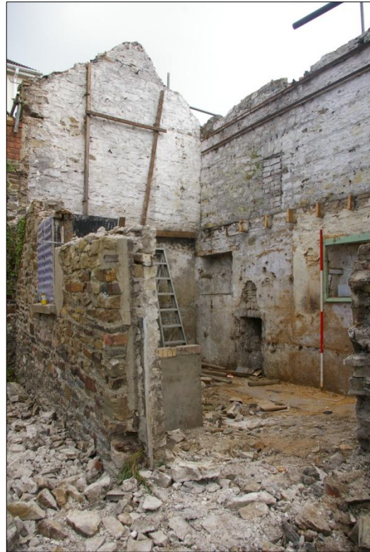
(LEFT) THE INTERNAL FACE OF THE EAST WALL OF THE BARN, FOLLOWING REMOVAL OF THE ROOF, INTERNAL FITTINGS AND PARTIAL DEMOLITION OF THE SOUTH AND WEST WALLS; VIEWED FROM THE SOUTH-WEST (2M SCALE).
