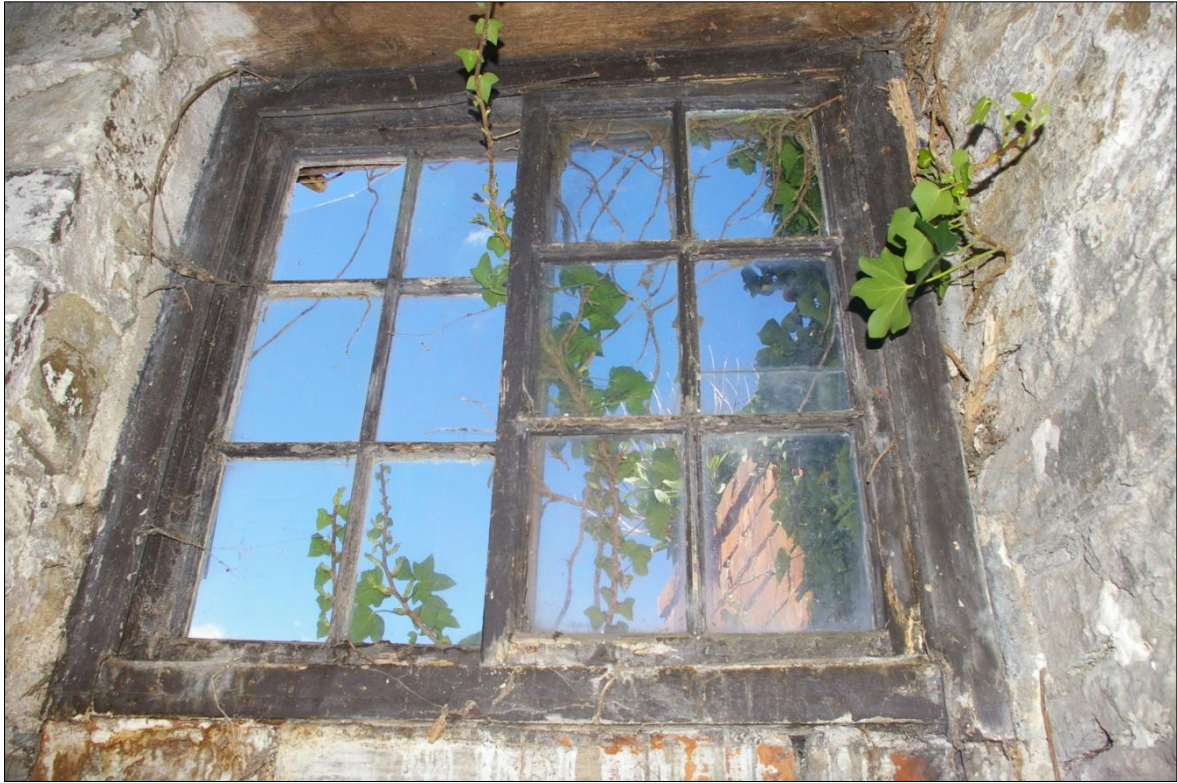
INTERNAL DETAIL OF THE SLIDING SASH WINDOW WITHIN THE BLOCKED LOADING DOOR IN THE WEST WALL OF THE BARN; VIEWED FROM THE EAST (NO SCALE).
