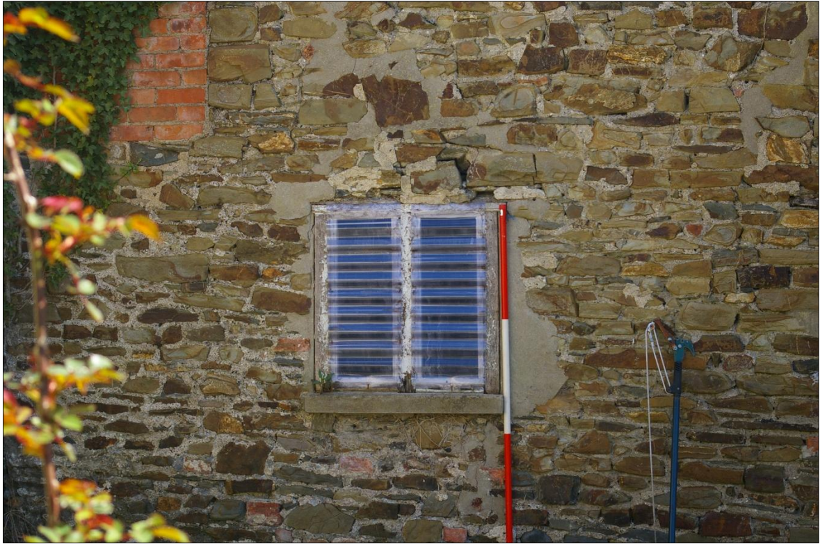
DETAIL OF THE WEST ELEVATION OF THE BARN, SHOWING THE GROUND FLOOR TIMBER WINDOW; VIEWED FROM THE WEST (2M SCALE).
