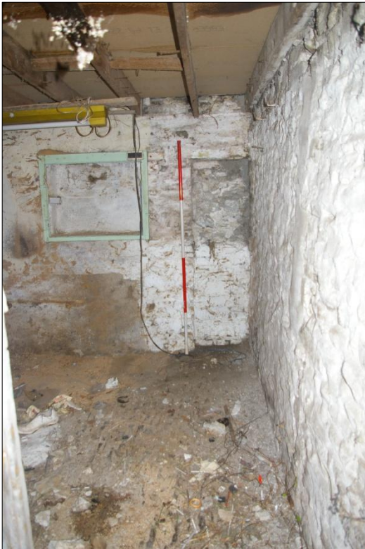
(LEFT) DETAIL OF THE INTERNAL FACE OF THE EAST WALL OF THE BARN, SHOWING THE BLOCKED DOORWAY AND COBBLED SURFACE AT THE SOUTH END; VIEWED FROM THE WEST (2M SCALE).
