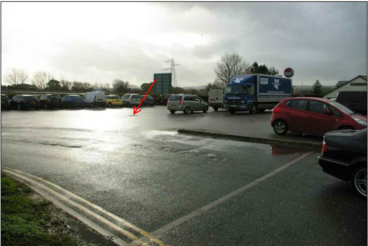
Area (C). Note the manhole cover in the centre of the car park (indicated) and the A30 embankment; viewed from the north-east.
