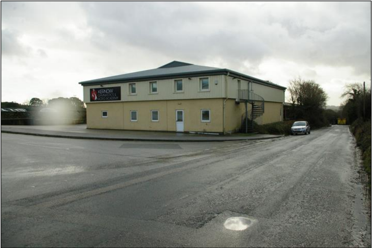
Building (E) from the north.
