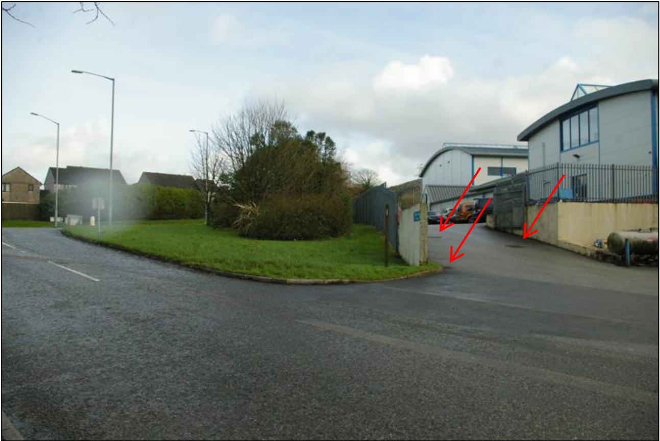
The northern side of the Kingsley Village building (manhole covers indicated); viewed from the west.
