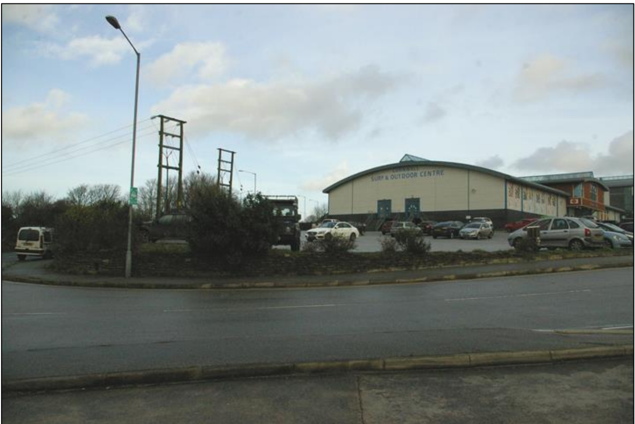
Kingsley Village and Area (B), viewed from the south-west.
