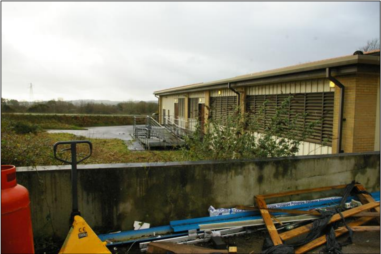
The south-east side of the building south of Building (E); viewed from the north-east.
