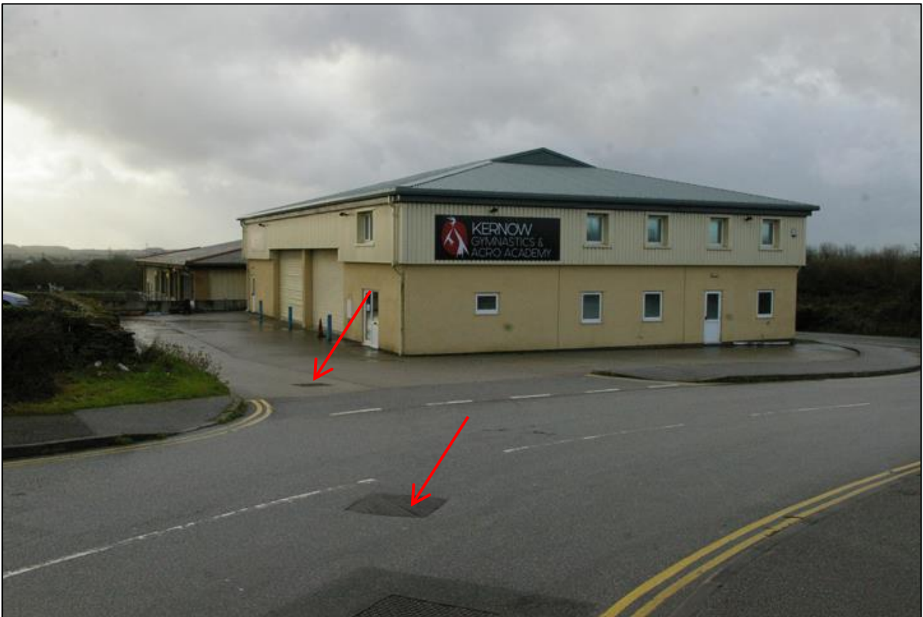
Building (E) from the east (manhole covers indicated).
