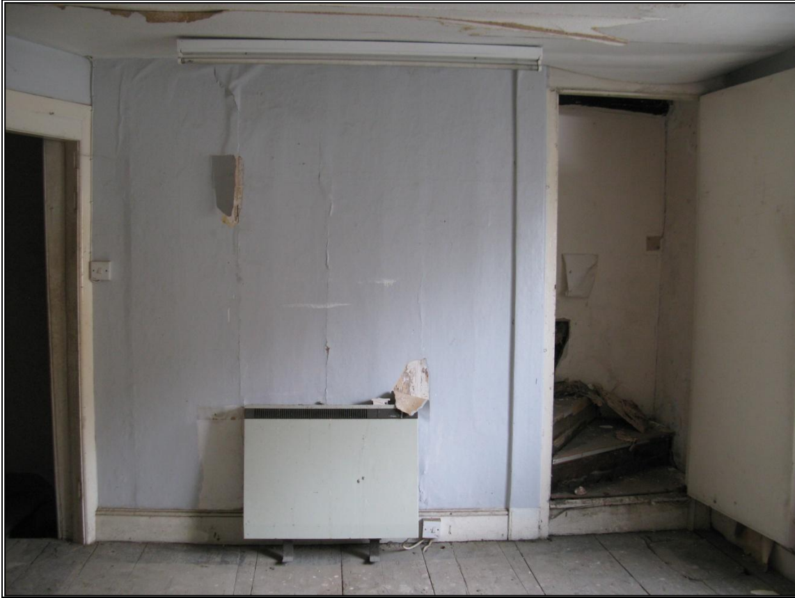
Figure 16: Attic stair in Room 10.
