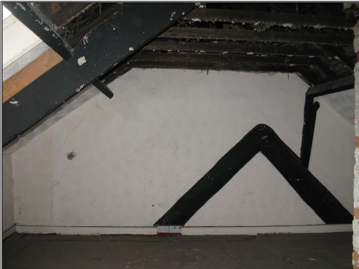
Figure 17: Early roof truss set in wall between 121 and 122 Boutport Street.
