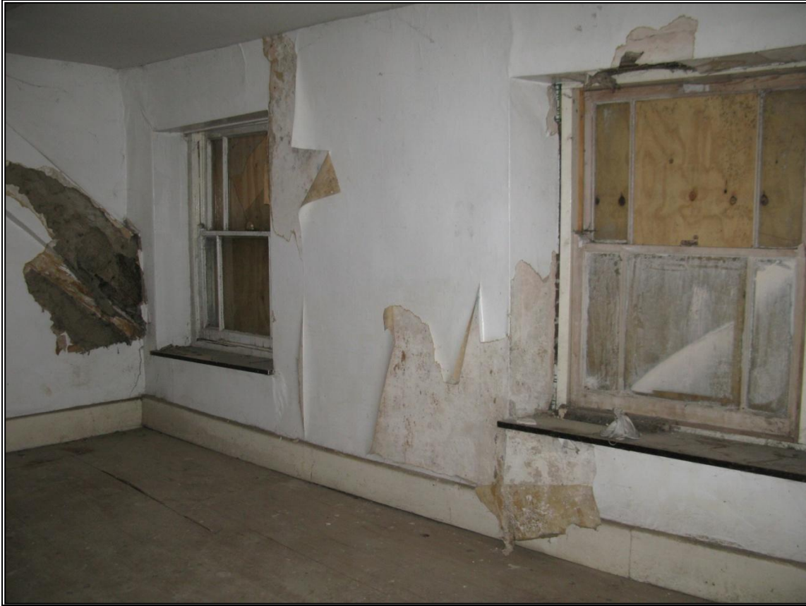
Figure 14: First floor sash windows and foot of early roof truss in the west wall.
