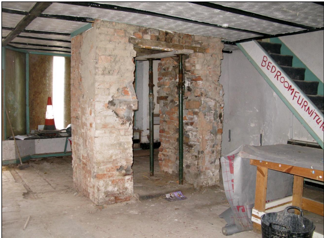
Figure 9: Rooms 1 & 2 showing partially dismantled stack.
