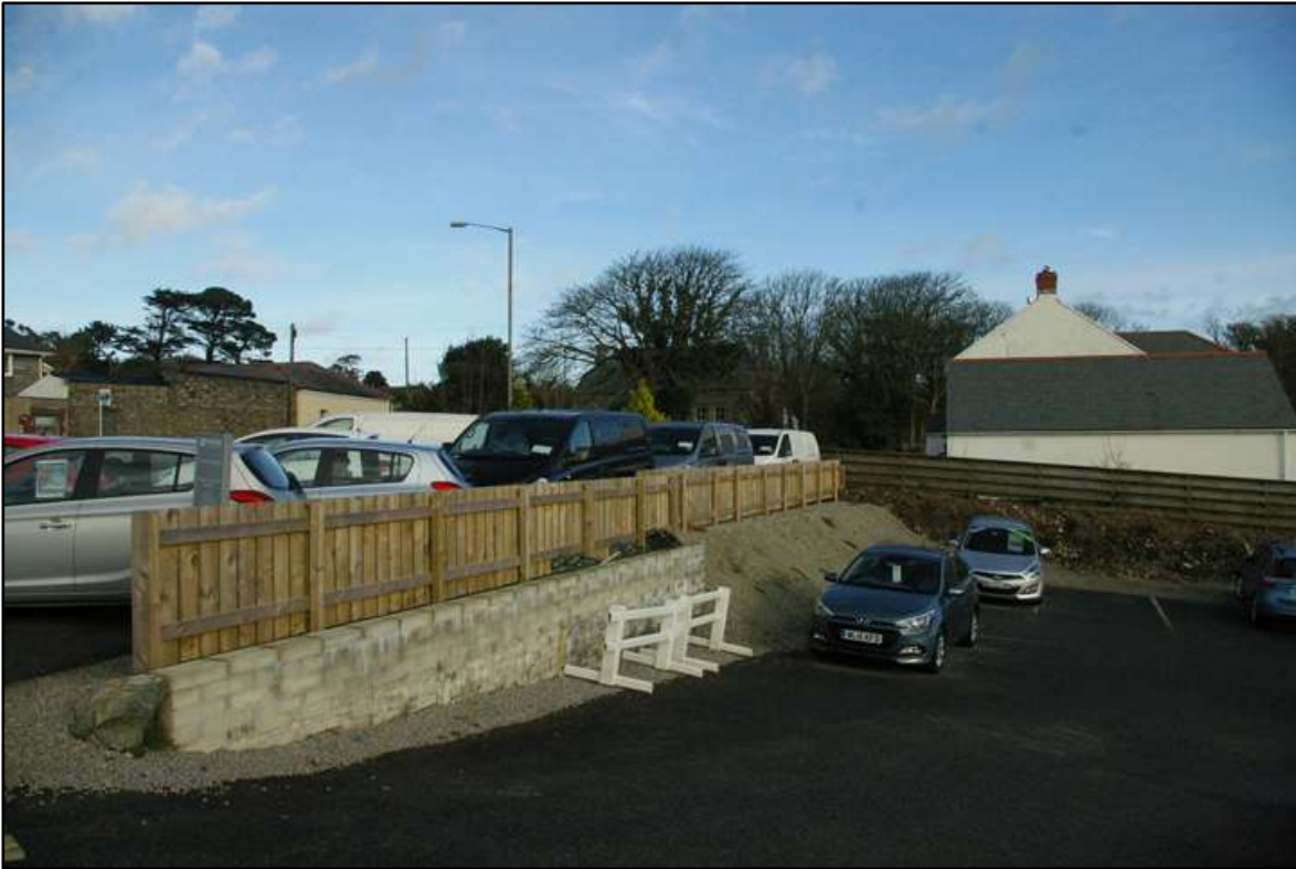
North-east part of car park looking towards Blackwater Literary Institute; Looking north-east (no scale).
