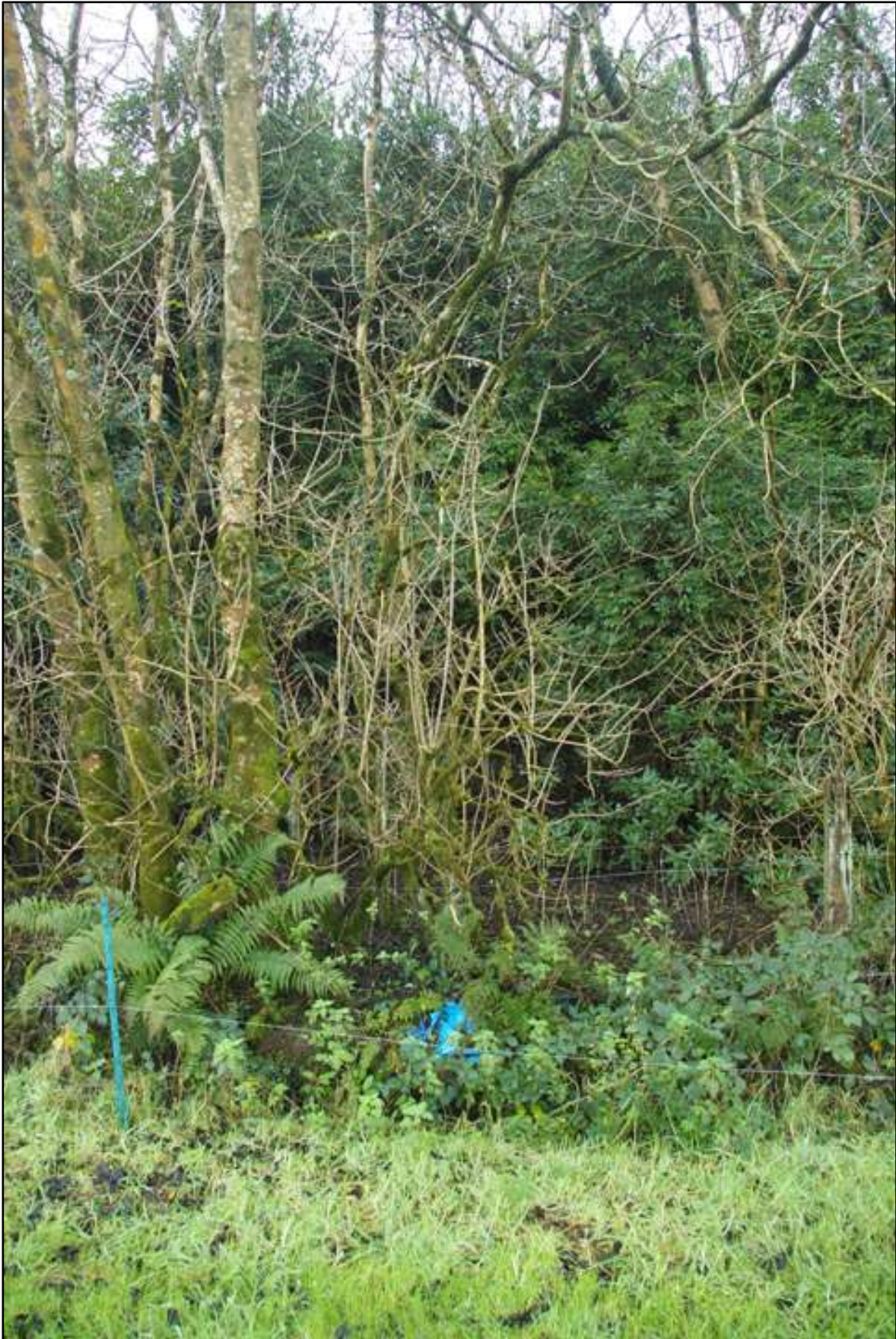
Verge of old railway embankment to south-west of the site; looking south-west (no scale).
