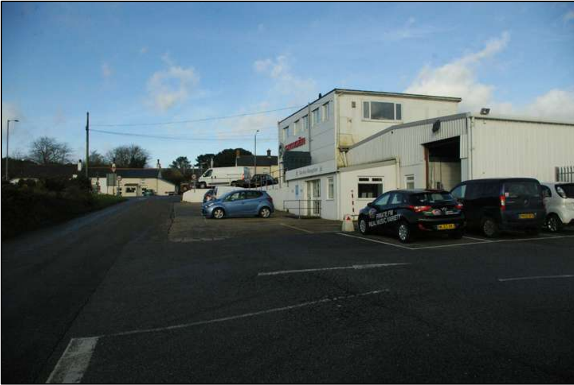
From rear car park entrance/south corner of existing building; looking north-west (no scale).
