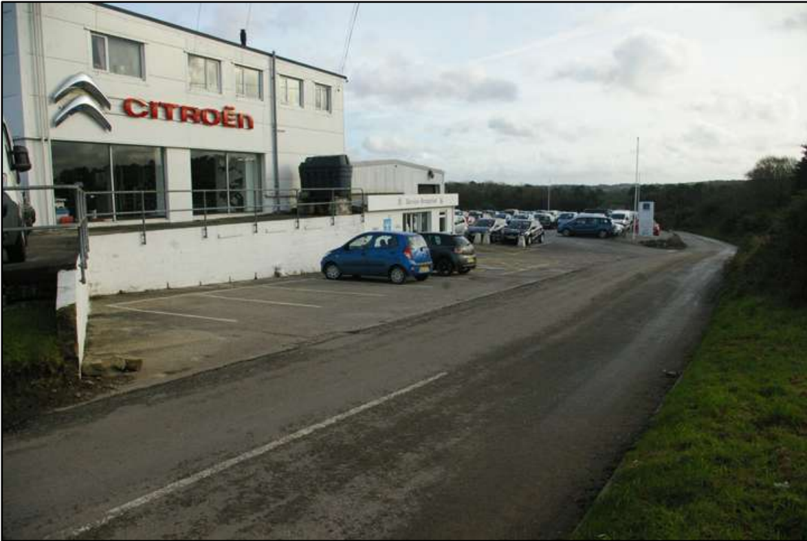
South-west side of the existing building; looking south-east (no scale).
