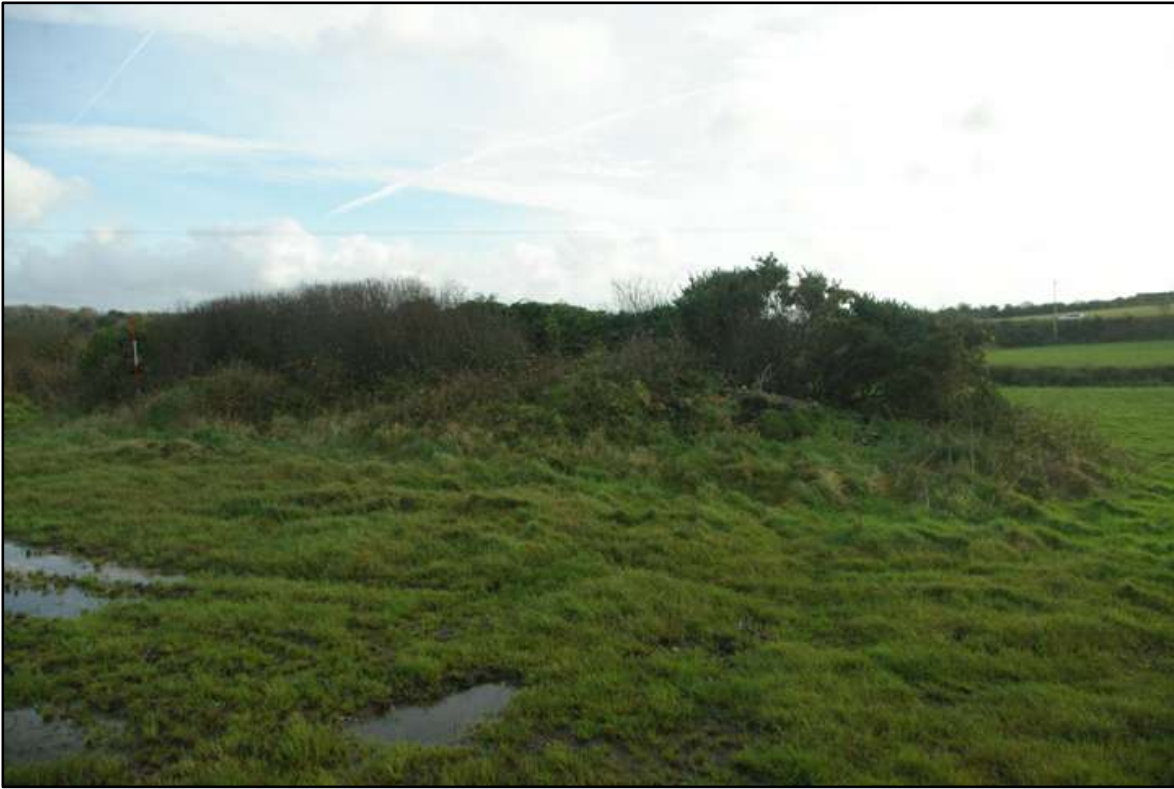
Ruin adjacent to tips c.5m×13m (0.5+m thick wall); looking south-east (2m scale).
