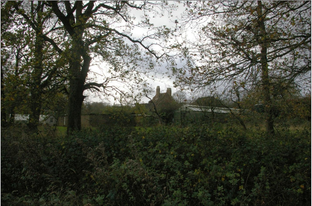
View to Crouchlands (farm)house across the 20 th century walled garden; viewed from the east.
