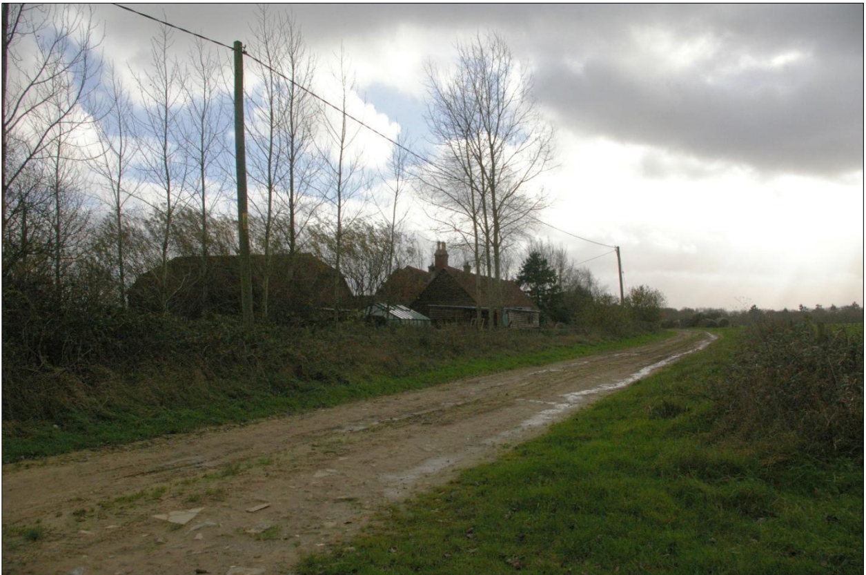
View to Lanelands, showing the screening provided to the west and north by its timber-boarded barns; viewed from the north-west.
