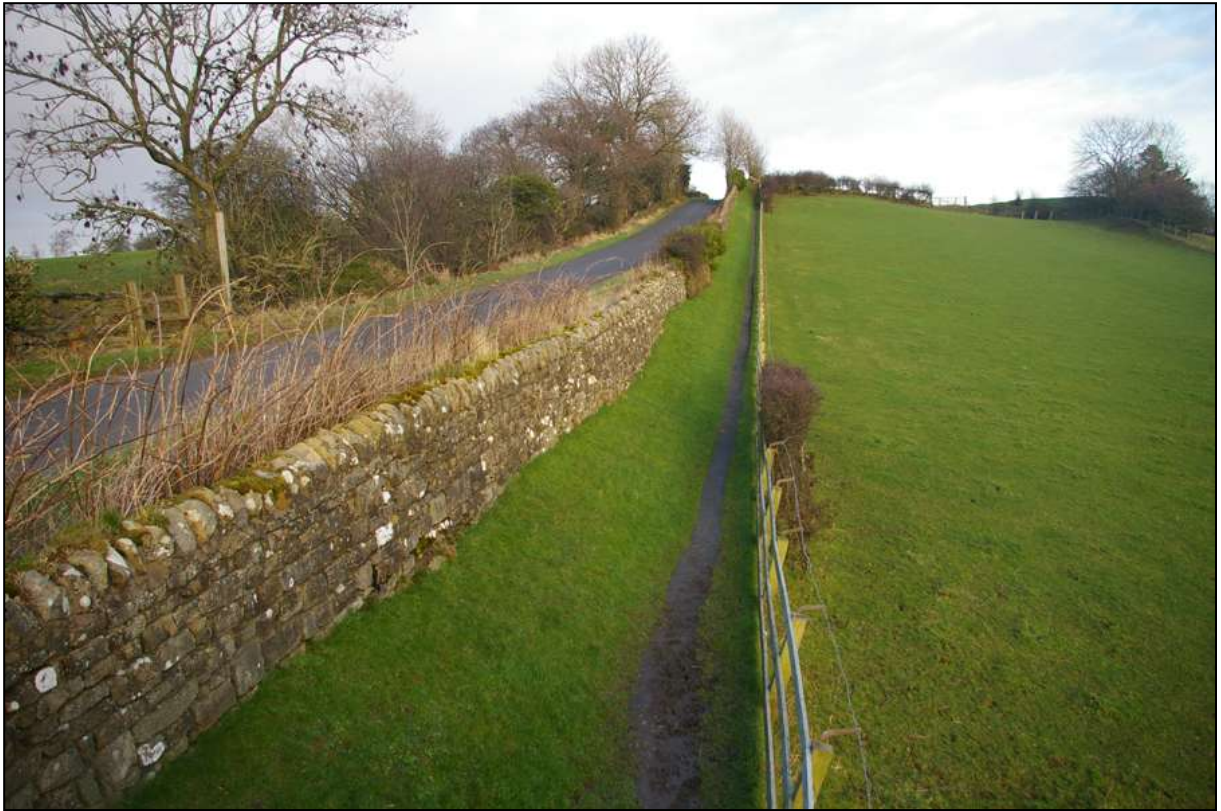
View of the wall at Banks; from the east.
