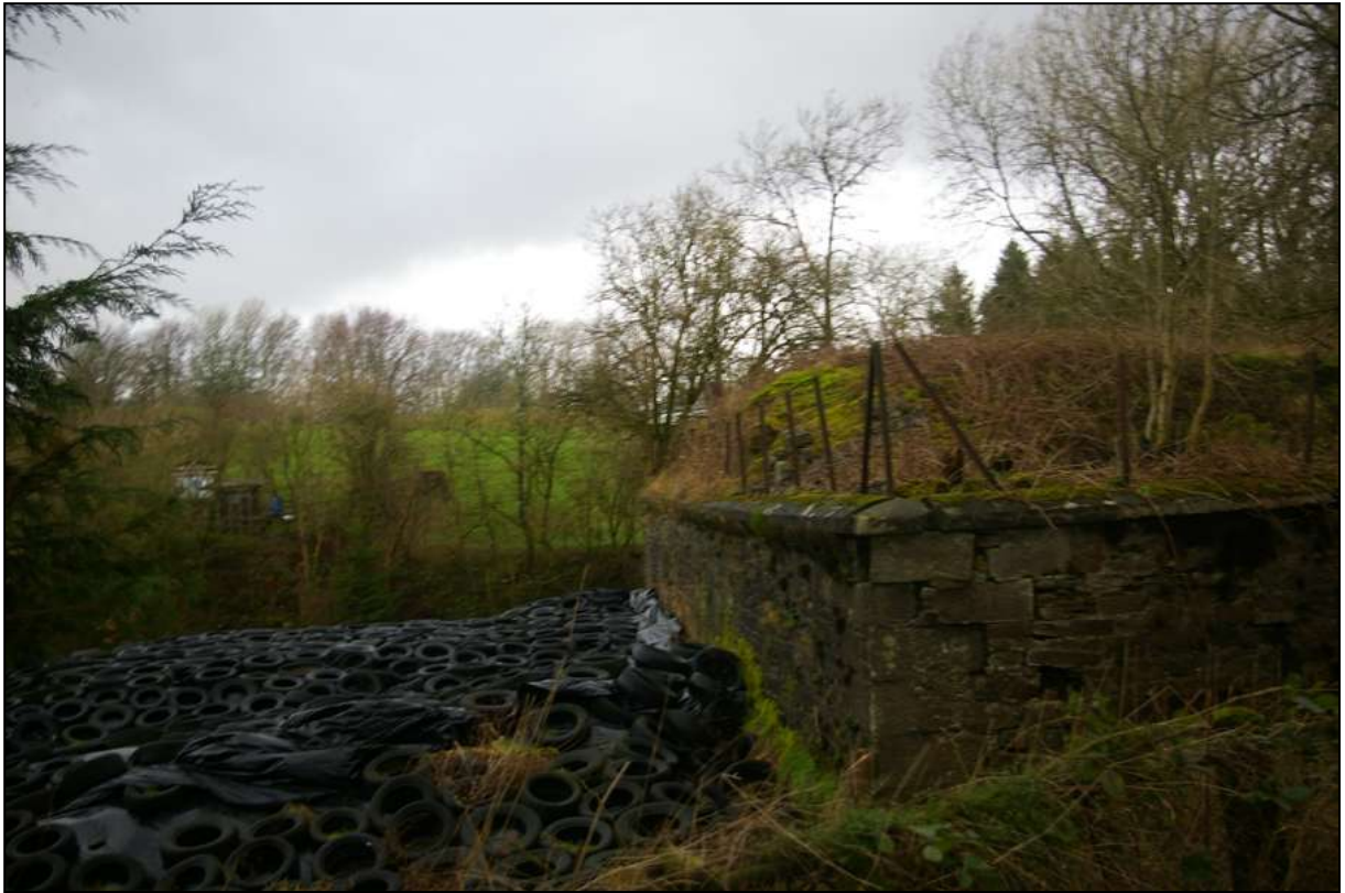
View of Harelawhil Limekilns; from the east, south-east.
