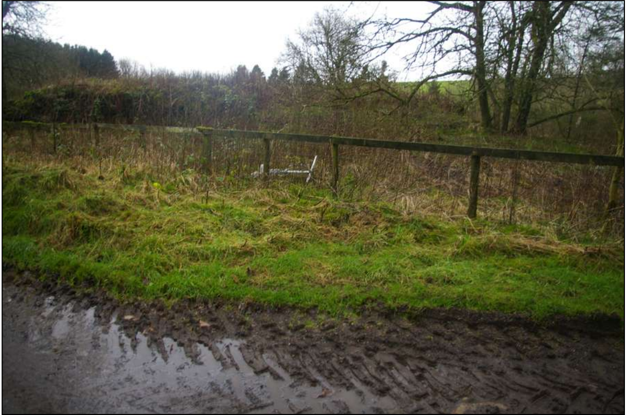
View of Harelawhil Limekilns; from the east, north-east.
