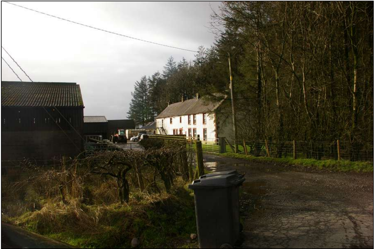
View along Cumcrook Farmhouse; from the north, north-east.
