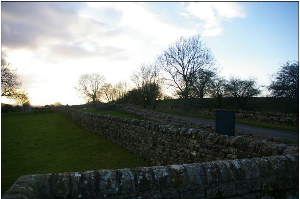
View north-west across the wall and one of the turrets/forts, near Banks; from the south-east.
