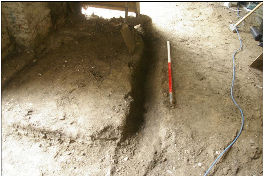
FIGURE 3: SERVICE TRENCH THROUGH LAYER (109); VIEWED FROM THE SOUTH (1M SCALE).
