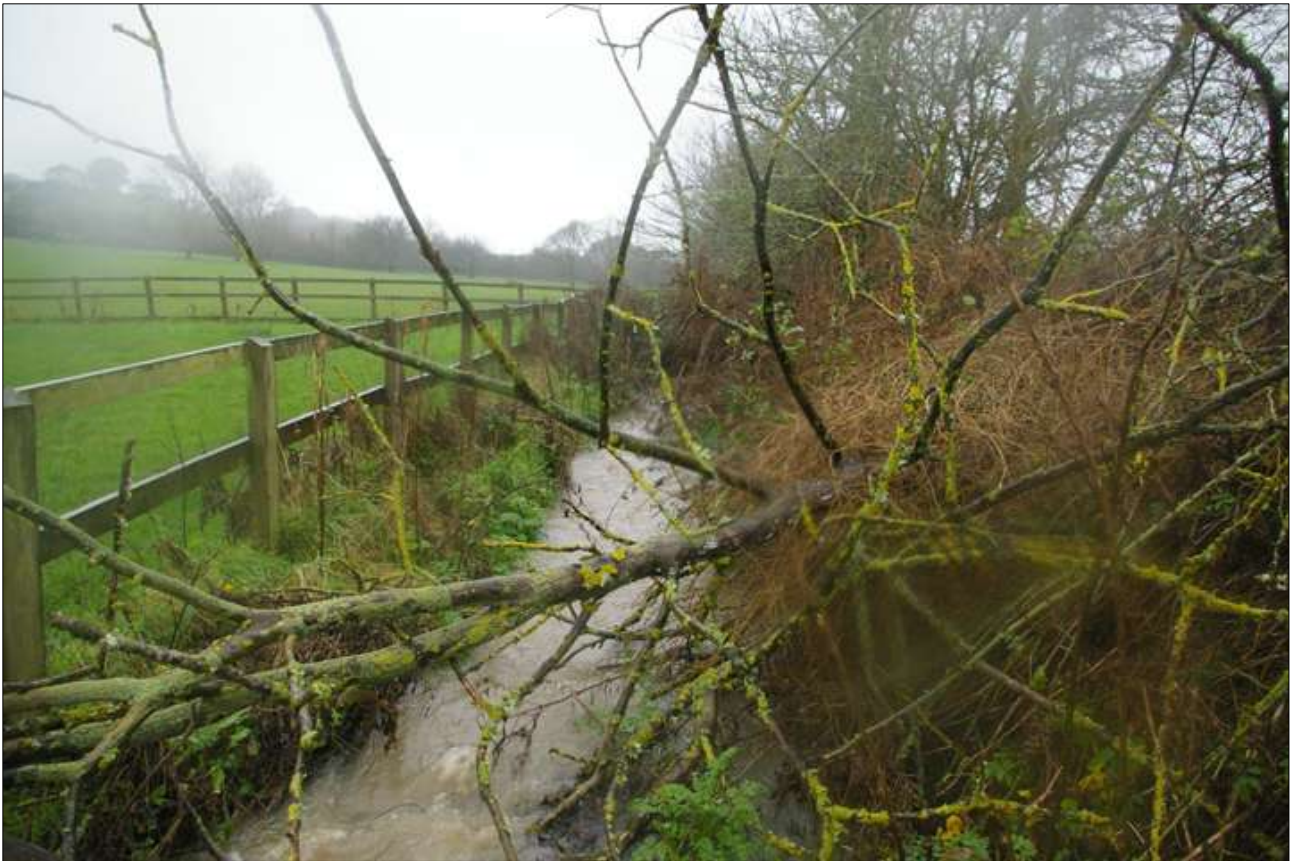
The south side of the southern boundary from its east end; looking west (no scale).
