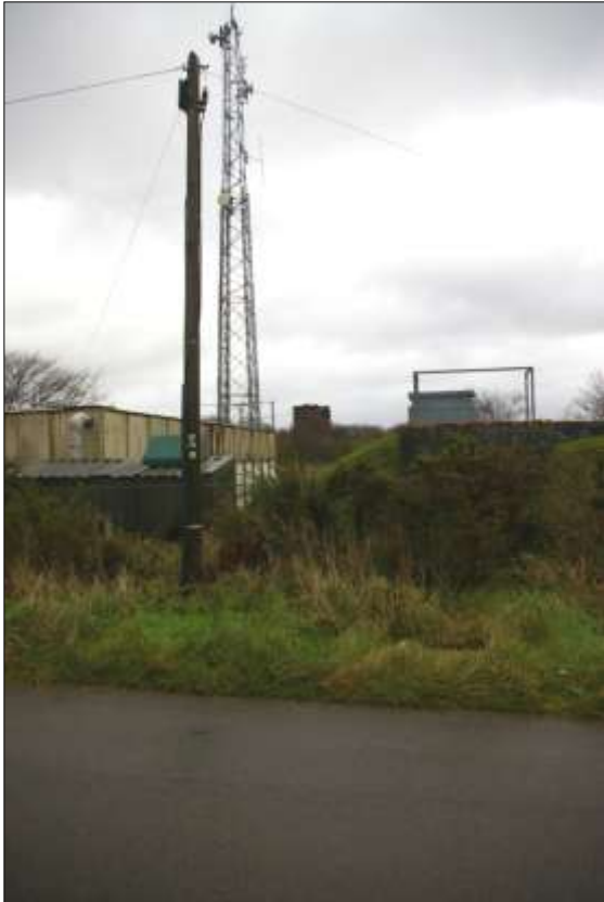
The telecoms mast and compound next to the west access to the Hingston Down Mine site; viewed from the west.
