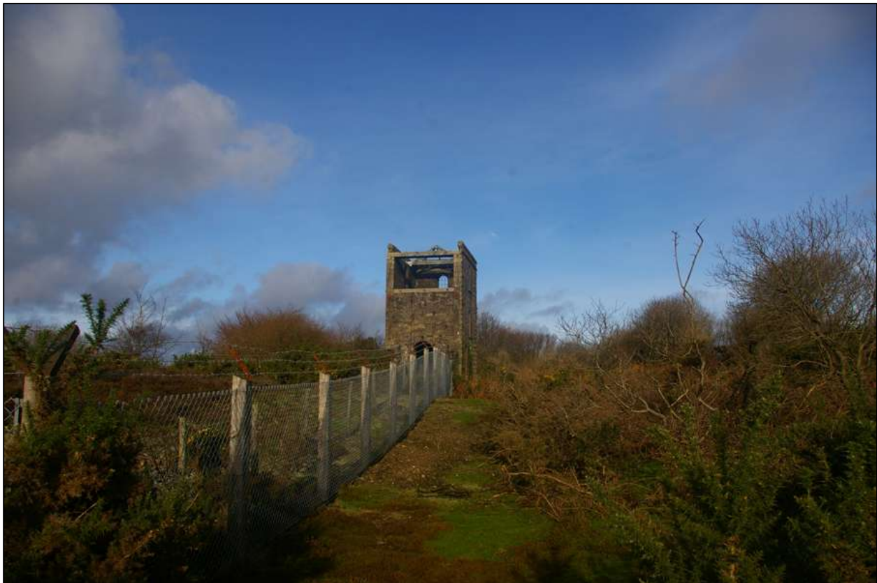
The enginehouse next to the fenced off mine shafts on the open moorland; viewed from the south-south-west.
