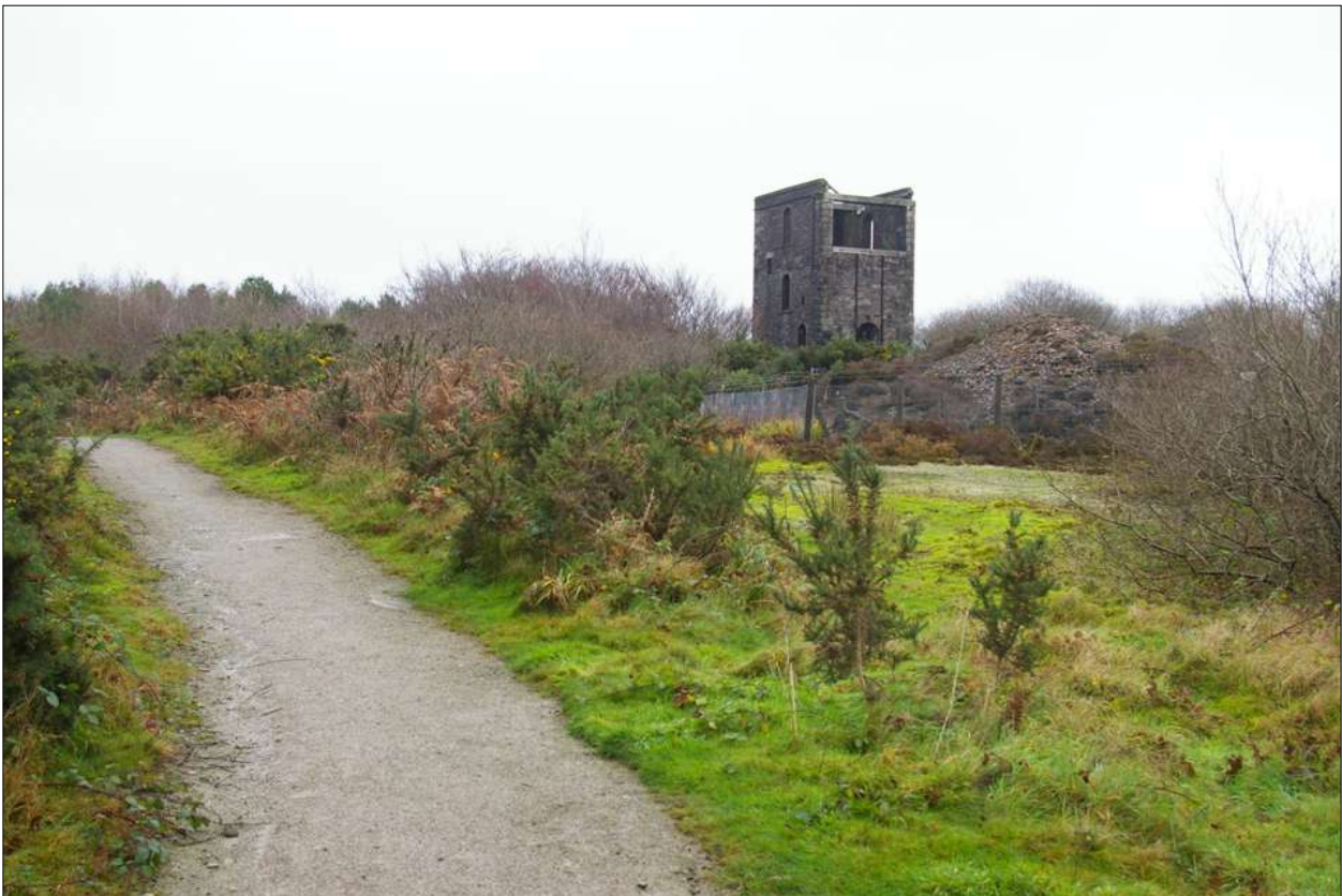
View across to the Listed enginehouse at Hingston Down Mine; viewed from the south-west.
