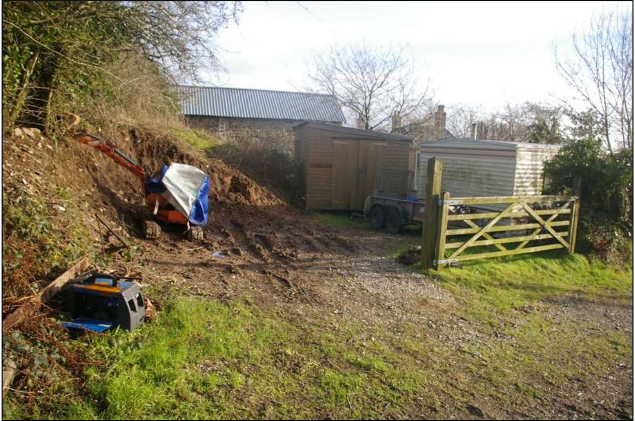
Salters Farmhouse from Old Mine Lane, opposite the south-eastern entrance in to the proposed development site. This shows the larger stone barns to the north-west of the farmhouse; viewed from the north-west.
