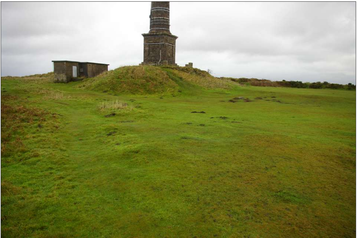
View across to the SAM enclosure on the top of Kit Hill, viewed from the south-west.
