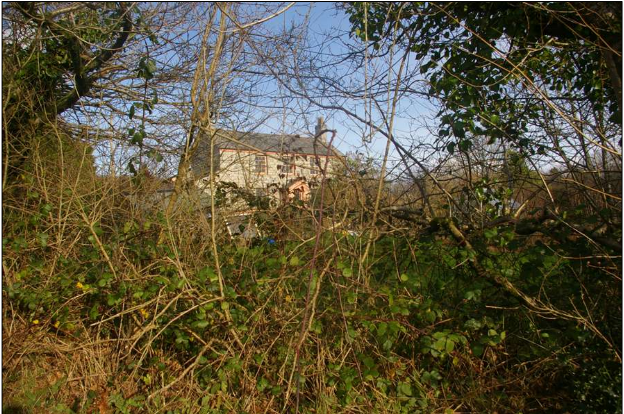
Salters Farmhouse, viewed through its garden hedge; viewed from the south-west.
