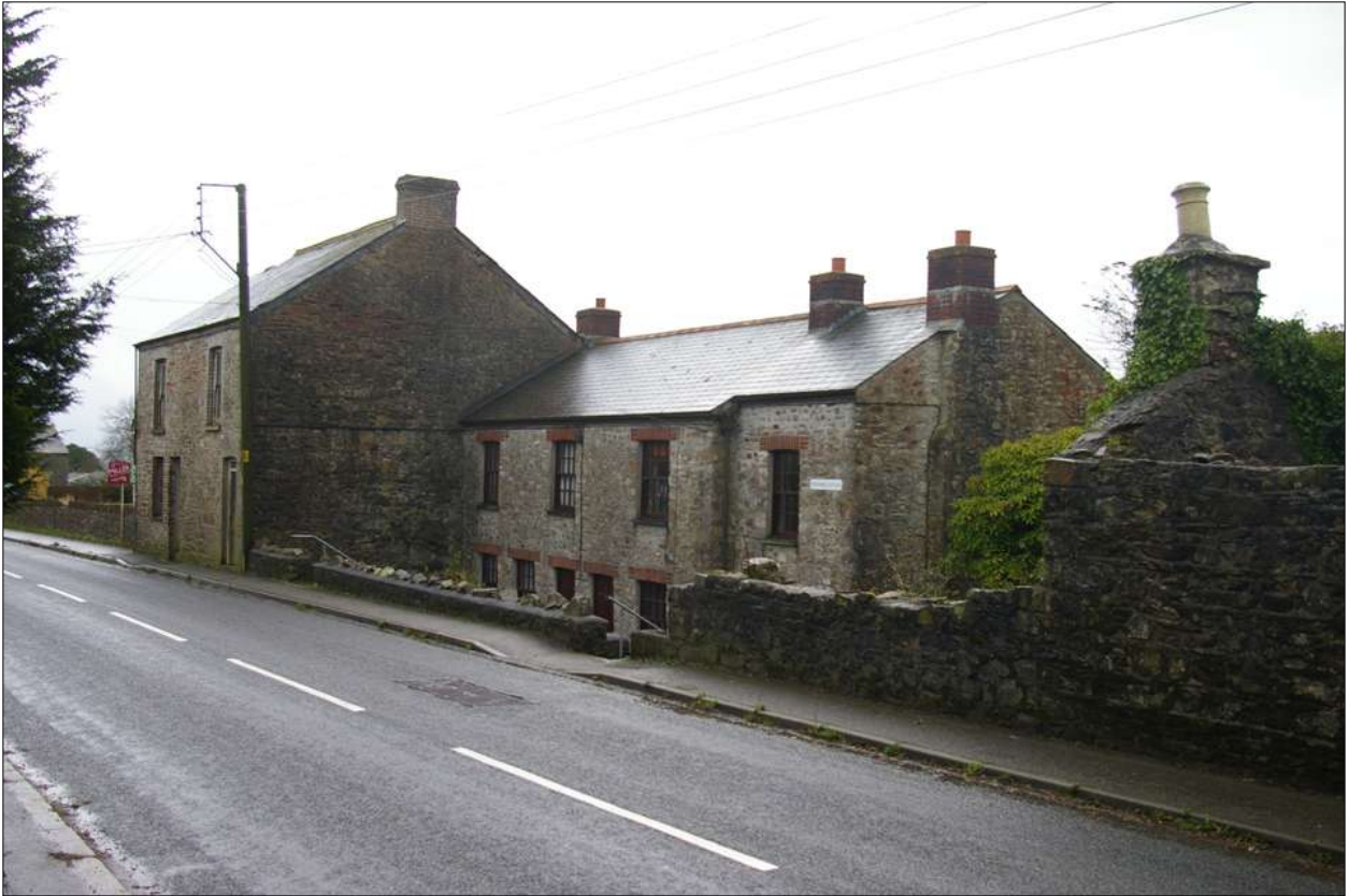
View of the GII Listed cottages in St Ann's Chapel, Candycroft and Vendor; viewed from the north-west.
