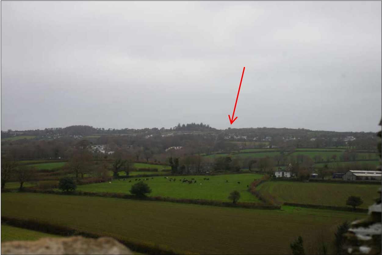
As above, detail. The Listed enginehouse at the Hingston Down Mine is indicated.
