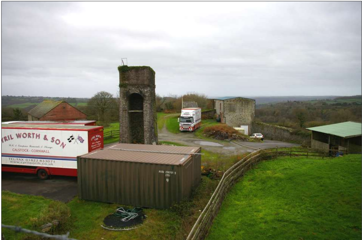
The watertower at East Calstock Mine, viewed from the north.
