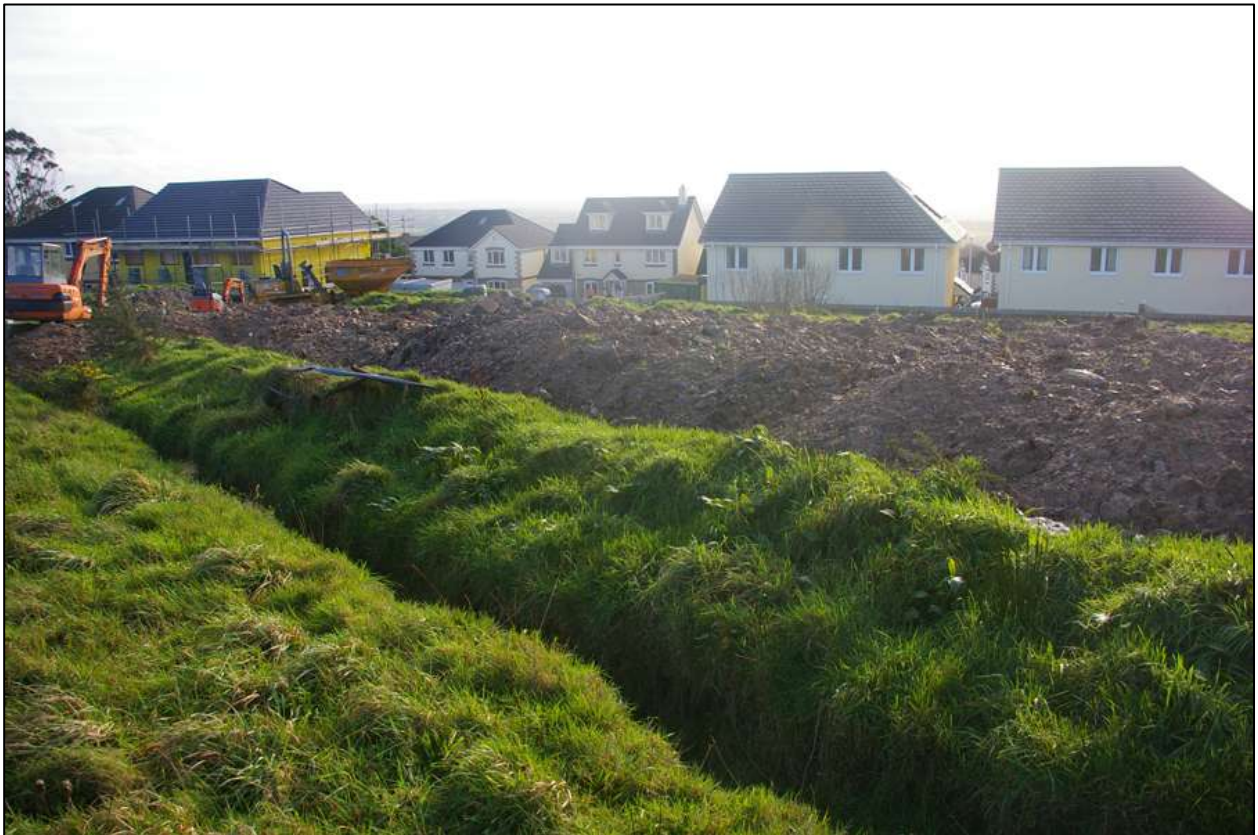
Modern housing development to the south of the site; viewed from the north-west.
