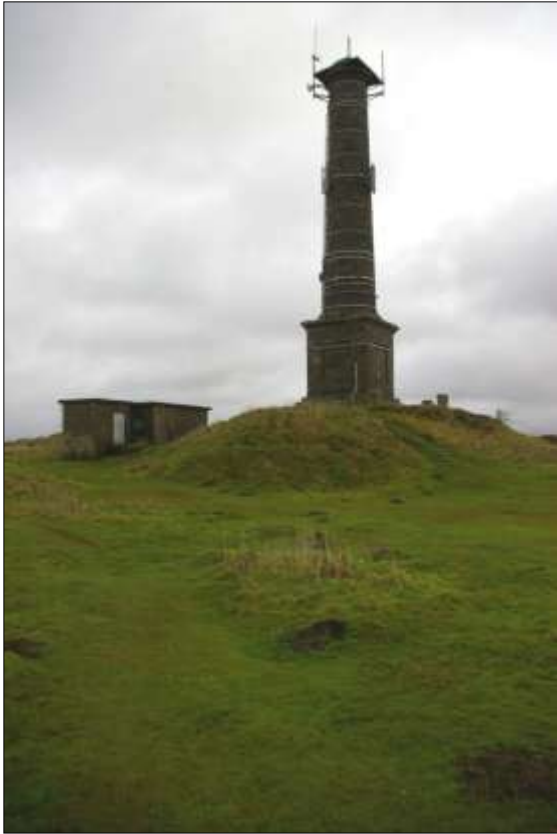
The needlessly elaborate chimney with telecom aerials at the summit of Kit Hill; viewed from the south-west.
