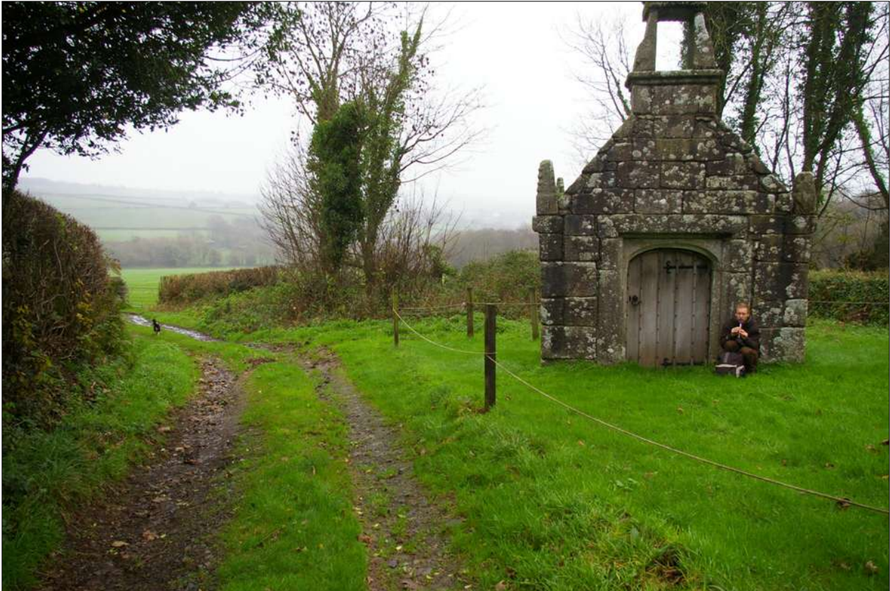
As above, viewed from the south.
