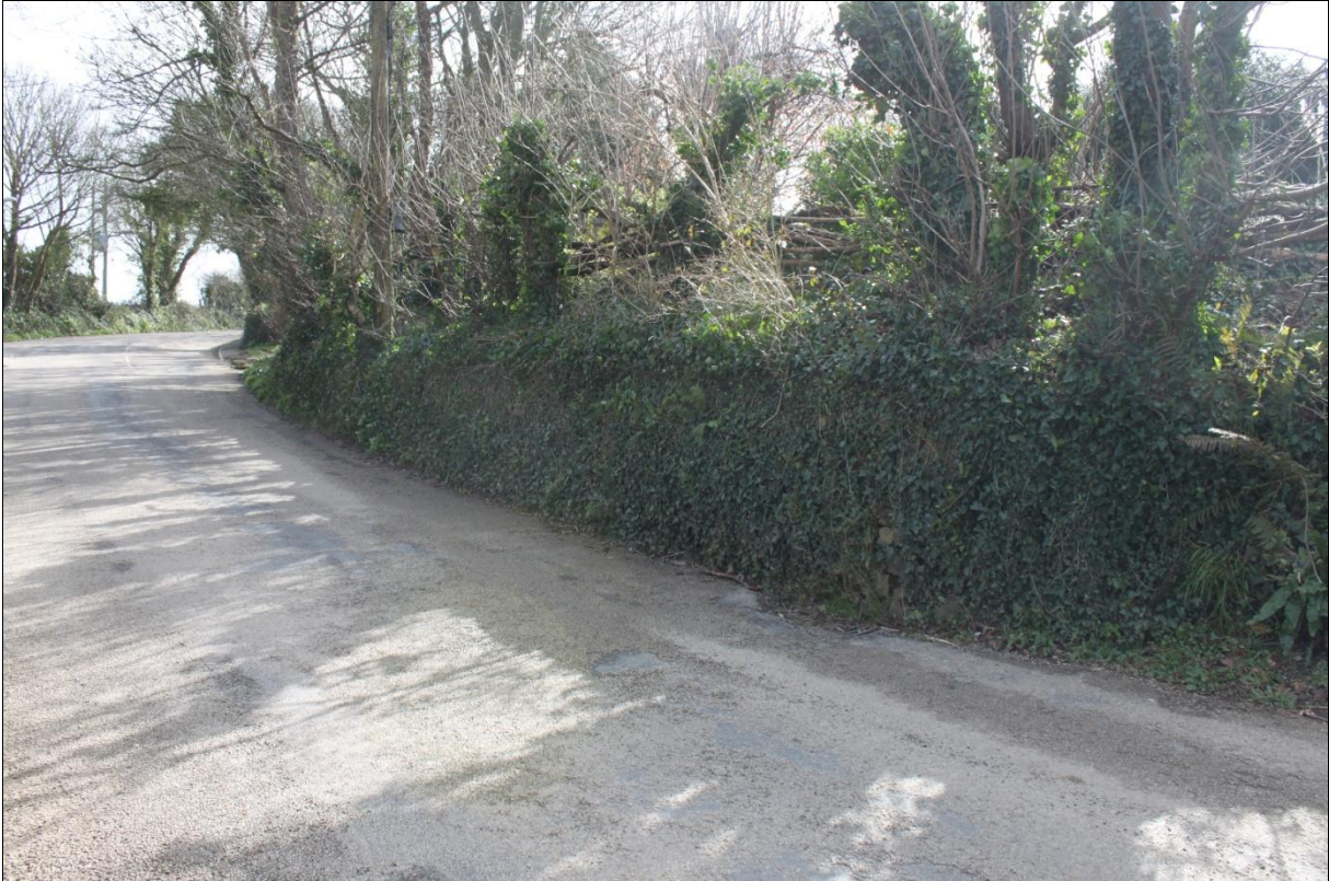
Boundary wall to Treloweth Cottages; viewed from the north-west.
