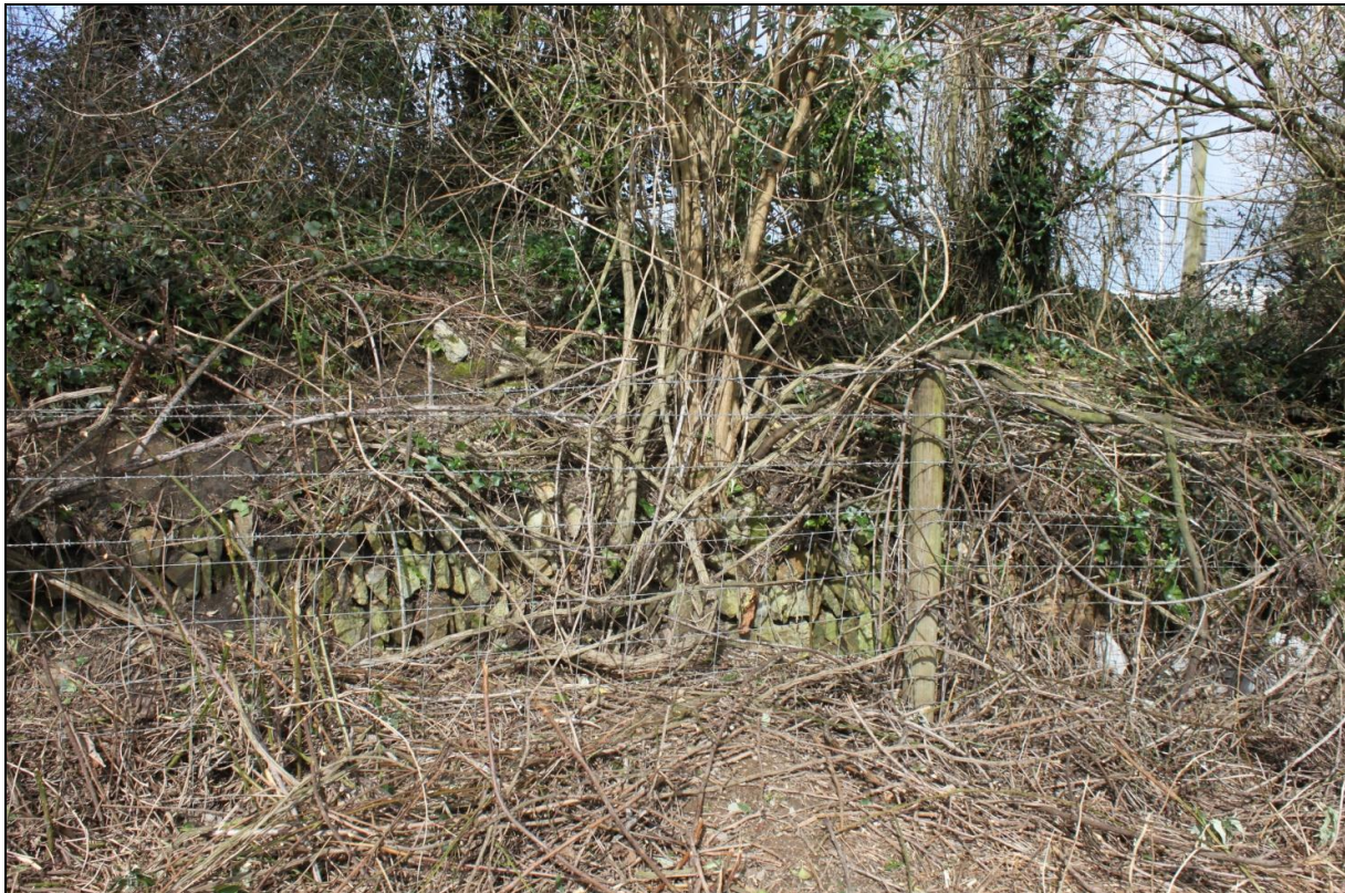
Northern boundary, stone wall; viewed from the south-east.
