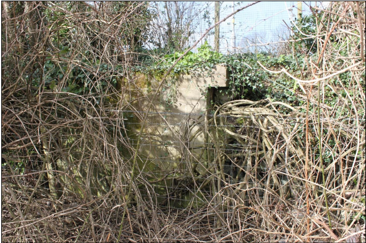
Concrete structure cut into north boundary; viewed from the south-east.
