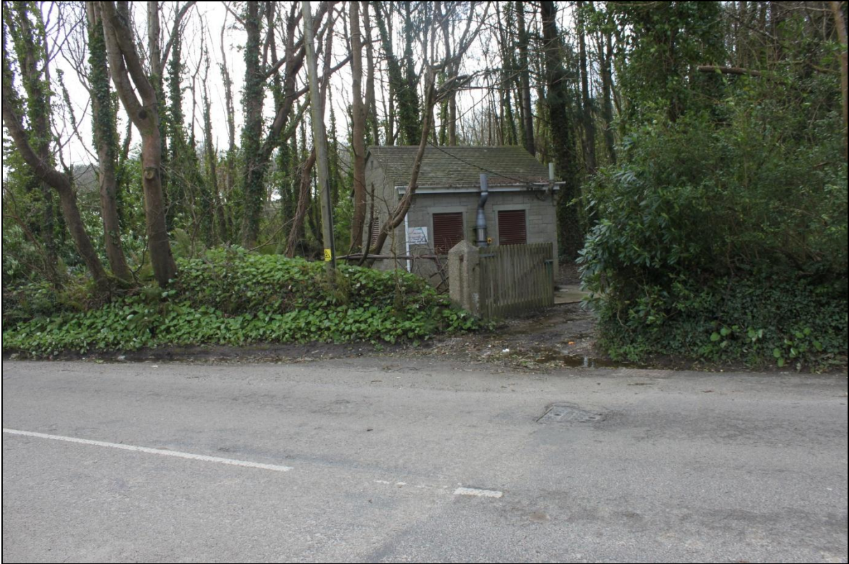
Pumphouse in woods; viewed from the north.
