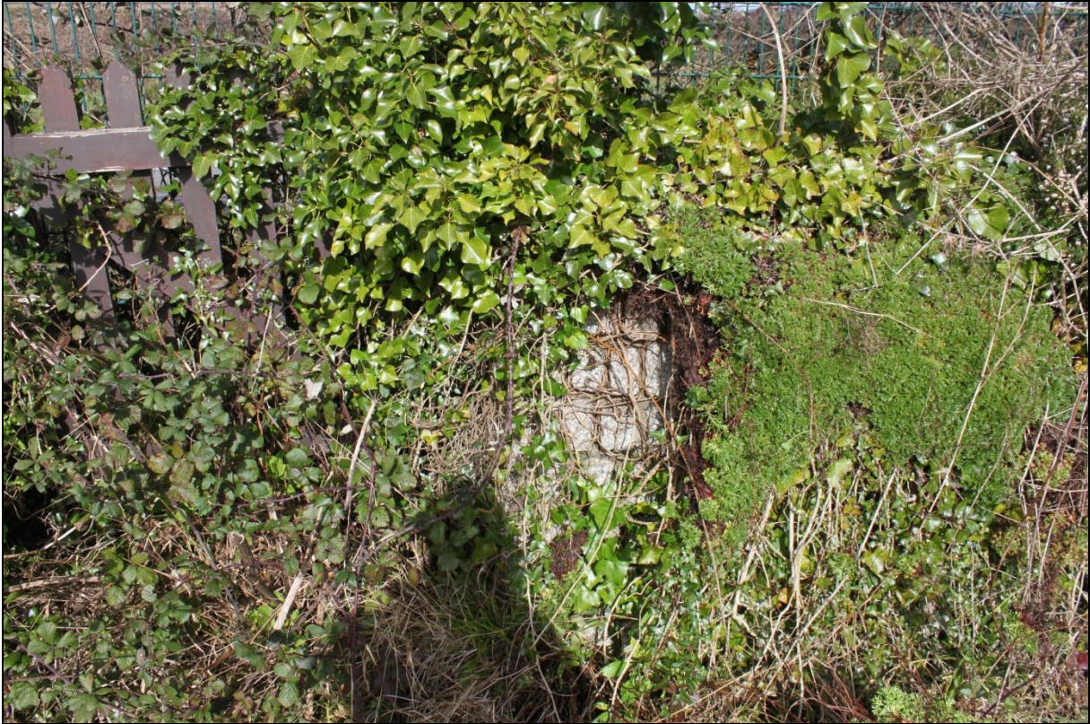
Detail of garden wall by gate; viewed from the south-west.
