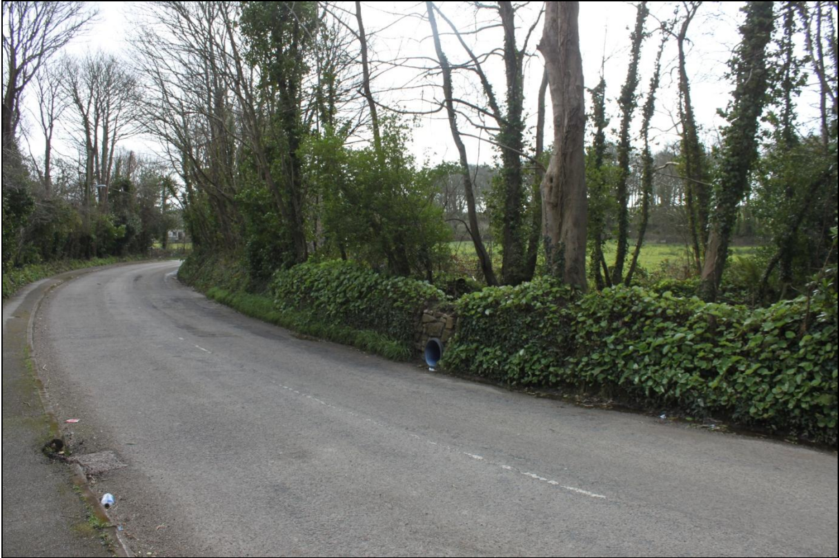
Recent drain/repair in southern/western boundary to road; viewed from the north.
