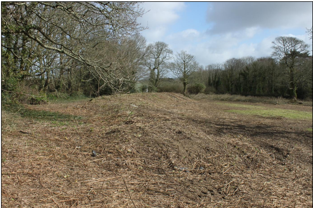
Earthen bund (containing contaminated soil) to east of field; viewed from the north-west.
