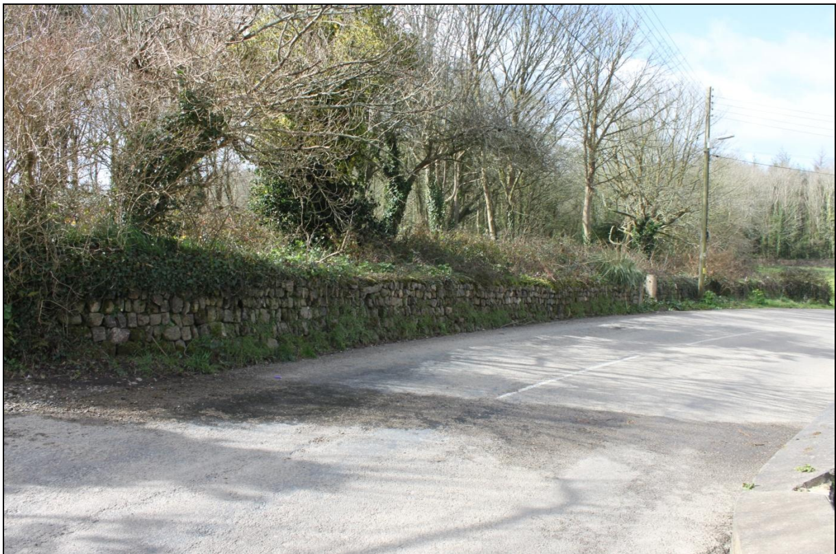
Boundary wall opposite Treloweth Farmhouse; viewed from the south-east.
