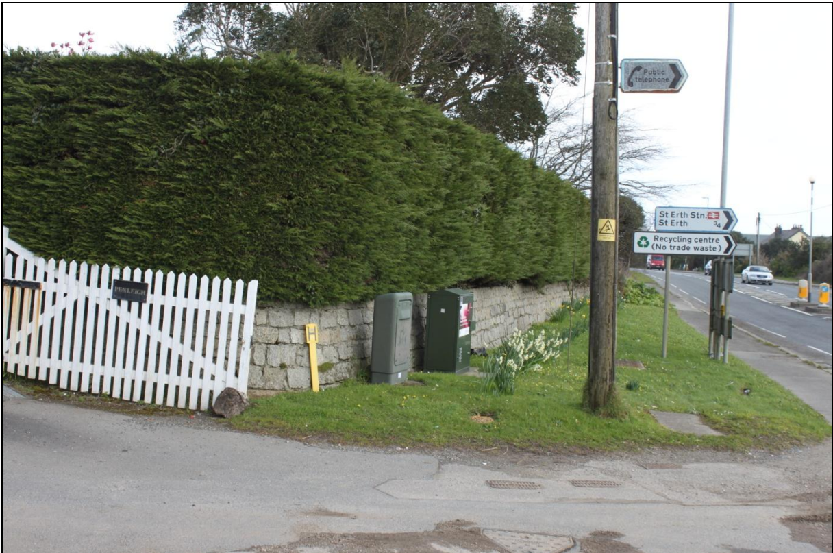
Boundary wall to Penleigh; viewed from the west.
