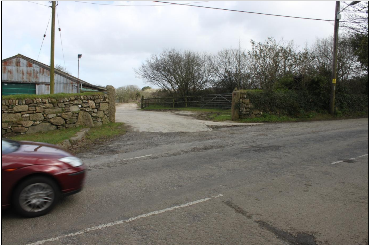
Rebuilt gateway into Treloweth farmyard; viewed from the south-west.
