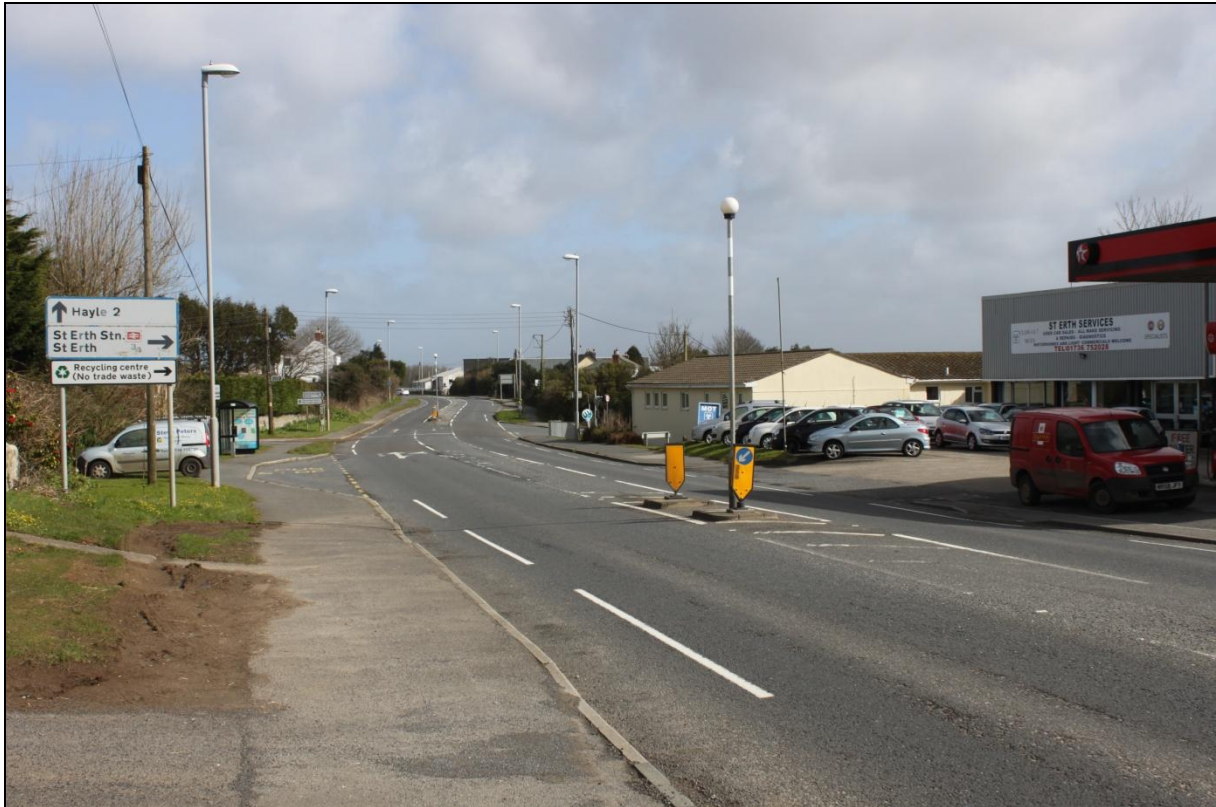
A30 showing junction; viewed from the south-west.
