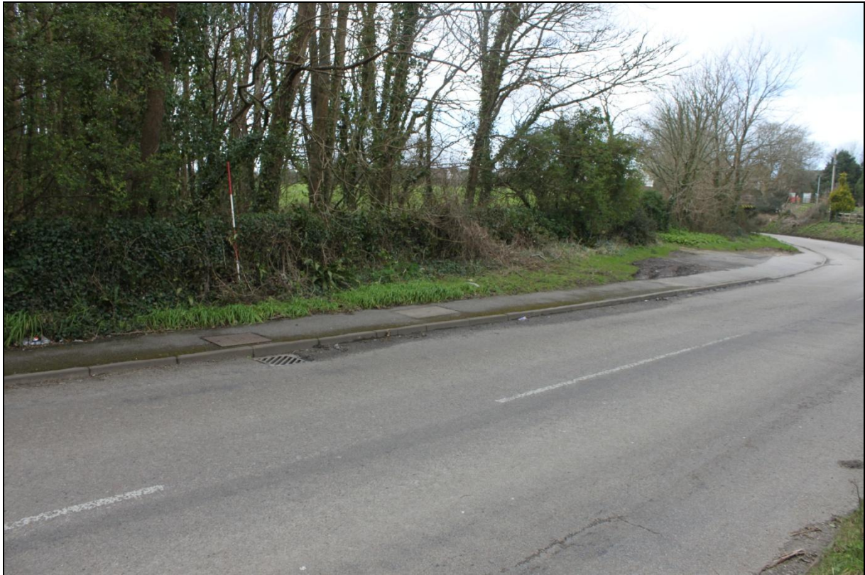
Stone wall/facing along road of woodland (general); viewed from the east (2m scale).
