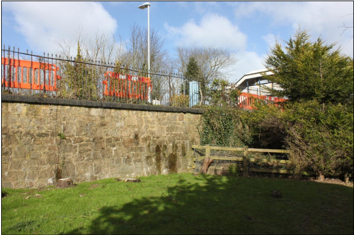
Platform retaining wall in Kingdom Hall plot; viewed from the south.
