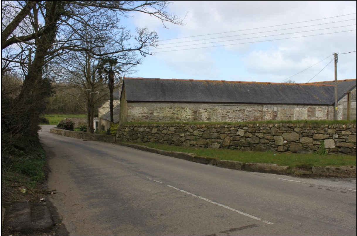
New boundary south of Treloweth; viewed from the south.
