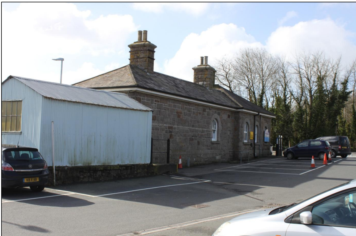
St Erth Station; viewed from the north-east.
