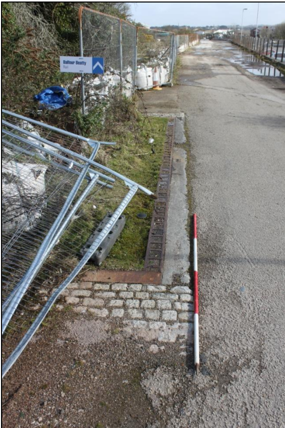
Footing for another structure to the west; viewed from the west (2m scale).
