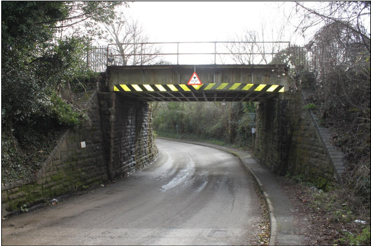
Railway bridge; viewed from the north-west.
