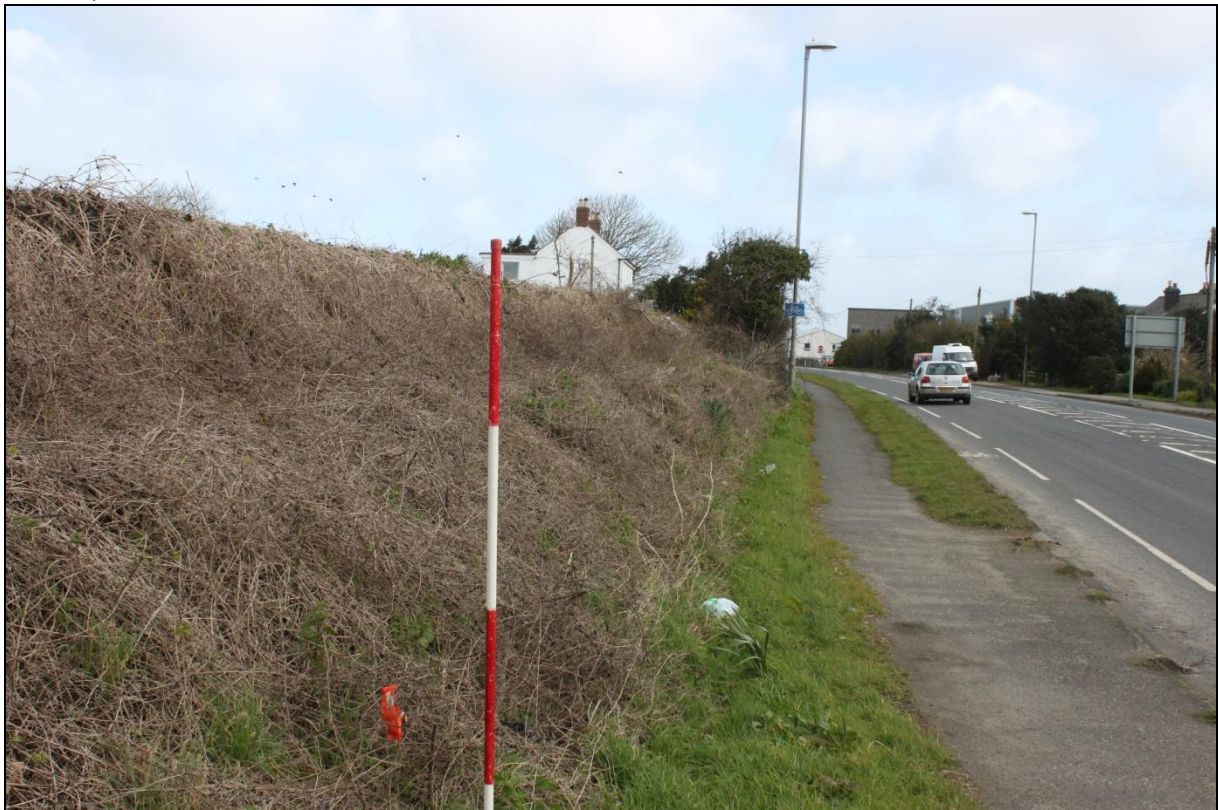
Hedgebank (and pipelines) against field to the north; viewed from the south-west (2m scale).
