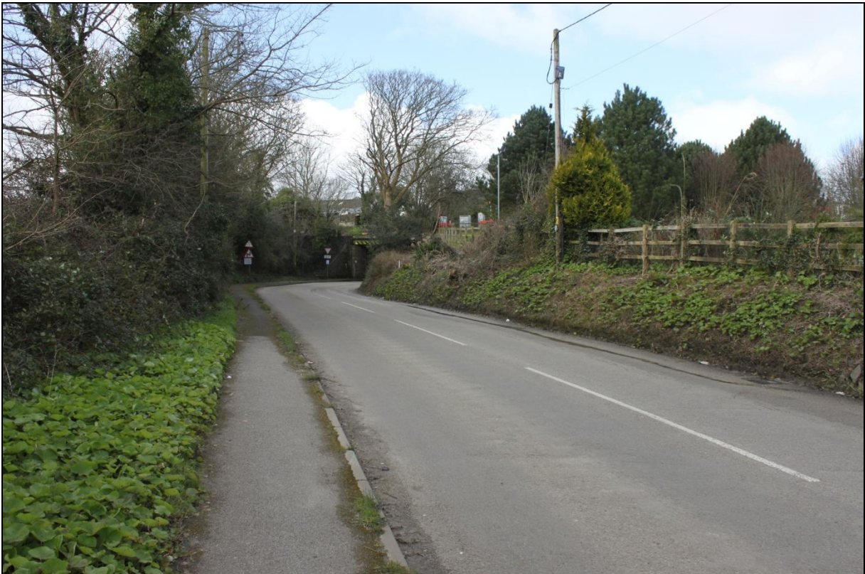
Approach to railway bridge; viewed from the east.
