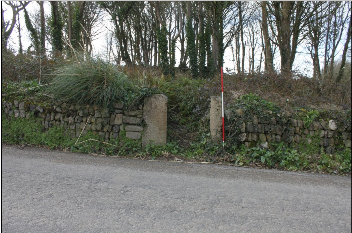
Gateway (possibly forced) in wall opposite Treloweth Farmhouse; viewed from the north-east (2m scale).
