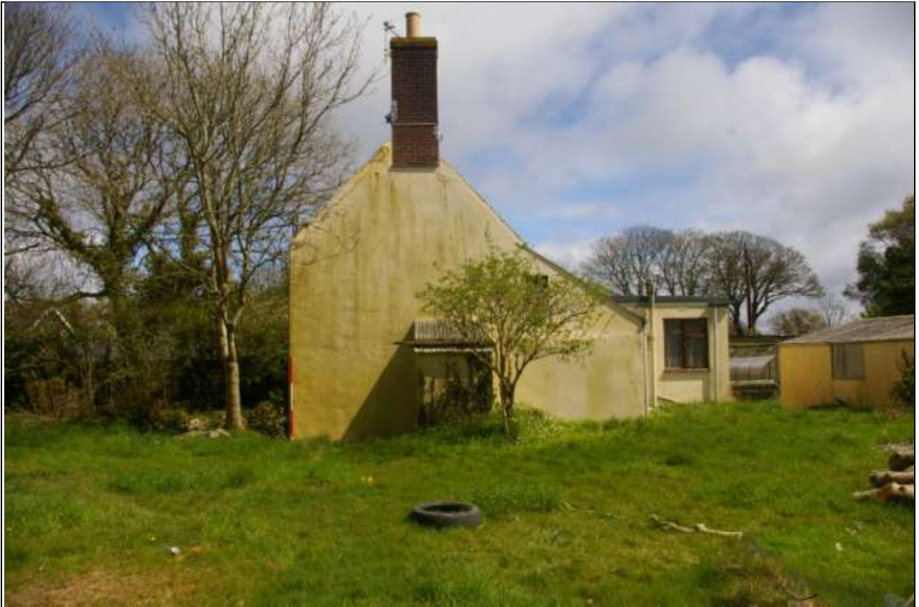
The west elevation of the farmhouse; from the west (2m scale).
