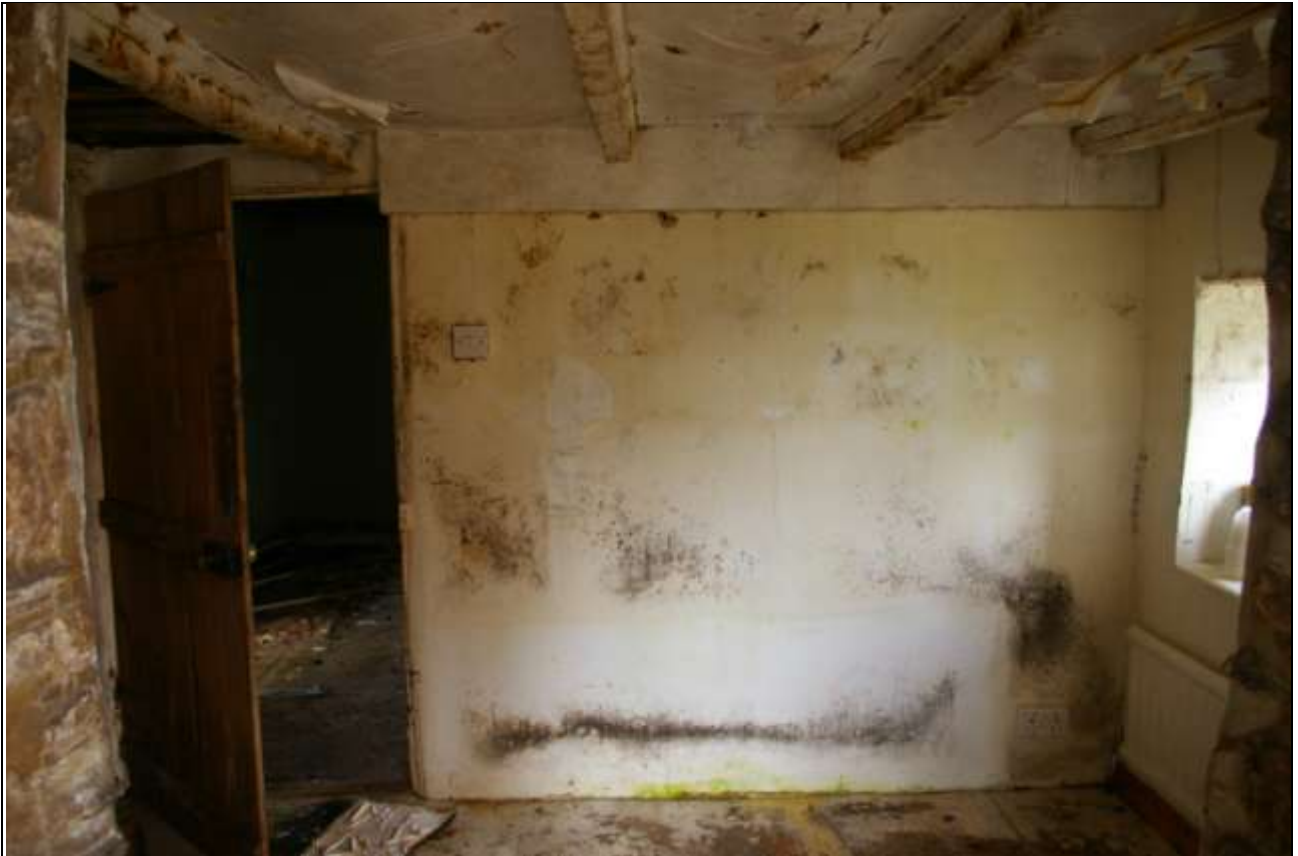
Room 4, with low ceiling, small narrow joists, possibly original, with plasterboard between. The door frame suggesting a change in status between the main range and 19 th century extension; from the south.
