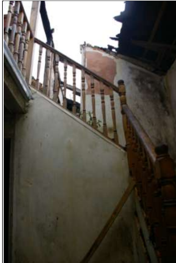
Room 2, the hallway, leading up to Room 11, the landing; showing the modern 20 th century staircase and the lost roof; from the west.
