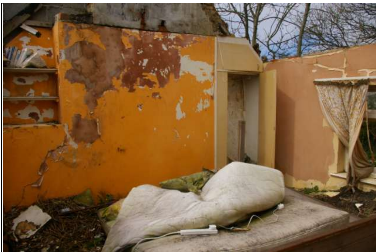
Room 14, showing the western chimney stack, possibly wholly 20 th century in date, as much of elevation is rebuilt in concrete block, cupboard to north of stack, shelves to south may block a former window opening; from the east, south-east.
