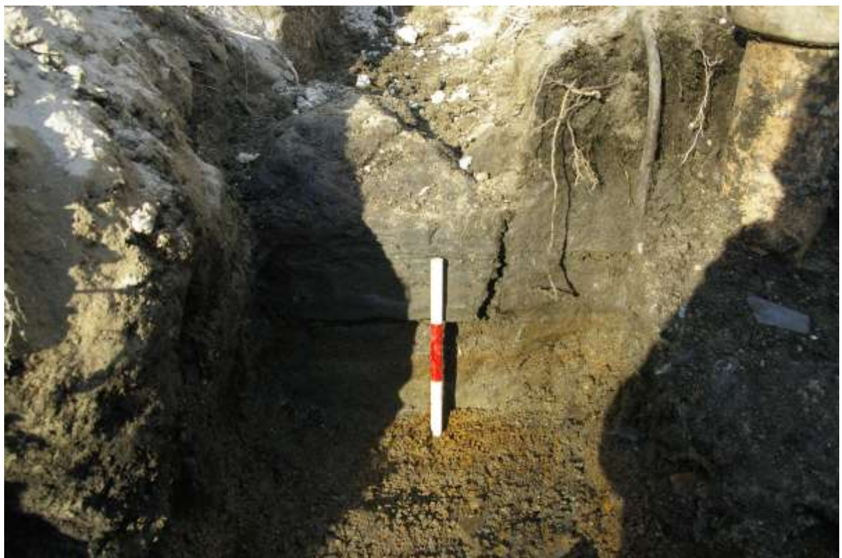
Figure 3: South facing elevation of leat wall {015}, Area 01; viewed from the west (0.30m scale).
