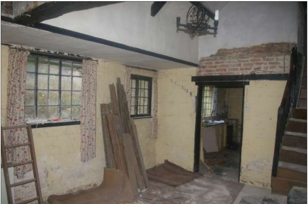
Figure 16: Room 7 from the south west showing doorway to Room 3.
