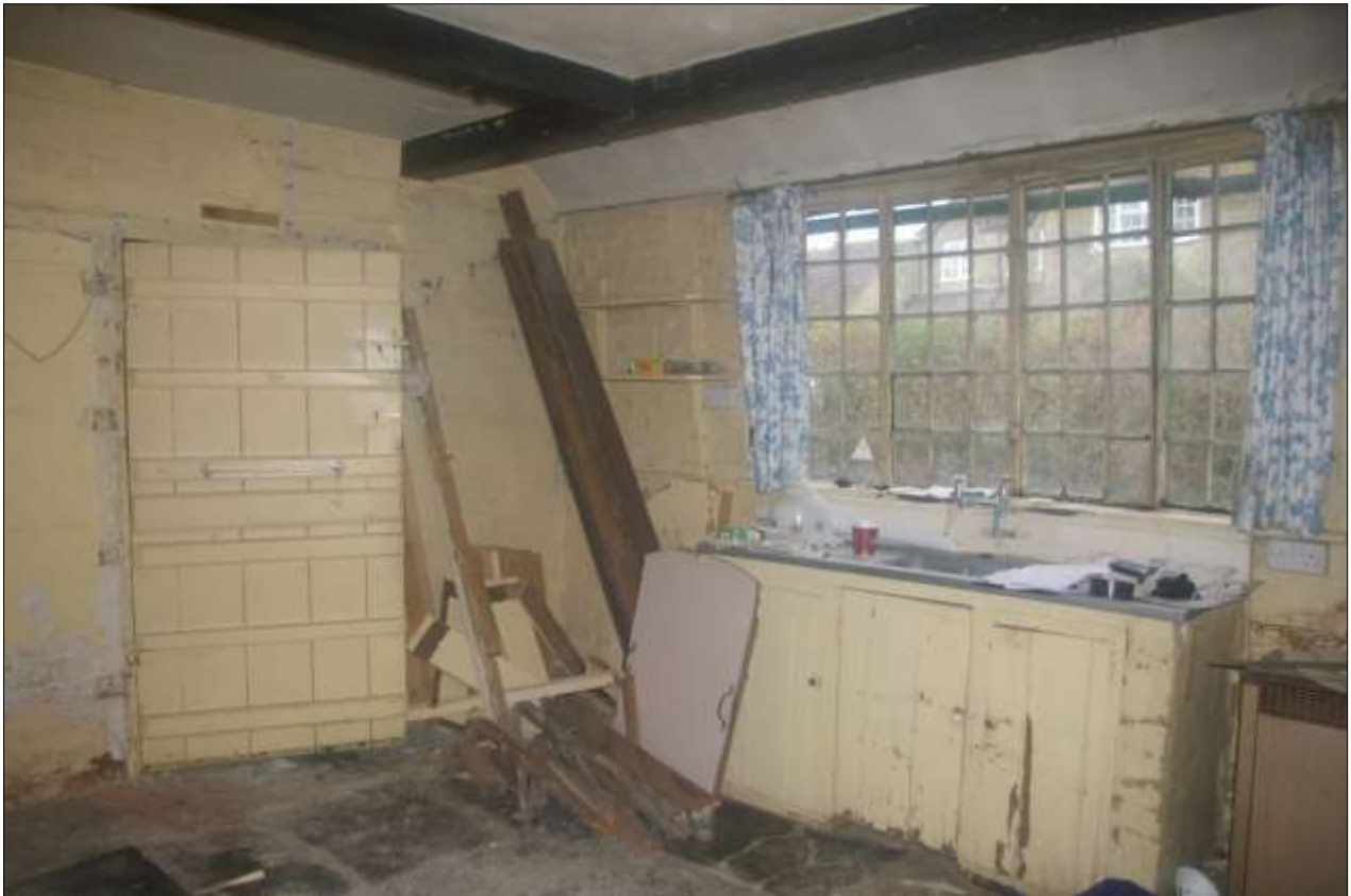
Figure 13: Room 3 from the south east showing former external 'stable' door.
