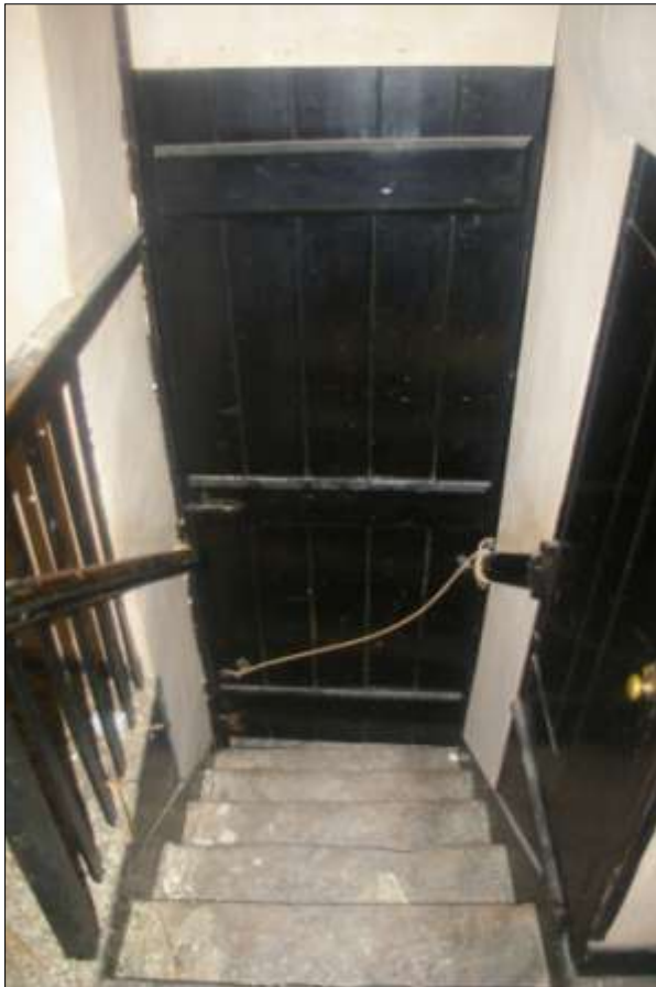
Figure 19: Stairwell from the first floor.
