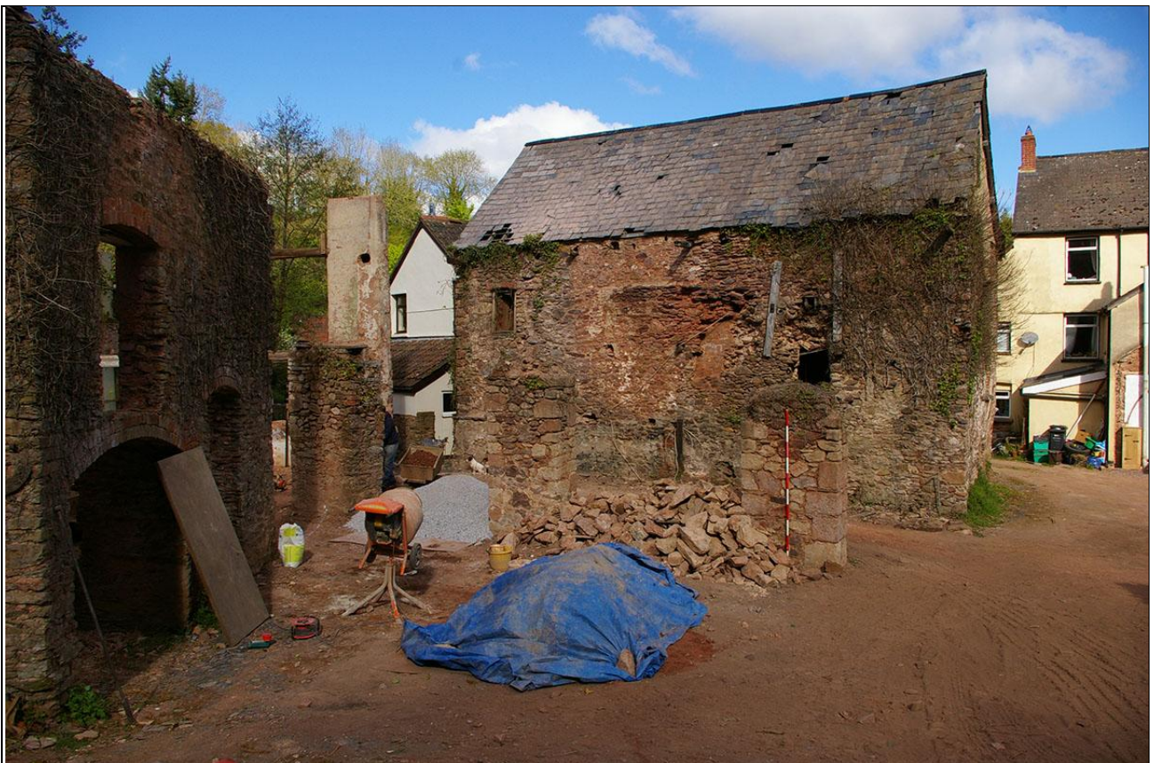
The adjacent wheel pit bracing walls/piers; from the east (2m scale).
