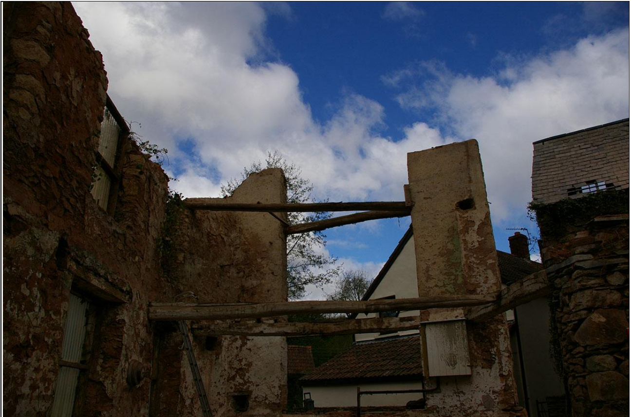
The dragon tie bracing and timbers bracing the large opening at the west end; from the east.
