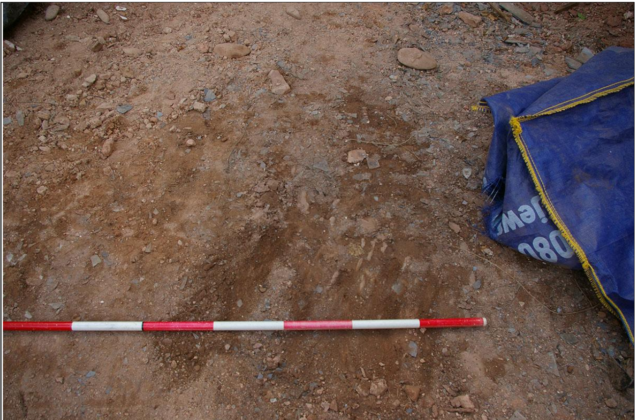
Small section of surviving slatestone cobbled floor to the north-east corner of the main compartment of the workshop, against the dividing stone partition wall; from the south (2m scale).
