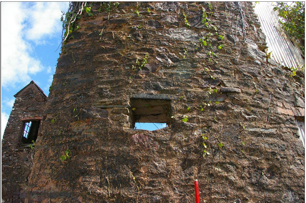
Socket in wall of the south-west corner; from the south (2m scale).
