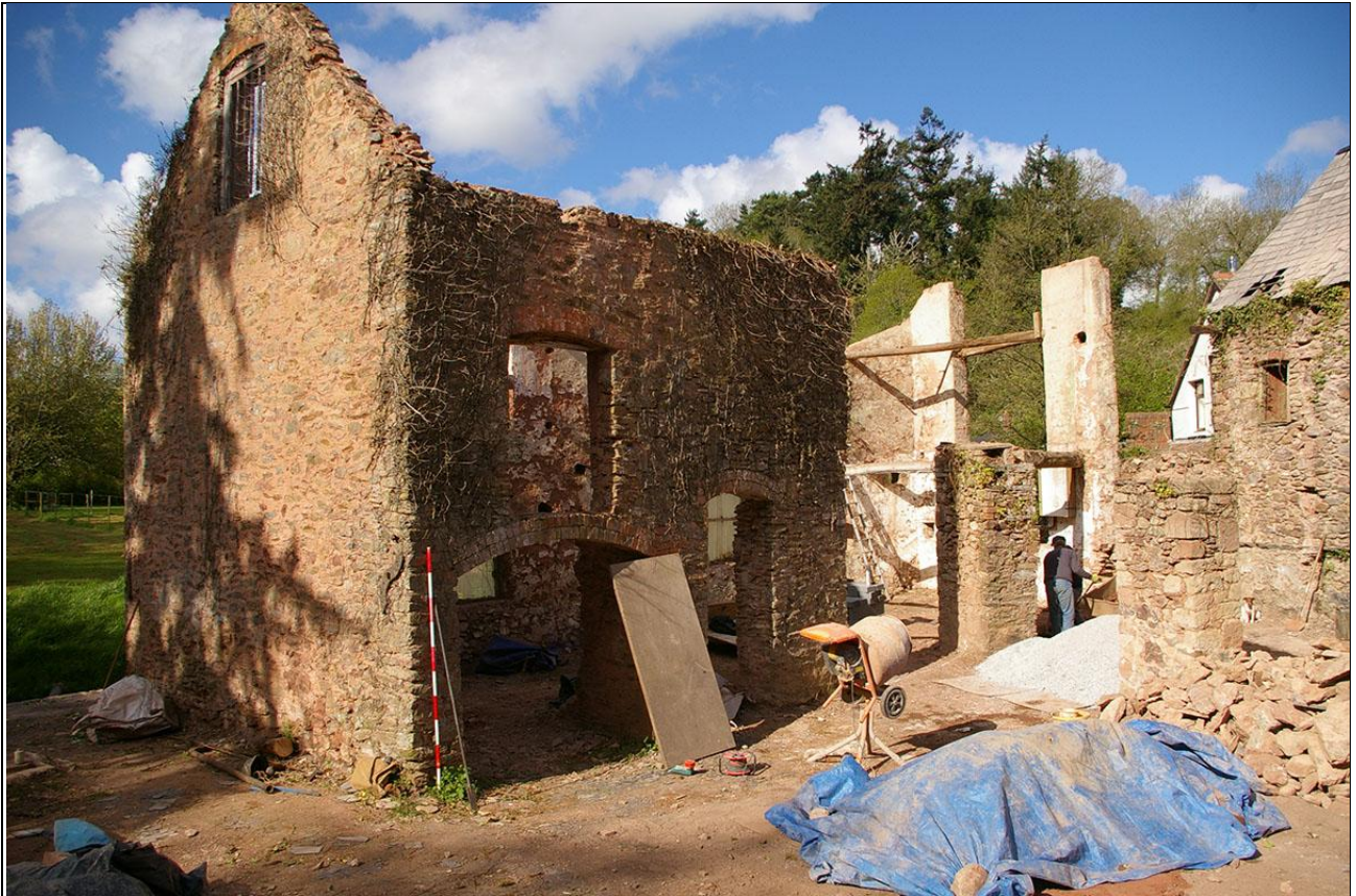
The east elevation of the workshop; from the north-east (2m scale).
