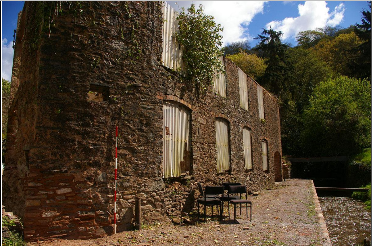
The south elevation; from the south-west (2m scale).
