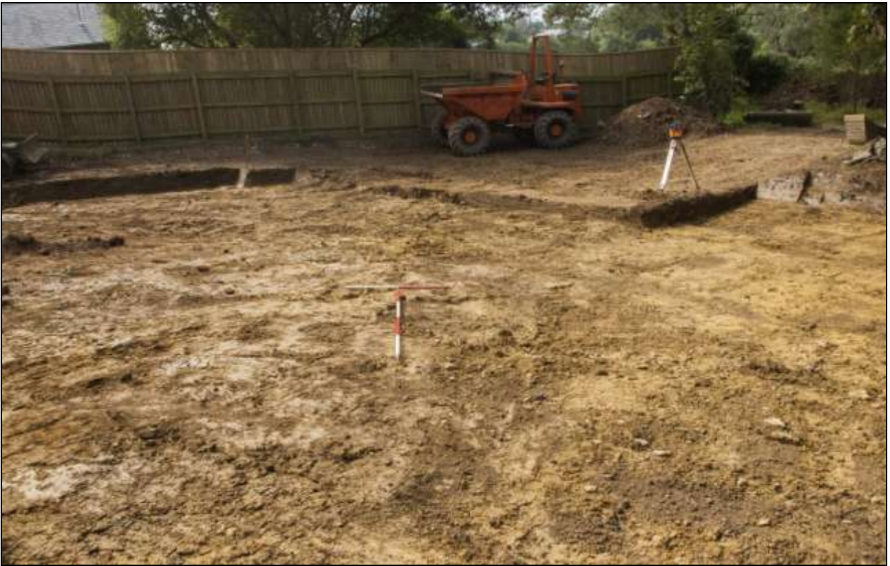
Figure 2: The site strip, viewed from the north-east (scale 1m & 2m).
