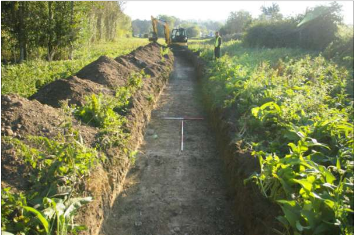
TRENCH 5, POST-EXCAVATION; VIEWED FROM THE WEST (1M & 2M SCALES).
