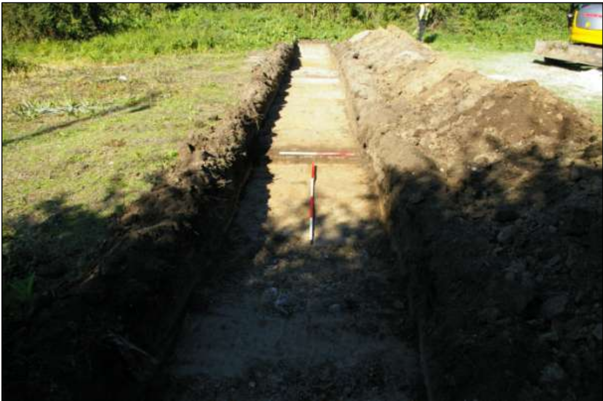
TRENCH 2, POST-EXCAVATION; VIEWED FROM THE SOUTH (1M & 2M SCALES).
