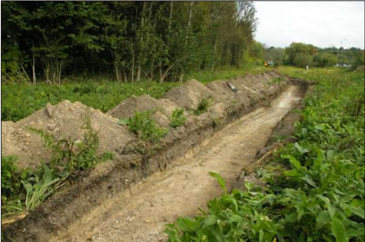
TRENCH 5, SOUTH FACING SECTION, OBLIQUE; VIEWED FROM THE SOUTH-WEST (2M SCALE).
