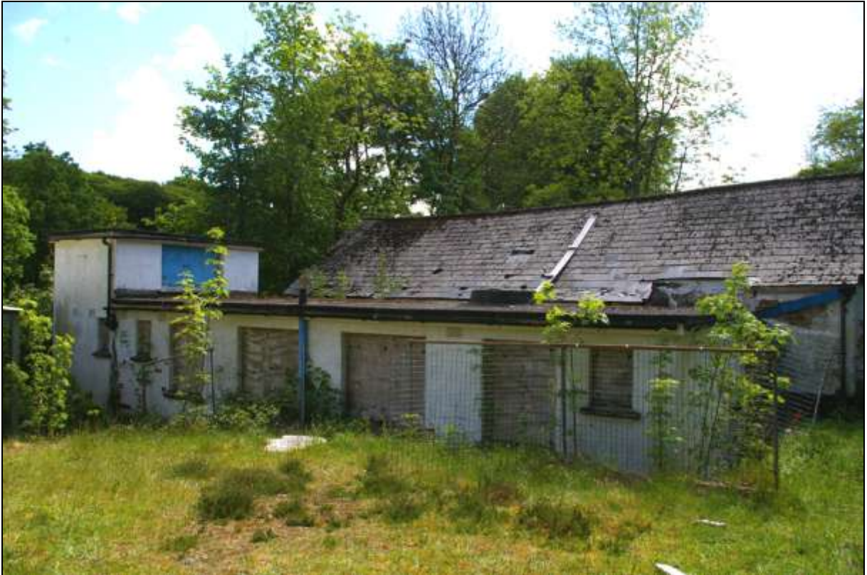
Figure 7: The north-facing elevation of the 20 th century flat-roofed, brick-built school buildings in 2012, viewed from the north-west.
