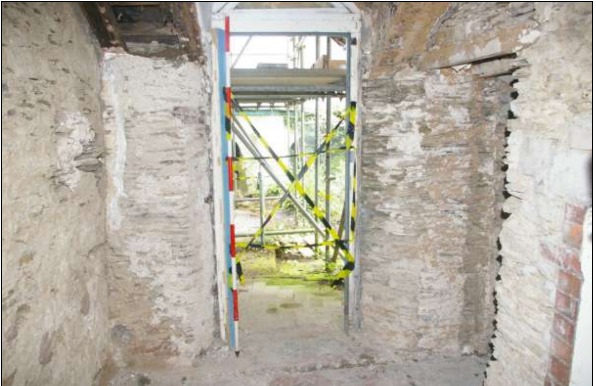
Figure 14: The external door to R9 in 2015, with blocked window splay to the left; viewed from the east (scale 2m).
