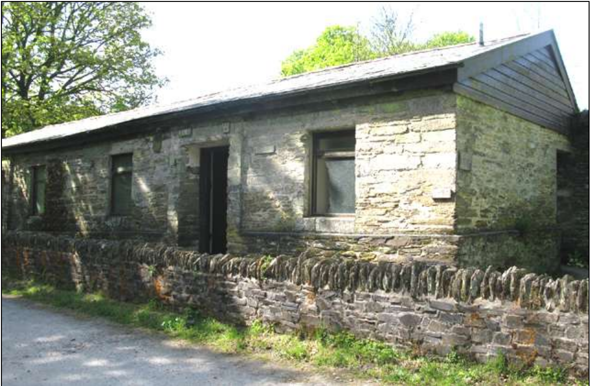
Figure 18: The east-facing elevation of the toilet block in 2012; from the north.
