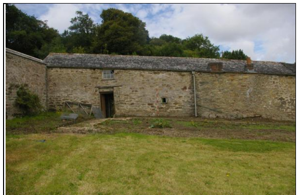
Figure 20: South end of the east elevation; from the east.
