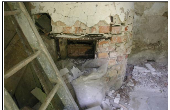
Figure 140: Detailed view of the copper; from the west.
