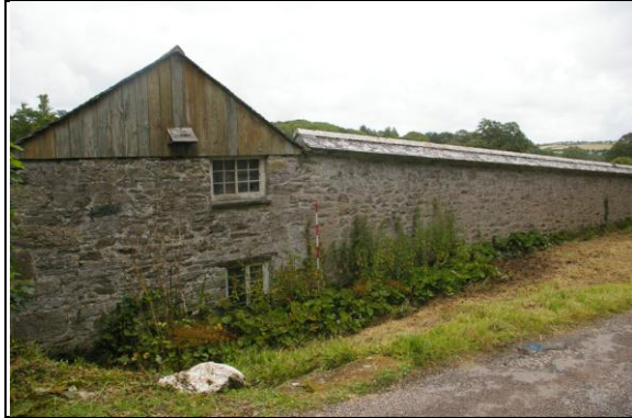
Figure 14: The south elevation and garden wall; from the south-west.
