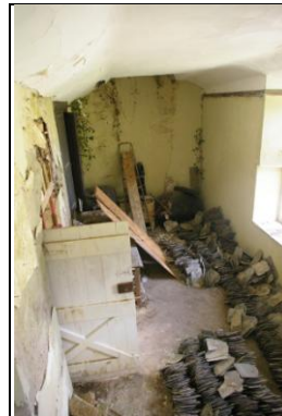
Figure 83: Room M, Section 4; from the south, south-west.
