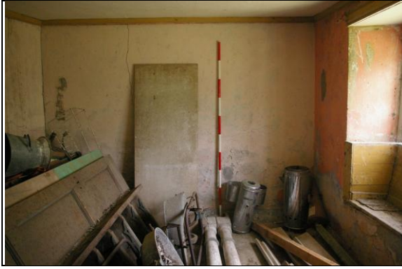
Figure 141: The south wall (stone partition, to first floor height to Room E) of Room H, Section 3; from the north.
