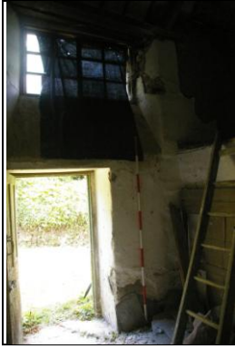
Figure 133: The doorway and window above in the west wall of Room E, Section 2; from the east, south-east.
