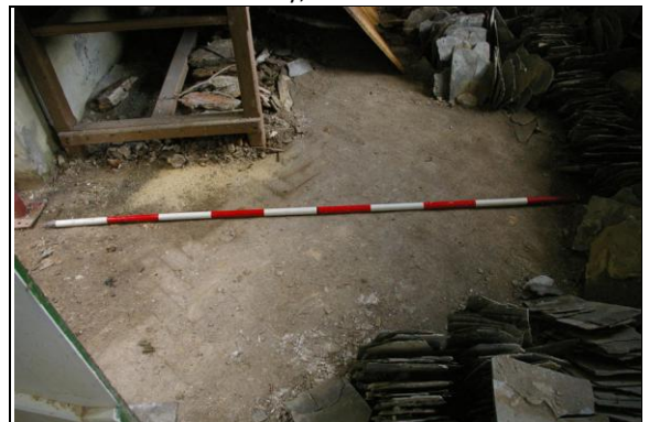
Figure 92: The parquet floor in Room M, Section 4; from the south.
