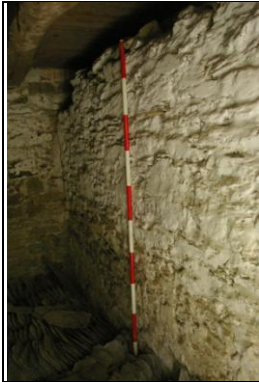
Figure 94: The stone partition wall, to first floor height only, between Room L and F; from the west, north-west.
