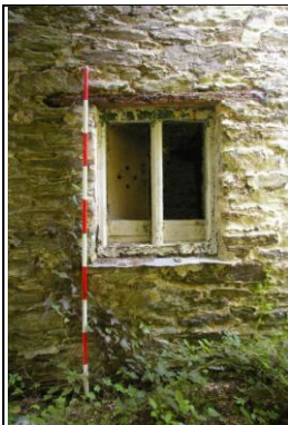
Figure 40: The mullion window in the animal house, Room L; from the west.
