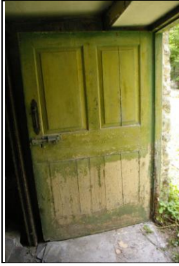
Figure 61: The door to Section 3; from the north.
