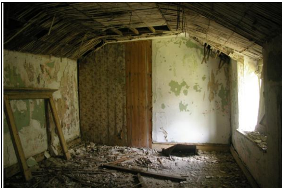
Figure 63: View of Room I, in Section 3; from the north, north-west.
