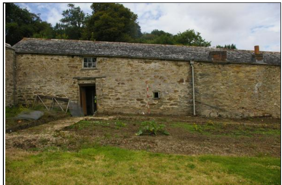
Figure 19: Section 1 running into Section 2; from the east.
