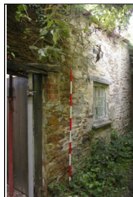
Figure 36: The west elevation of Section 4; from the north, north-west.
