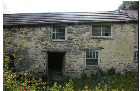
Figure 44: The west elevation of Section 3; from the west.
