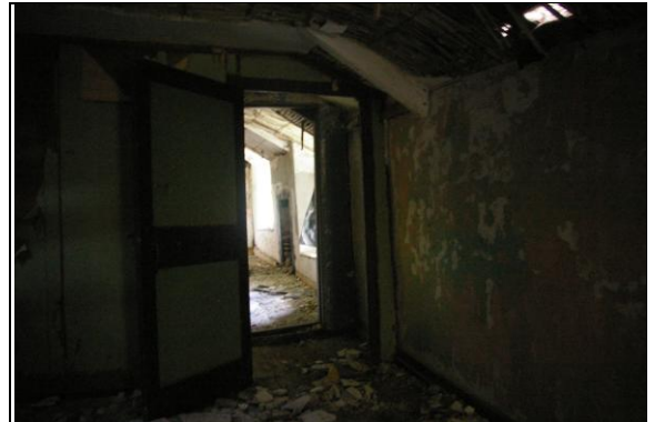
Figure 74: View through to Room I, from Room J, in Section 3; from the north, north-east.
