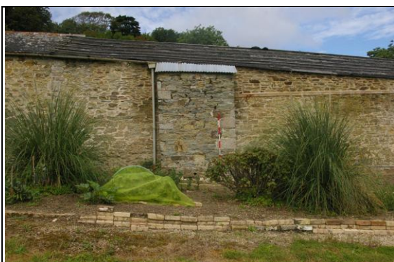
Figure 24: Detail of the Section 3 chimney stack; from the east.
