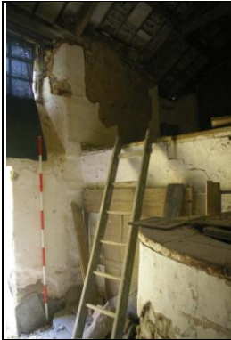
Figure 134: The ladder to the raised area in Section 2, formerly the first floor, before conversion to a laundry; from the east, south-east.
