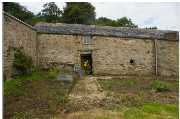
Figure 18: Section 1's east elevation; from the east.
