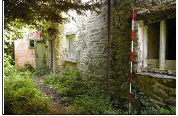
Figure 41: View along the west elevation of Section 4; from the south-west.
