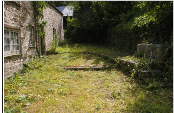
Figure 153: The south end of the yards; from the north.
