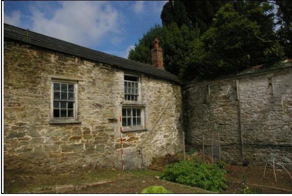
Figure 29: The north-east corner of the building, where it abuts the earlier wall of the former glass house or peach house; from the south-east.
