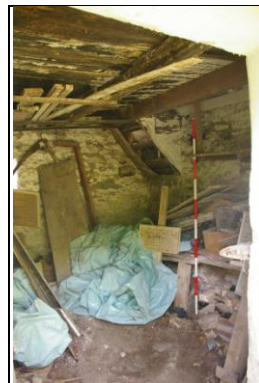
Figure 116: View into Room D, in Section 2; from the west, north-west.
