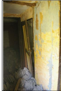
Figure 59: The door to the understair cupboard in Section 3; from the south-west.
