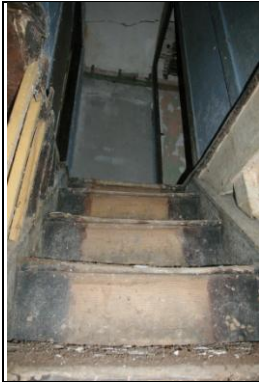
Figure 62: View up the stairs in Section 3; from the east.
