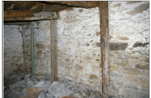
Figure 99: View down the east wall of the animal house, Room L; from the south-west.
