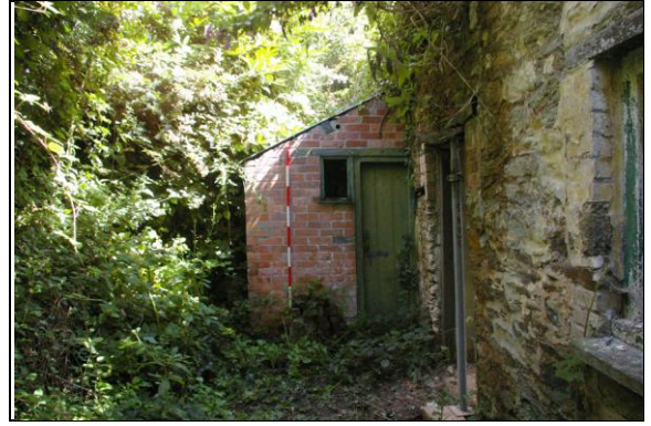
Figure 33: The brick built privy which abuts the west elevation of Section 4; from the south.
