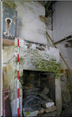
Figure 127: The chimney stack in Room E, Section 2; from the west, north-west.
