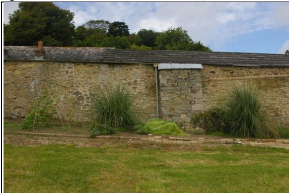
Figure 23: The east elevation of Section 3; from the east.
