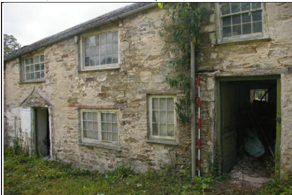
Figure 47: View along the west elevation of Section 2; from the south-west.
