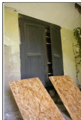
Figure 84: The cupboard in Room M, Section 4; from the east south east.
