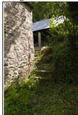
Figure 155: The dressed granite block steps which rise around the south-west corner of the building, giving access to the back drive; from the north-west.
