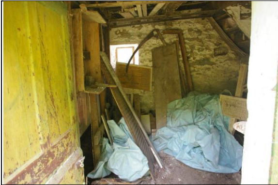
Figure 118: The east wall of Room D, Section 2; from the west.
