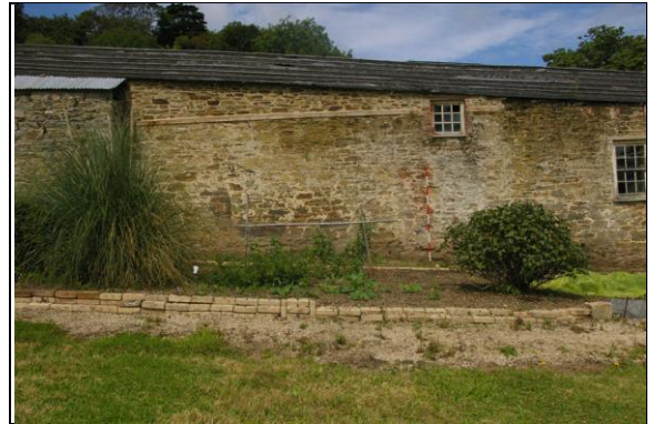
Figure 26: Northern part of the east elevation of Section 3; from the east.
