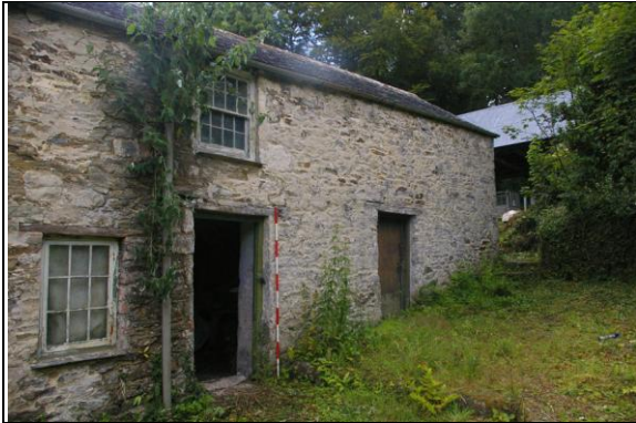
Figure 54: View of the south end of the west elevation of the building; from the north-west.
