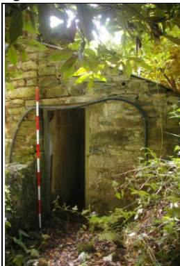
Figure 31: View of the small stone-built privy which abuts the west wall of Section 4, serving the sunken gardeners walkway; from the north.
