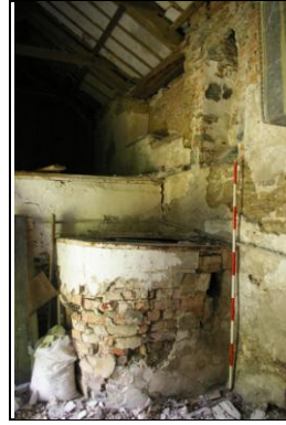
Figure 129: The copper inserted into Section 2, Room E; from the south, south-west.
