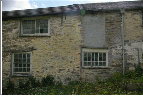
Figure 45: The west elevation between Section 2 and Section 3; from the west.
