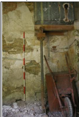
Figure 128: View of the water tank in Room E, Section 2; from the west.
