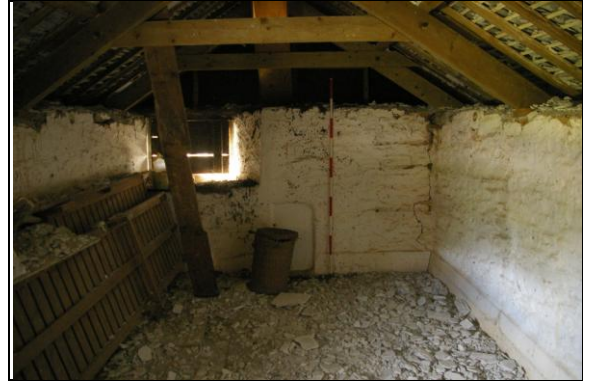
Figure 105: View of the south elevation of Room B, in Section 1, with fireplace built into the width of the wall; from the north.
