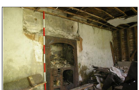
Figure 148: The east wall of Room G, in Section 3, with the cast-iron grate; from the north-west.
