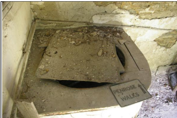
Figure 135: The top of the copper in Section 2; from the west.
