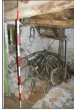
Figure 97: View of where the stairway from Room M is forced through the wall Room L; from the south-east.
