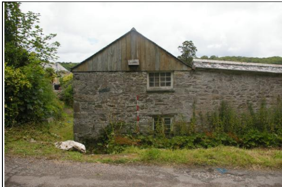
Figure 15: View of the south elevation; from the south.
