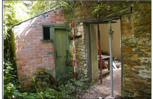
Figure 34: The doorway to Room M in Section 4; from the south-west.
