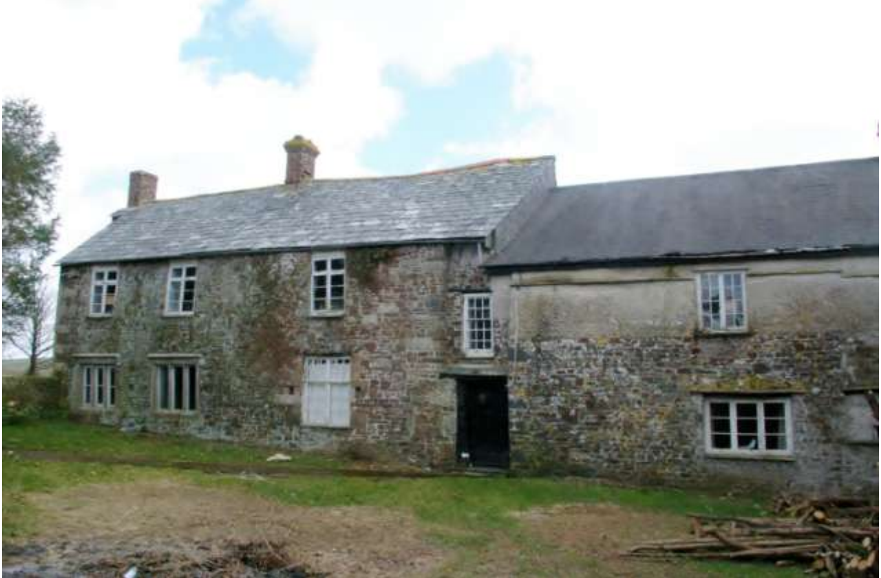
The north elevation; from the north west.
