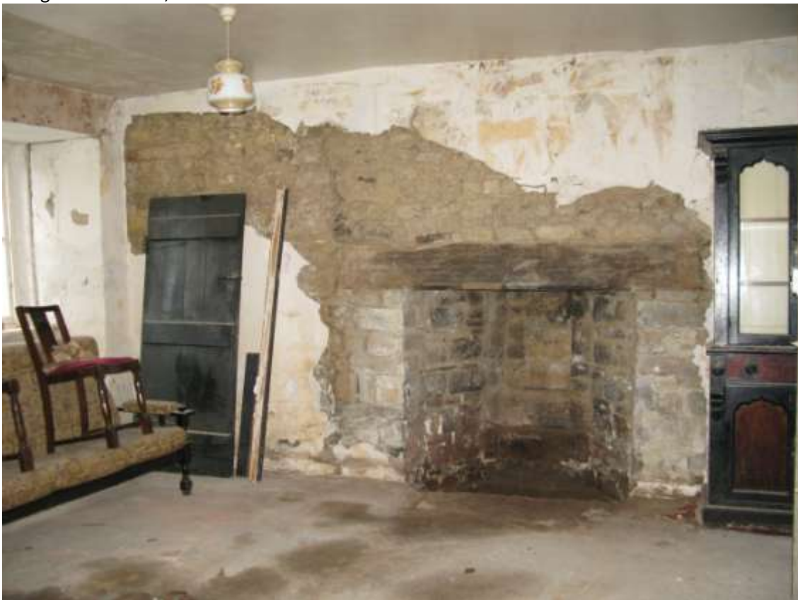
The 17 th century fireplace in the eastern ground floor room; from the south west.
