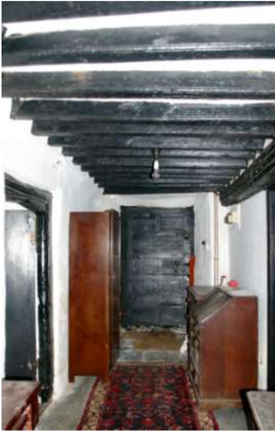
The cross passage; from the south.
