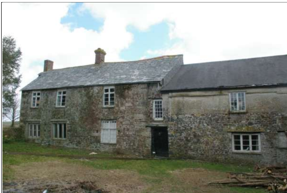
Figure 9: Shot of the north elevation, viewed from the north-east.
