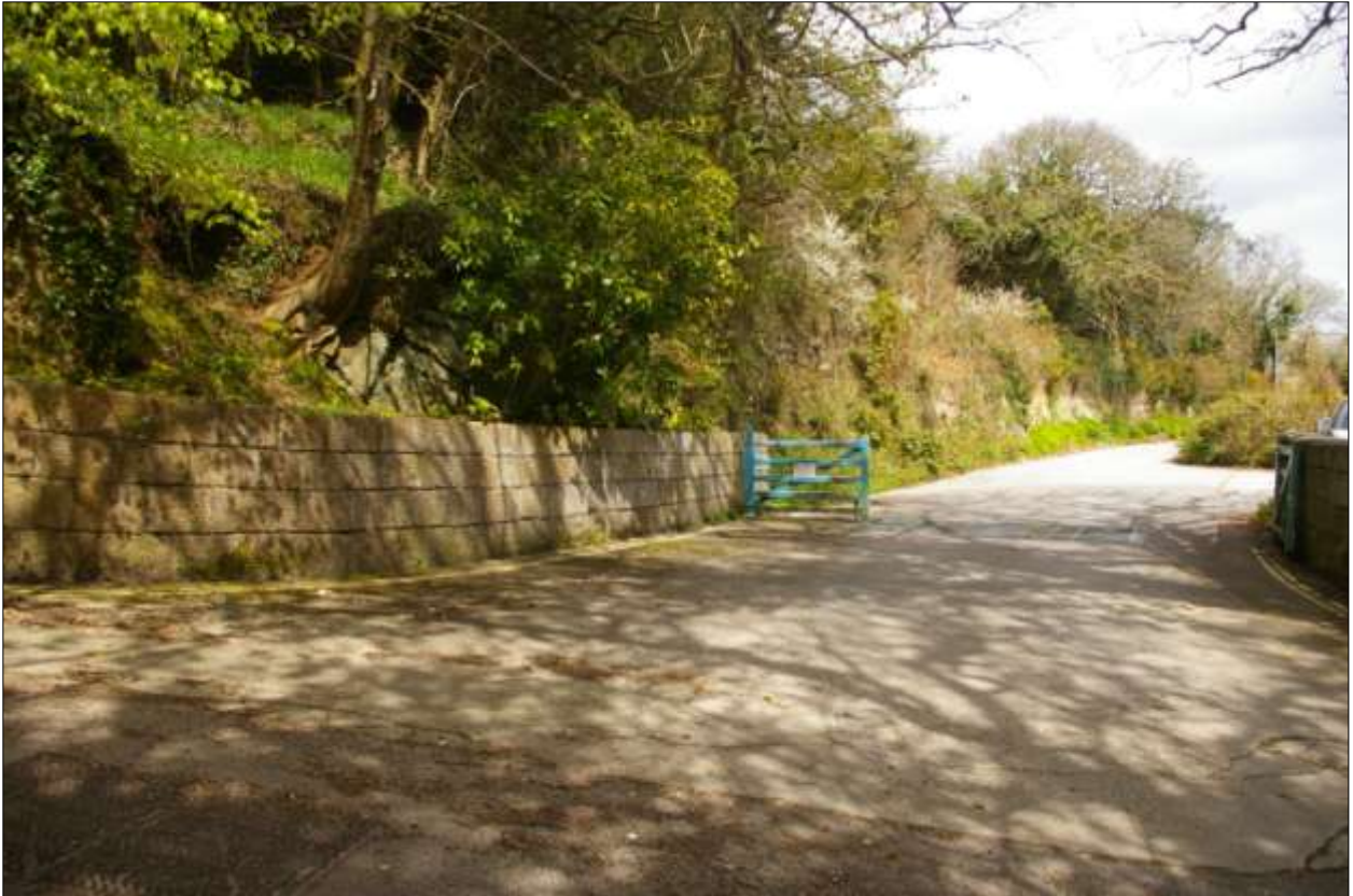
The entrance to the site, off Packsaddle Hill, showing the wide splayed opening and concrete road; from the west.
