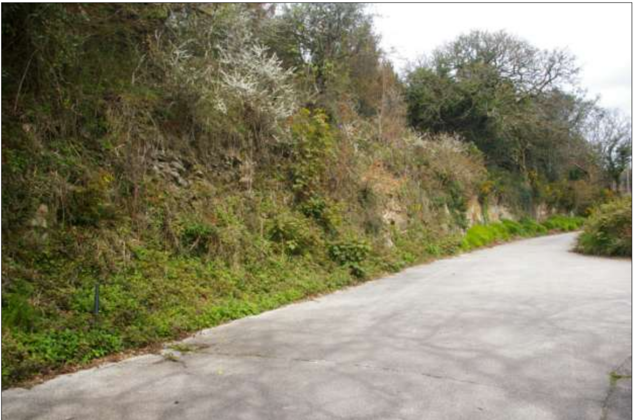
The northern boundary of the site, showing how the upper northern half of the site has been steeply terraced into the slope to make a driveway to the houses to the east; from the west-south-west.
