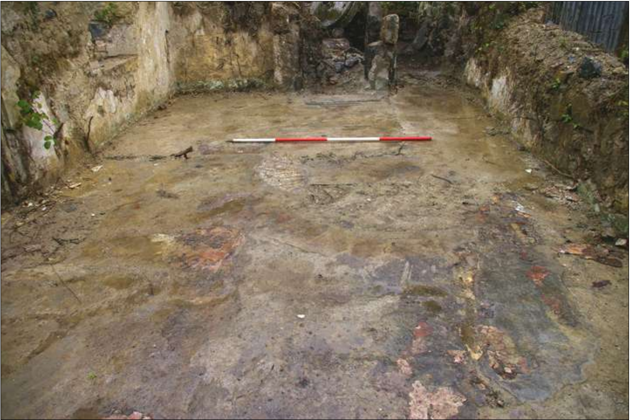
General view of the concrete floor of the cottage; viewed from the north (scale 2m).
