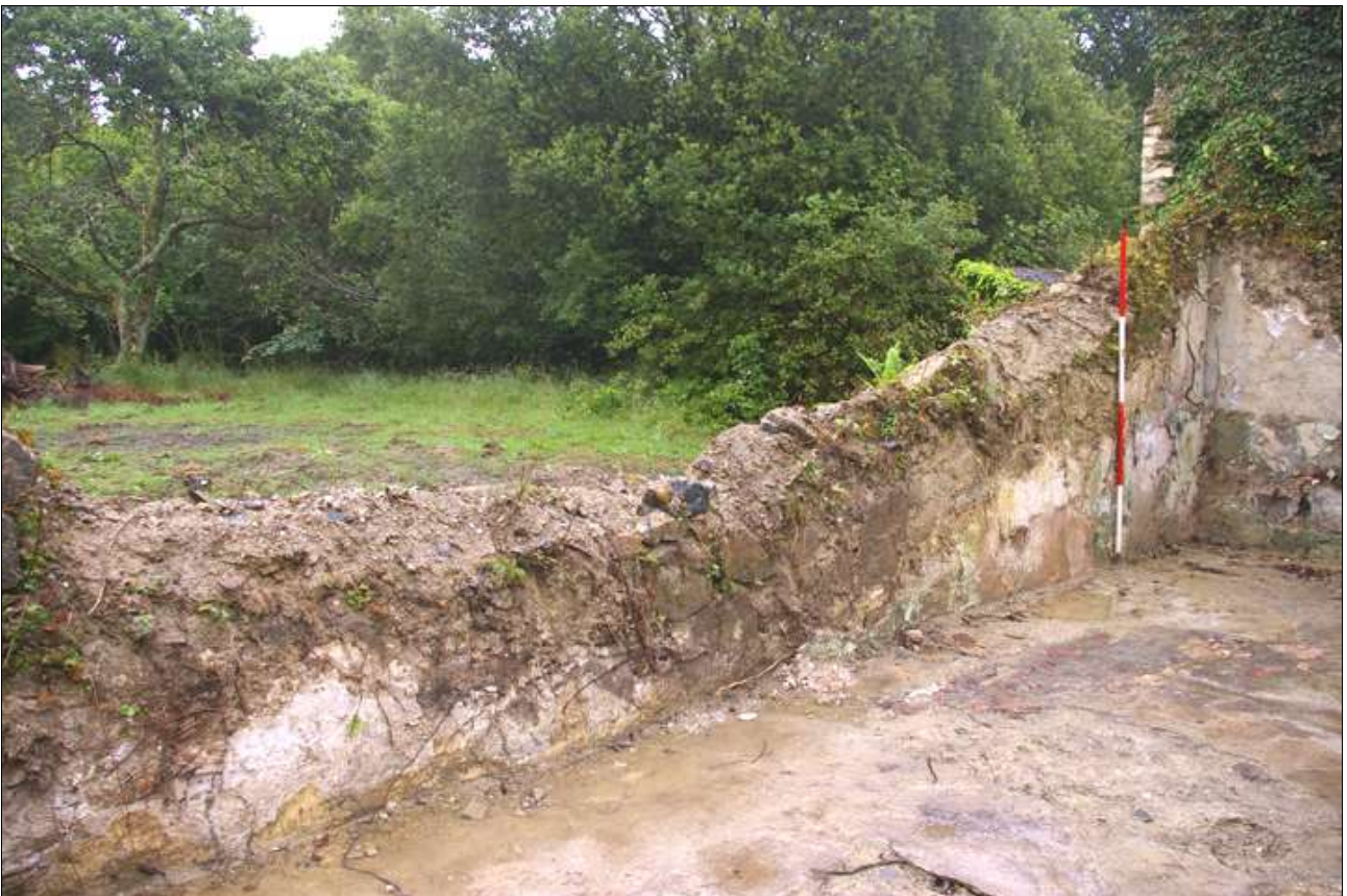
The internal elevation of the east wall of the cottage; viewed from the north-west (scale 2m).
