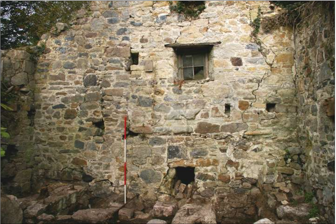
The interior of the north wall of the mill after the machinery was removed; viewed from the south-east (scale 2m).
