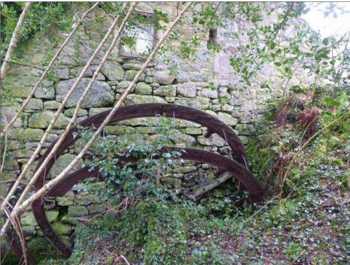
North gable of the Mill, with wheelpit and waterwheel (photo: M Watts).
