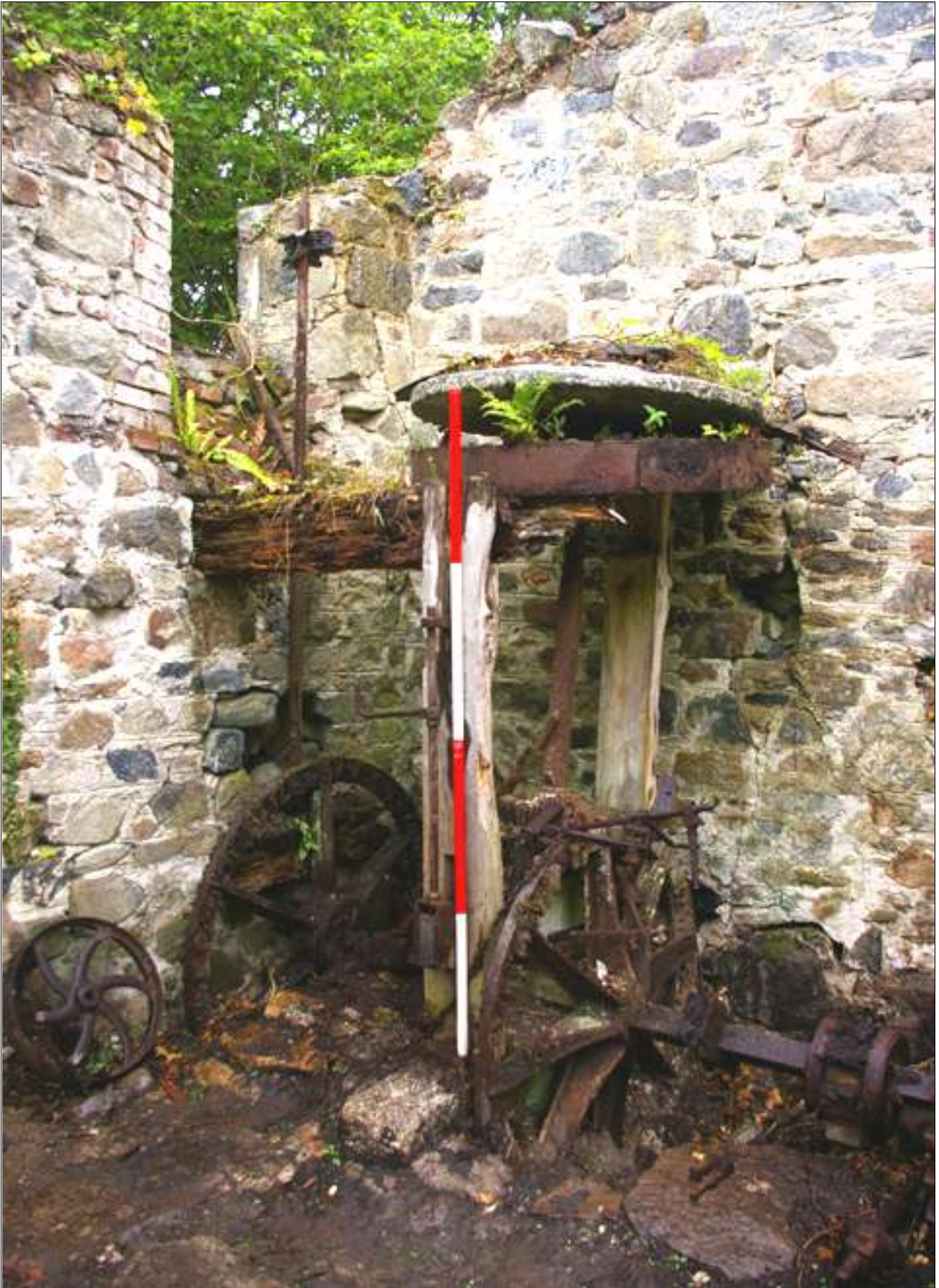
The upstream layshaft, driving gears and millstones; viewed from the south-east (scale 2m).
