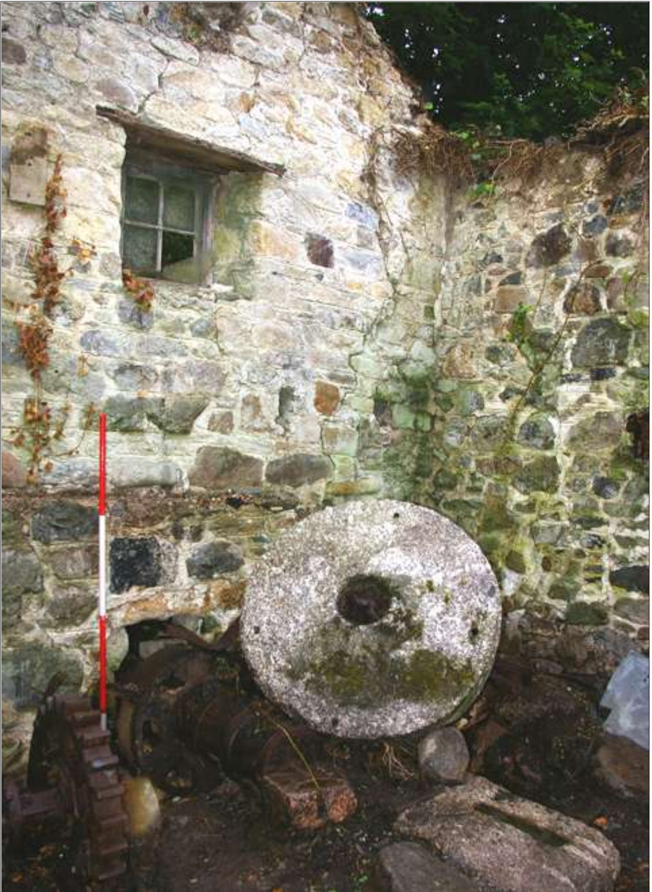
The downstream layshaft and millstones; viewed from the south-west (scale 2m).
