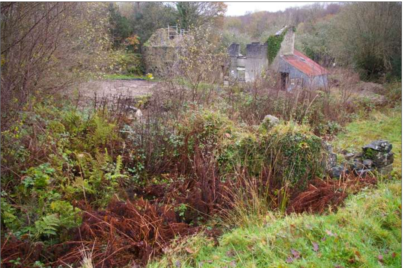
Looking across the collapsed building south-west of the mill and cottage; viewed from the south-west.
