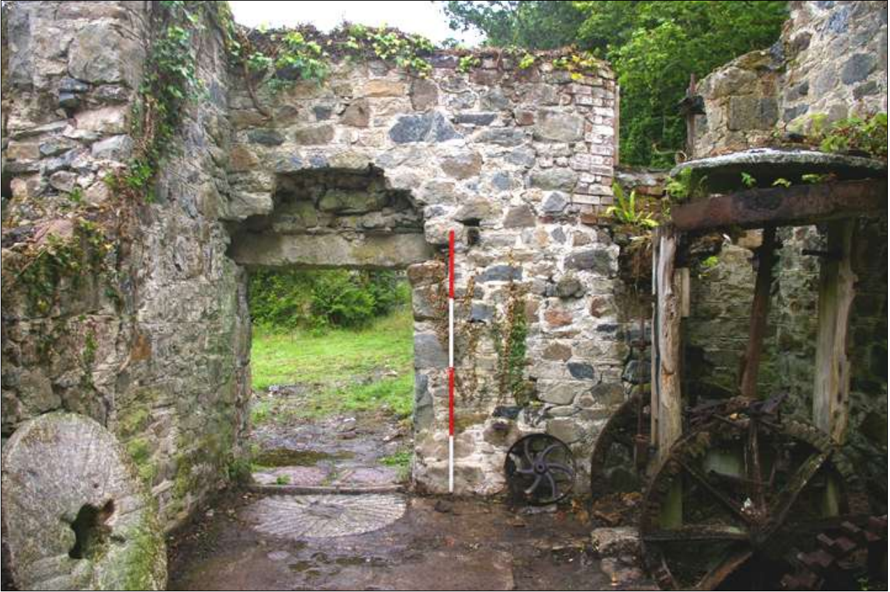
The internal elevation of the west wall of the mill; viewed from the east (scale 2m).
