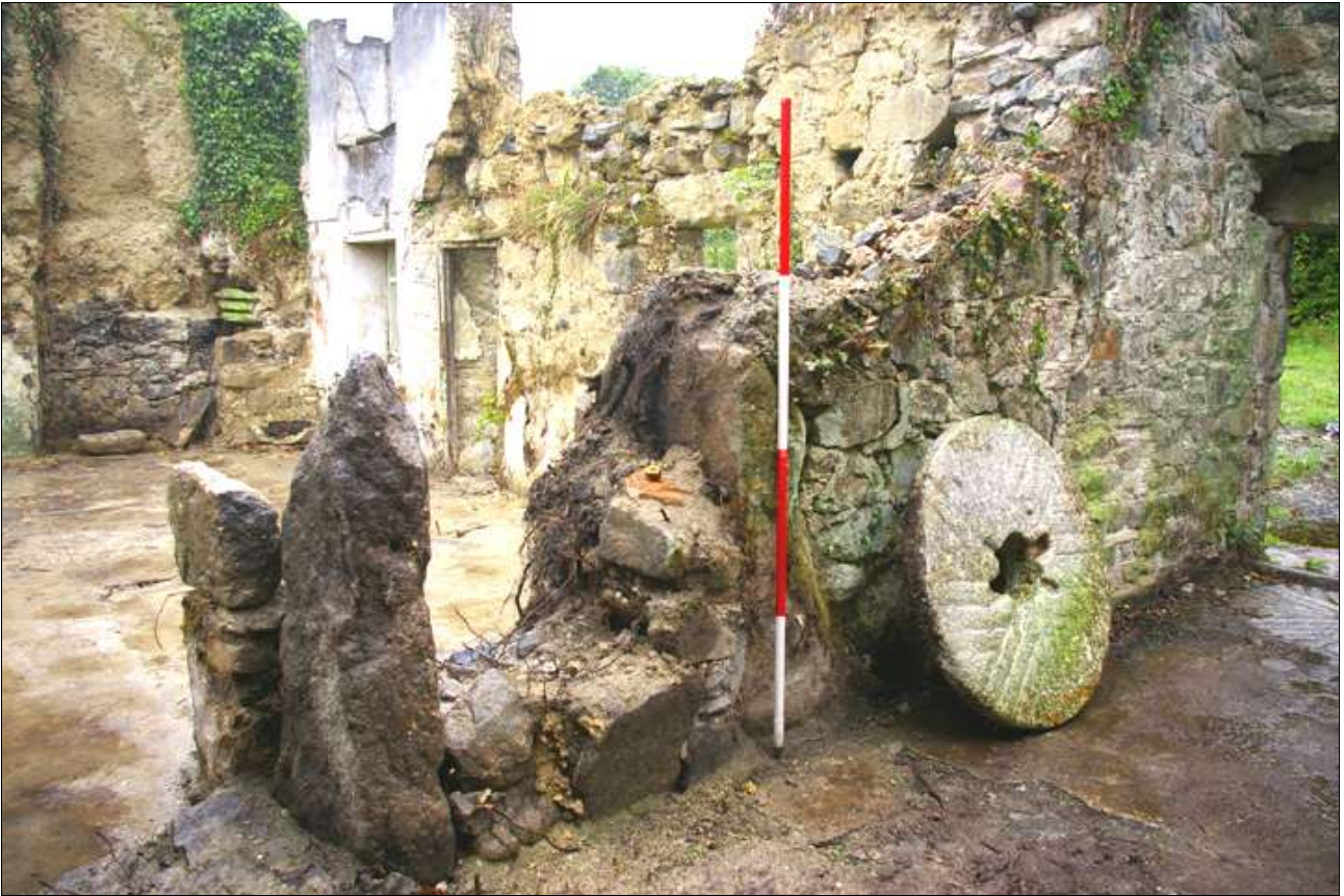
The south wall of the mill, showing the blocked orthostat doorway; viewed from the north-east (scale 2m).
