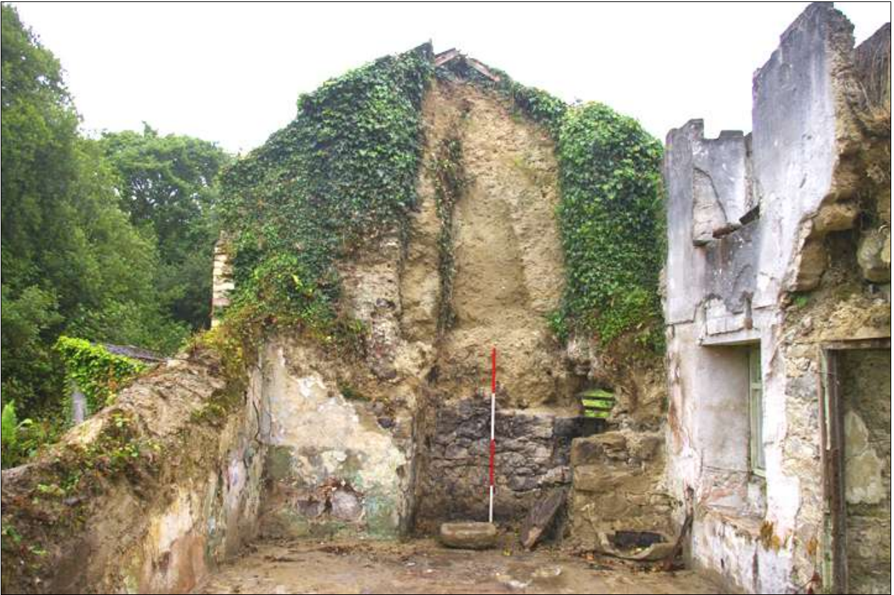
The interior of the cottage, showing the southern gable stack and flue; viewed from the north (scale 2m).
