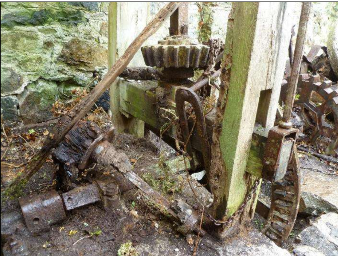
Bridge posts and drive to upstream millstones (photo: M Watts).
