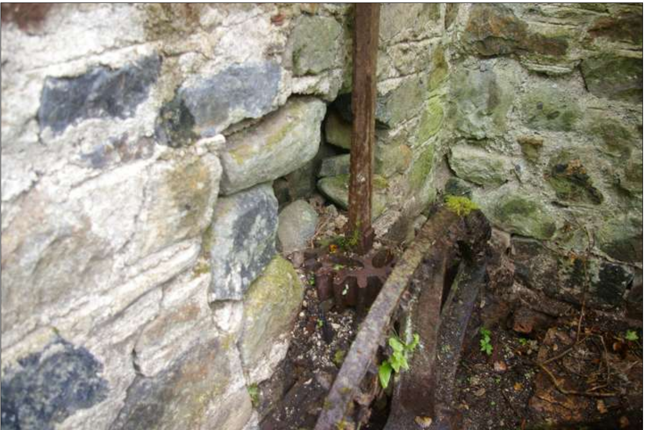
Detail of the point where the layshaft breaches the west wall of the Mill; viewed from the south-east.
