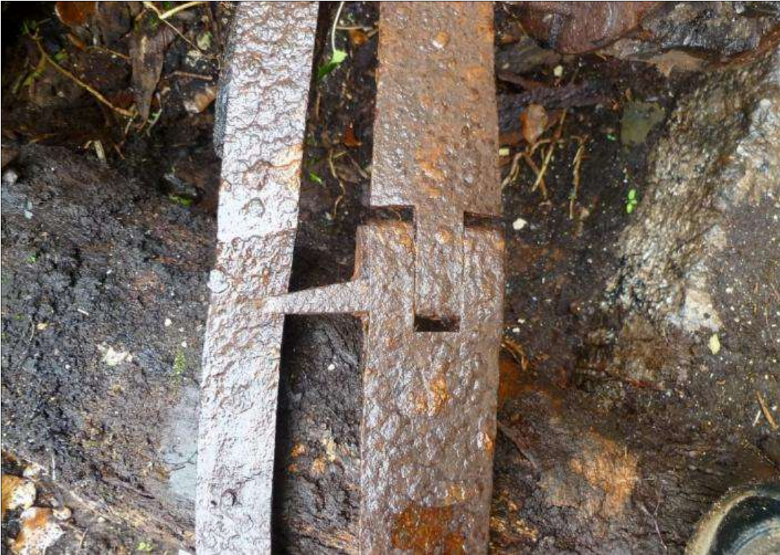
Detail of forged connection to iron band with wedge to tighten it around circumference of stone drive gear (photo: M Watts).
