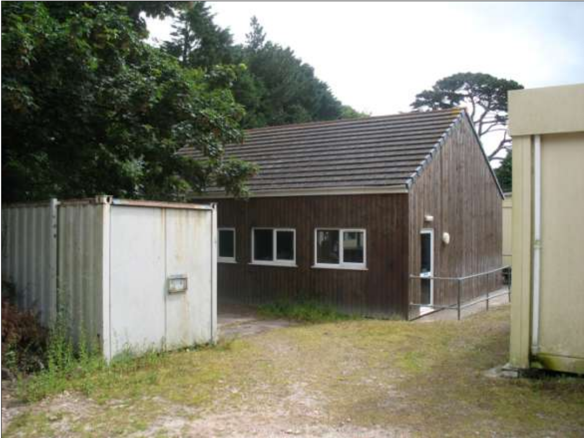
TEMPORARY CLASSROOM #4; VIEWED FROM THE SOUTH-WEST. THIS STRUCTURE WOULD BE RETAINED.
