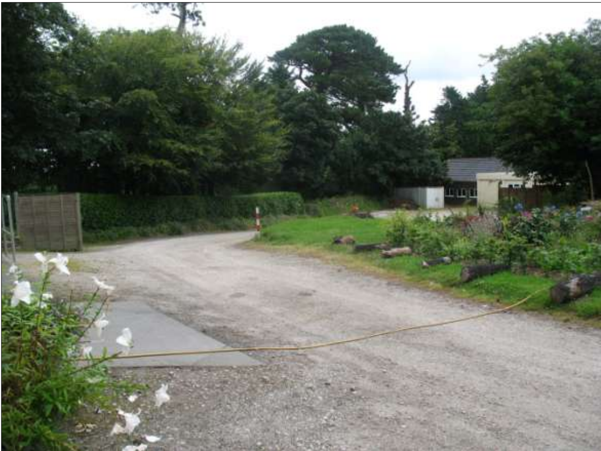
THE ENTRANCE TO THE NEW CAR PARK; VIEWED FROM THE SOUTH.
