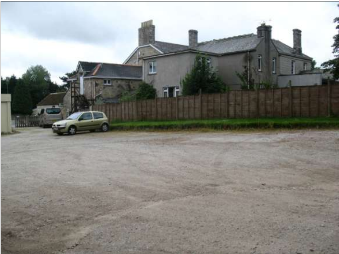
THE MAIN HOUSE, AS VIEWED FROM ACROSS THE NEW CAR PARK; VIEWED FROM THE NORTH-WEST.
