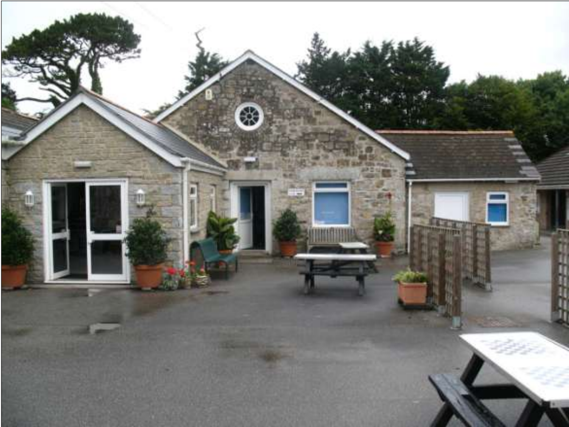
AS ABOVE, VIEWED FROM THE SOUTH.
