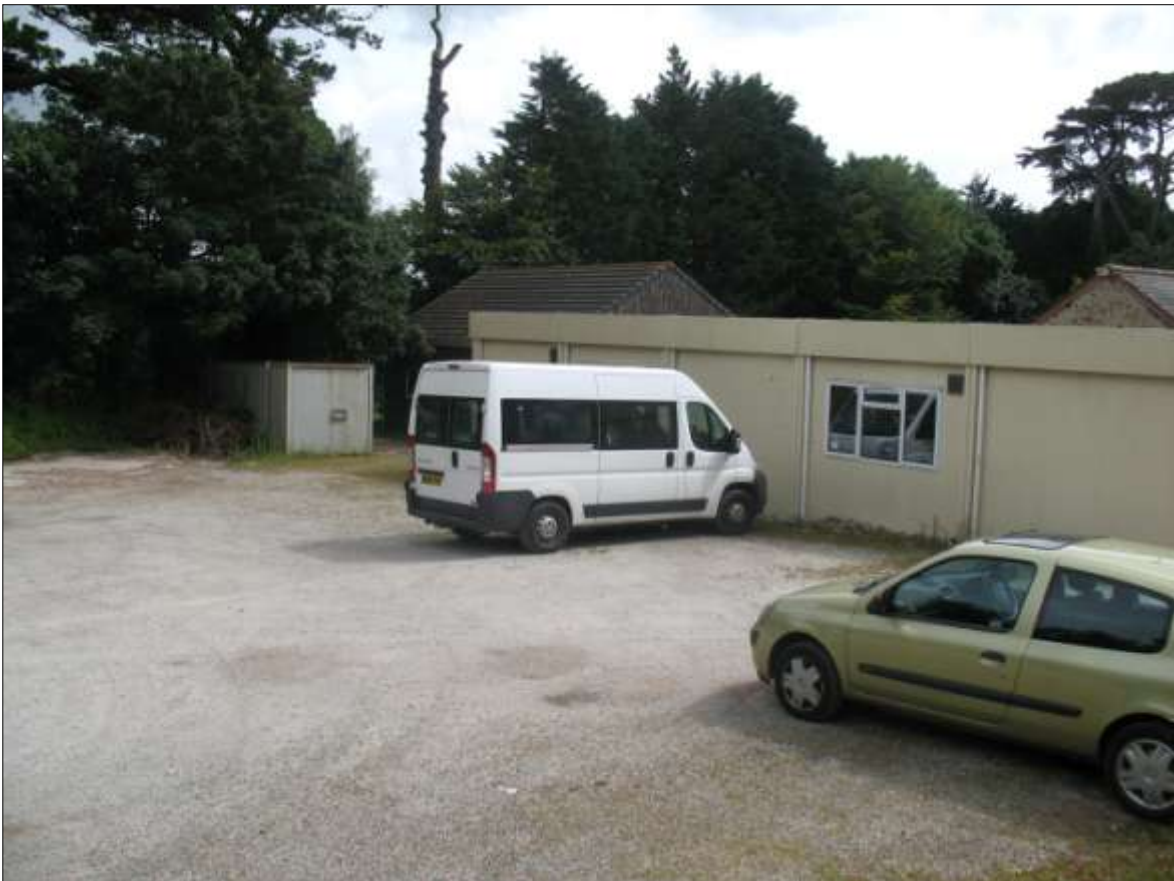
TEMPORARY CLASSROOM #5; VIEWED FROM THE SOUTH-WEST.
