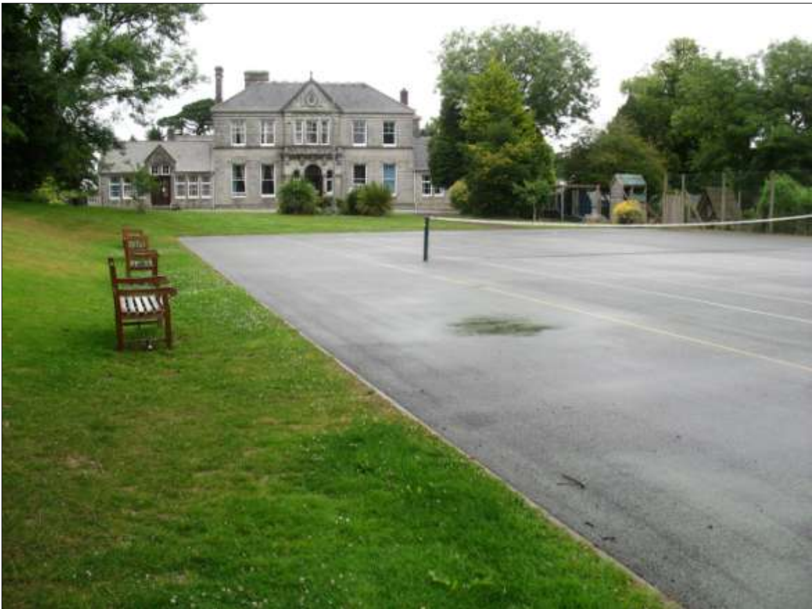
THE SOUTH ELEVATION, VIEWED FROM ACROSS THE TENNIS COURT TO THE SOUTH.
