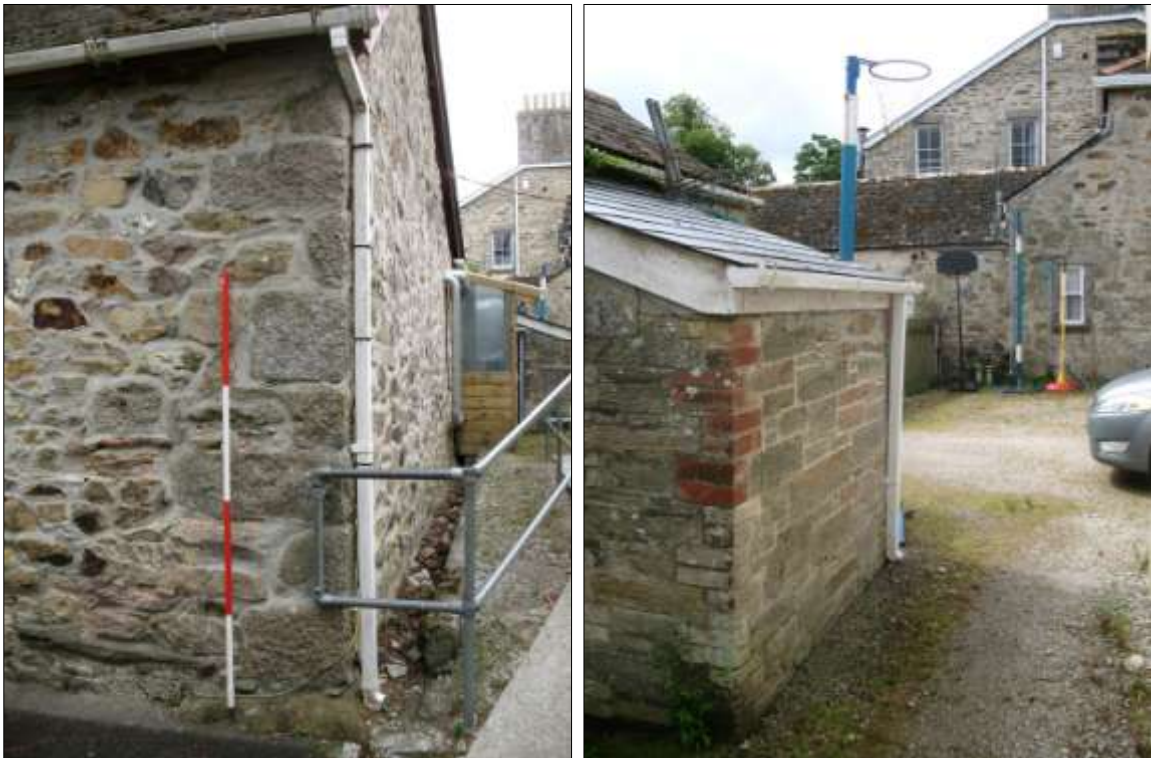
LEFT: QUOINS TO NORTH-WEST CORNER OF THE OUTBUILDINGS (SCALE 2M).
