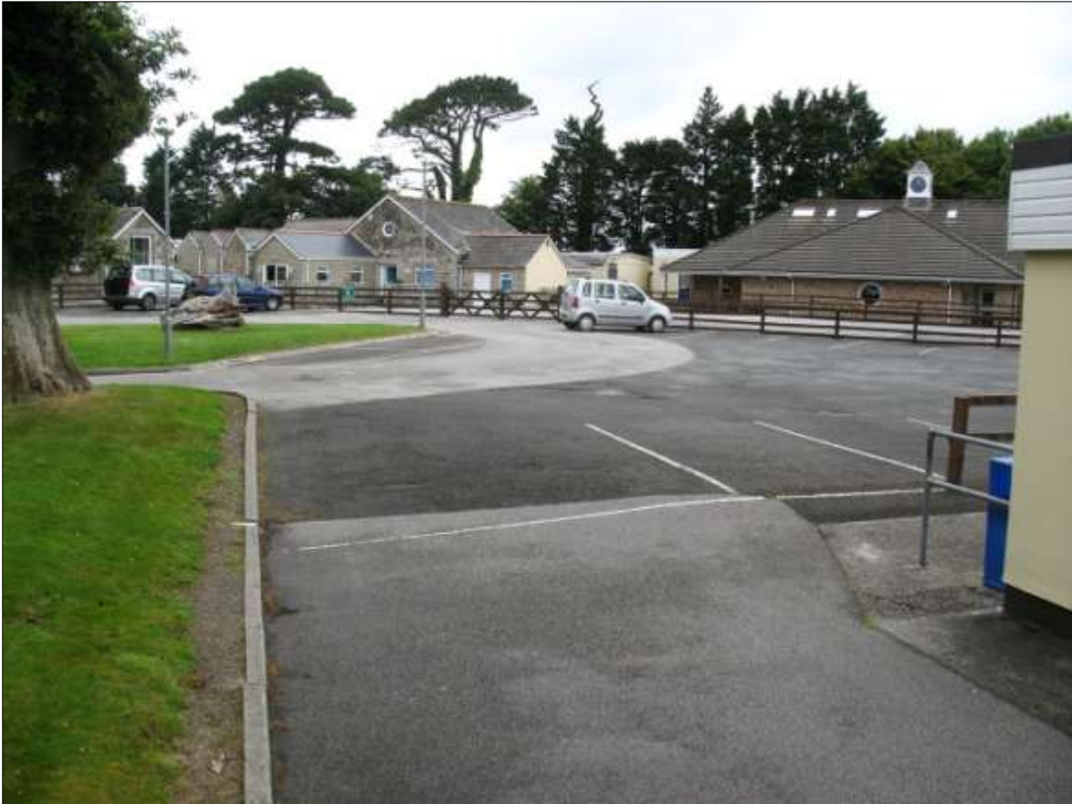
VIEW ACROSS THE EASTERN CAR PARK FROM THE SOUTH-EAST, SHOWING THE 1870S OUTBUILDINGS (LEFT).
