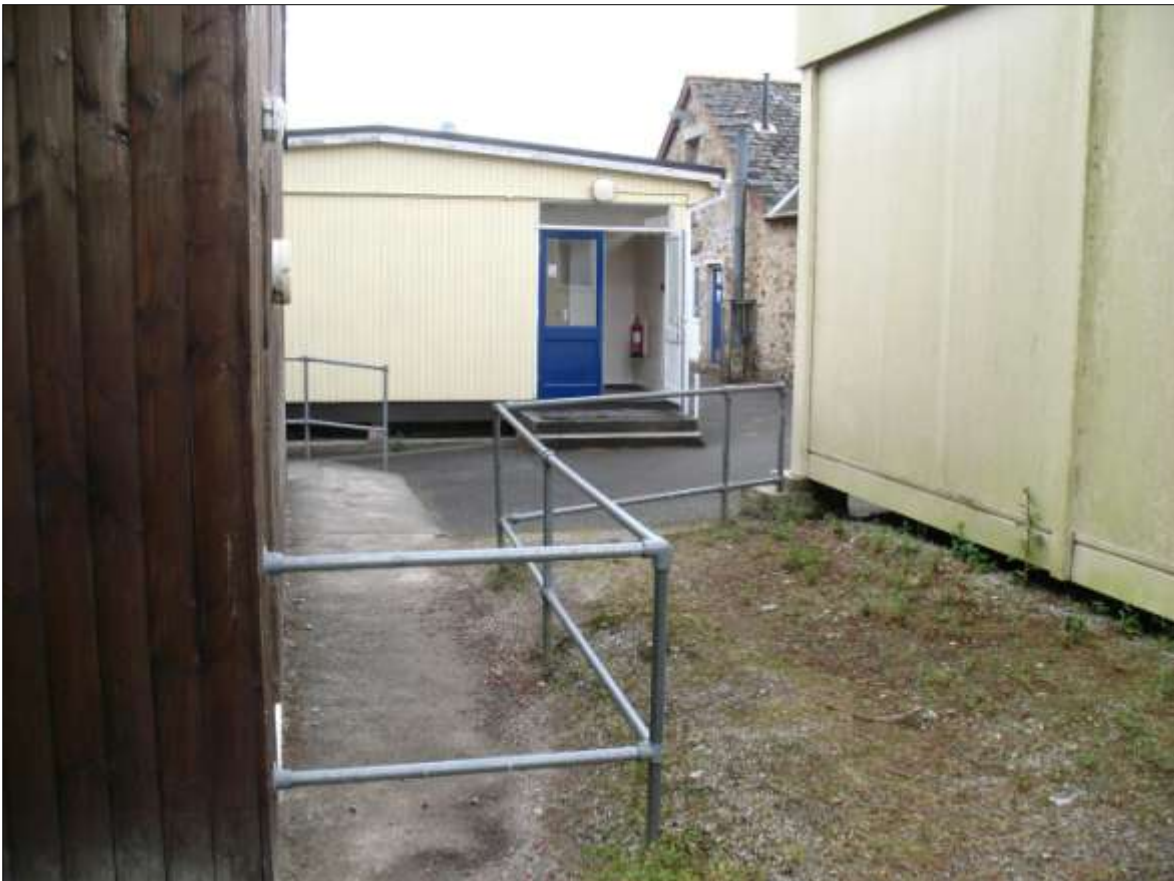
TEMPORARY CLASSROOM #3; VIEWED FROM THE WEST BETWEEN TC#4 AND TC#5.
