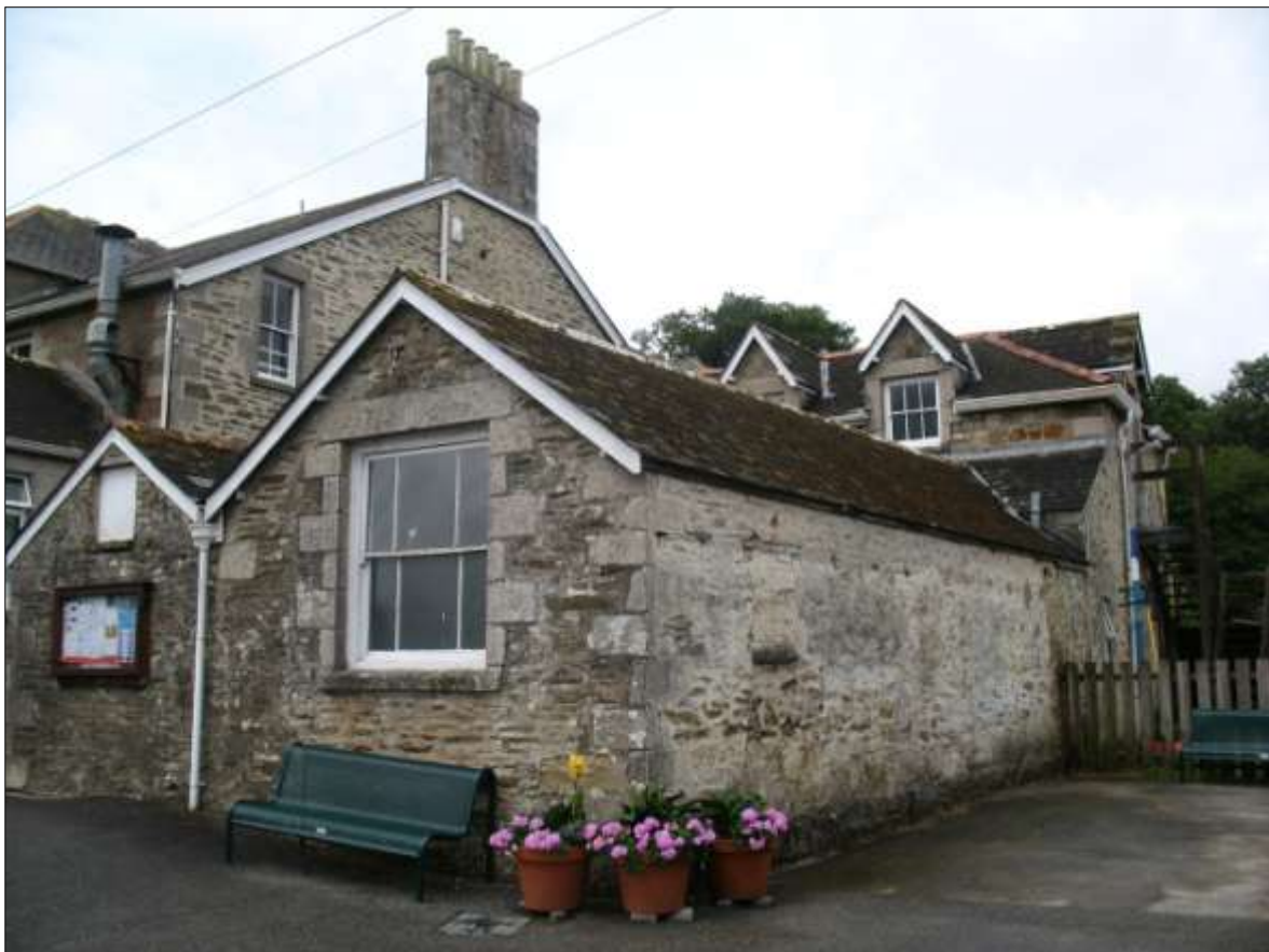
THE SINGLE-STOREY SECTION OF THE BACKBLOCK; VIEWED FROM THE NORTH-EAST.
