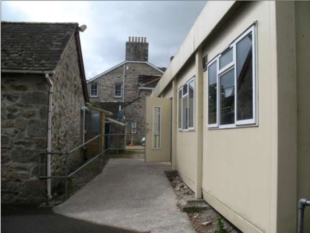
TEMPORARY CLASSROOM #5; VIEWED FROM THE NORTH.
