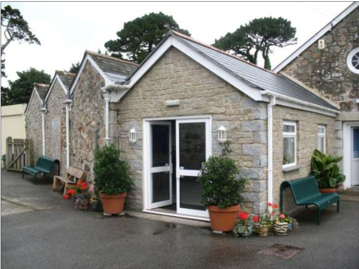
THE SOUTH ELEVATION OF THE OUTBUILDINGS; VIEWED FROM THE SOUTH-EAST.
