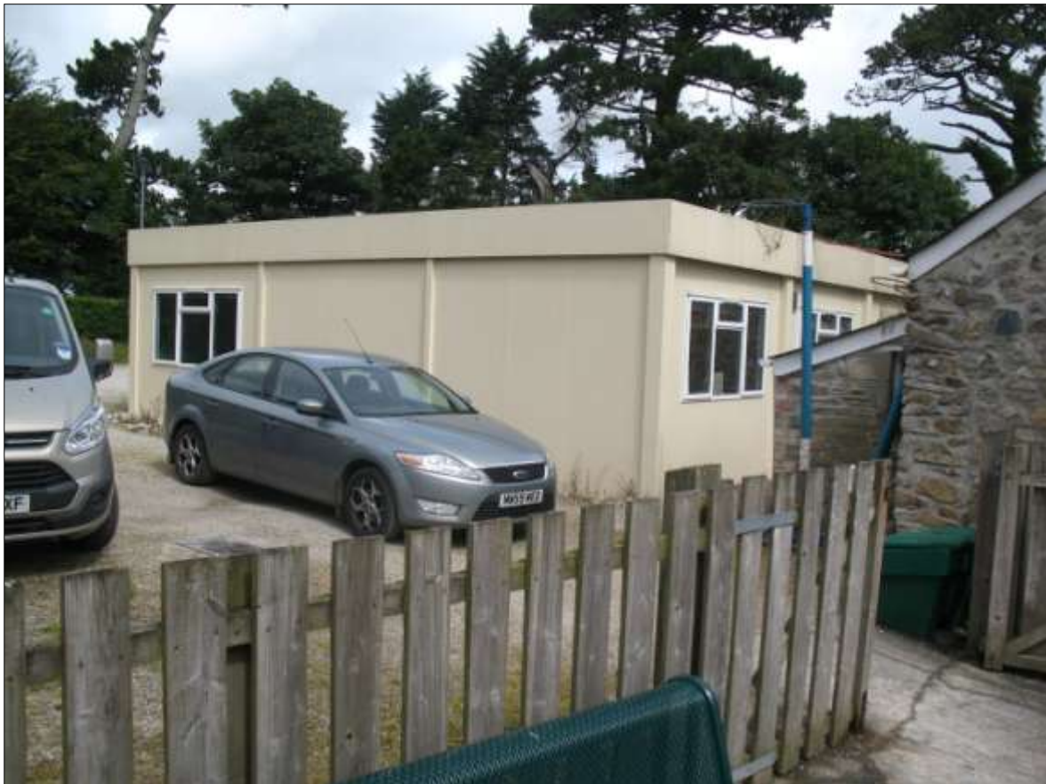
TEMPORARY CLASSROOM #5 (TC#5); VIEWED FROM THE SOUTH-EAST.
