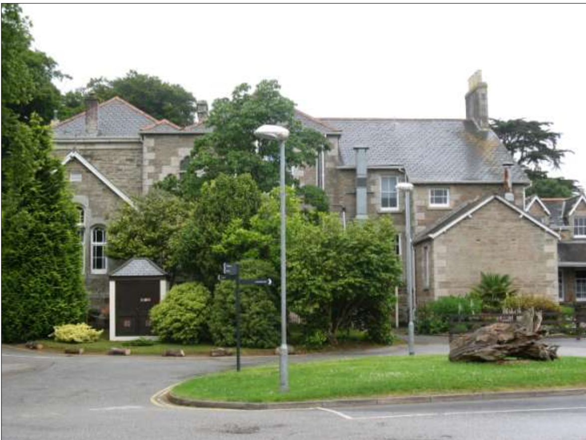
THE EAST ELEVATION OF THE MAIN HOUSE; VIEWED FROM THE EAST. NOTE THE USED OF STONE RUBBLE.
