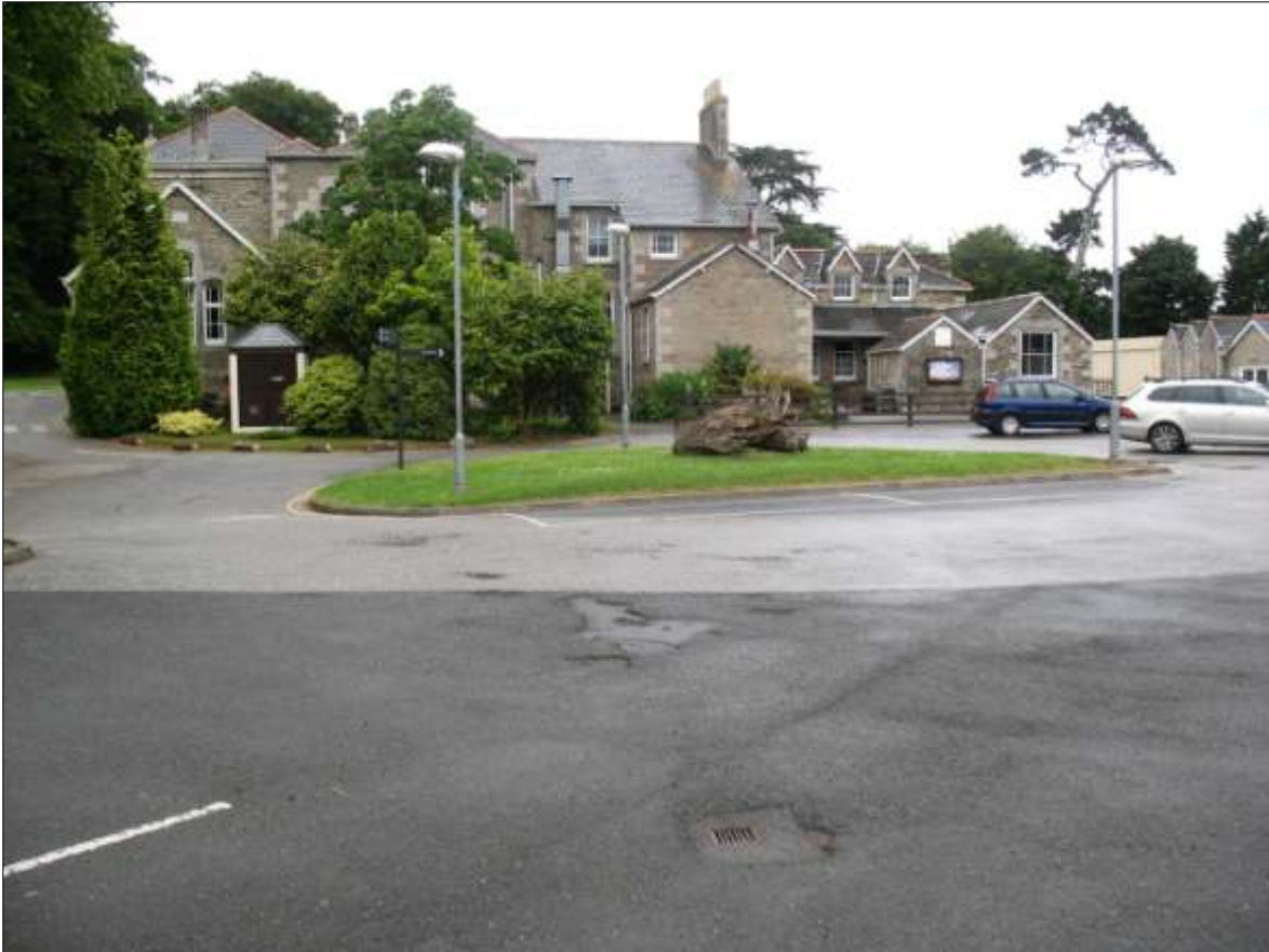
THE EAST ELEVATION OF THE HOUSE, WITH THE EAST CAR PARK IN THE FOREGROUND; VIEWED FROM THE EAST.
