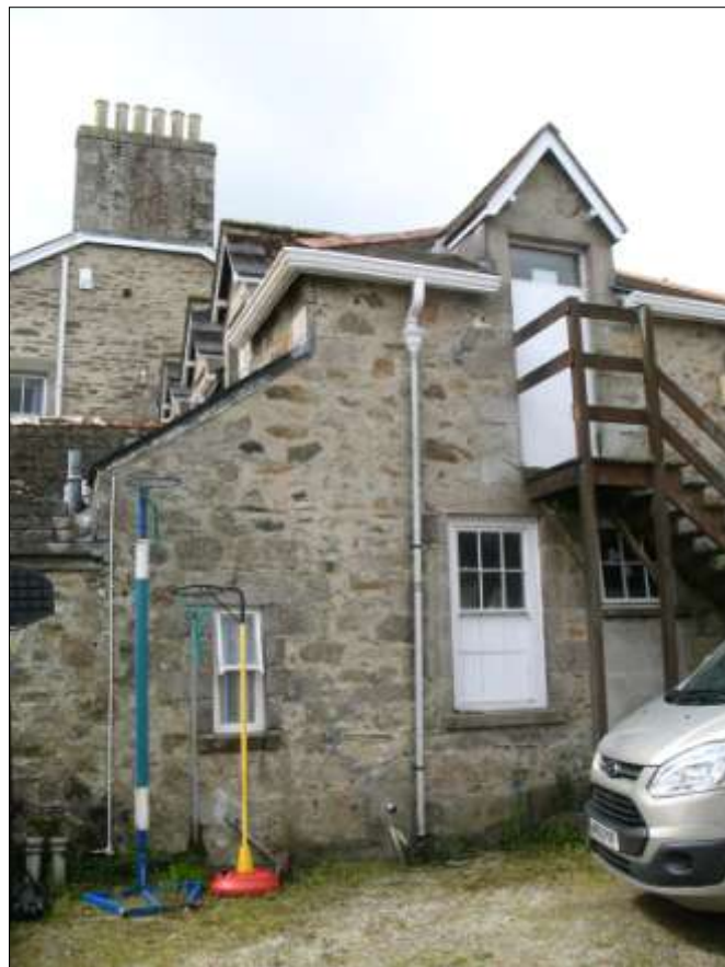
THE TWO-STOREY SECTION OF BACKBLOCK; VIEWED FROM THE NORTH.
