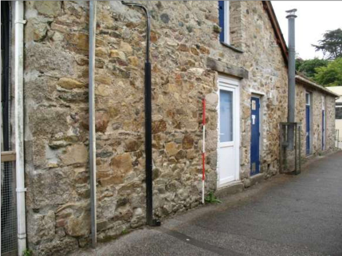
THE NORTH ELEVATION; VIEWED FROM THE NORTH-EAST (SCALE 2M).
