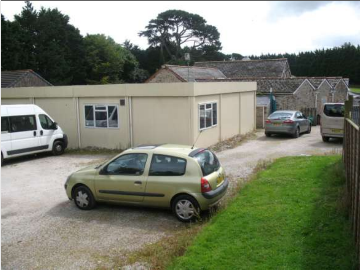
TEMPORARY CLASSROOM #5; VIEWED FROM THE SOUTH-WEST.
