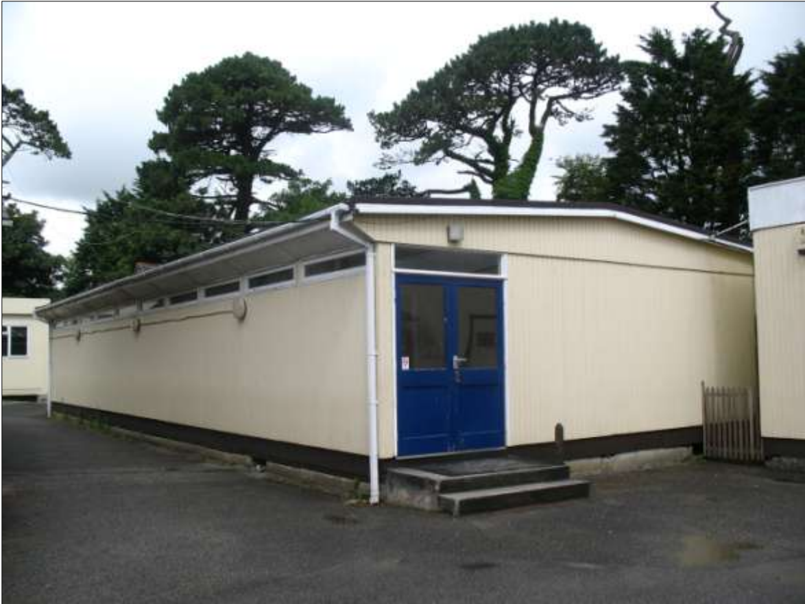
TEMPORARY CLASSROOM #3; VIEWED FROM THE SOUTH-EAST.
