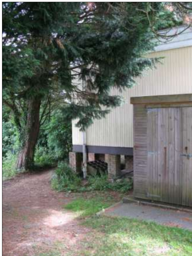
THE NORTH END OF TEMPORARY CLASSROOM #1; VIEWED FROM THE WEST.
