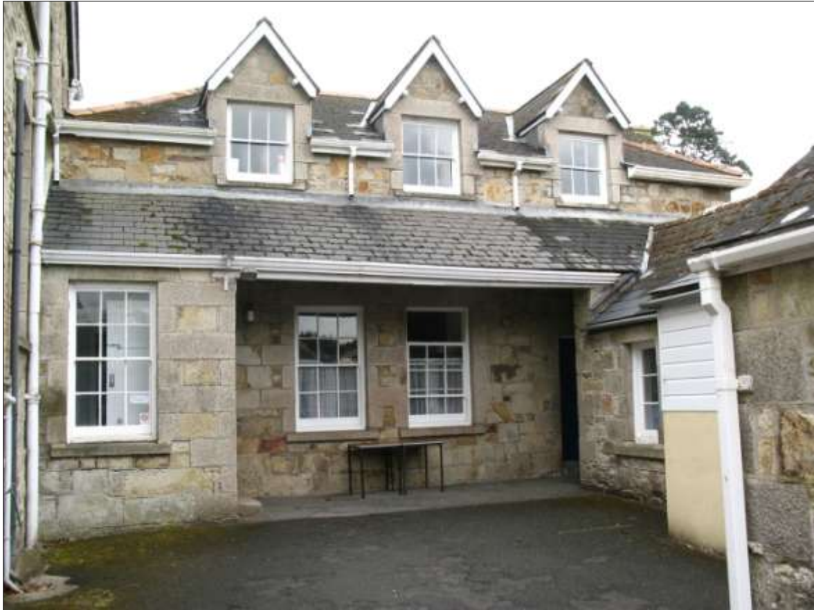
THE TWO-STOREY SECTION OF BACKBLOCK; VIEWED FROM THE EAST.
