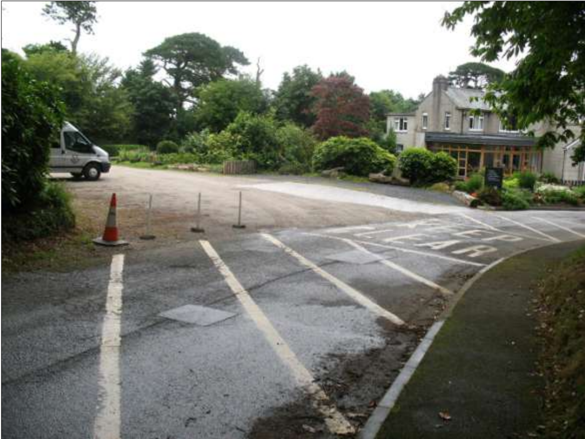
THE MAIN DRIVE SHOWING THE ENTRANCE TO THE NEW CAR PARK TO THE WEST; VIEWED FROM THE WEST.
