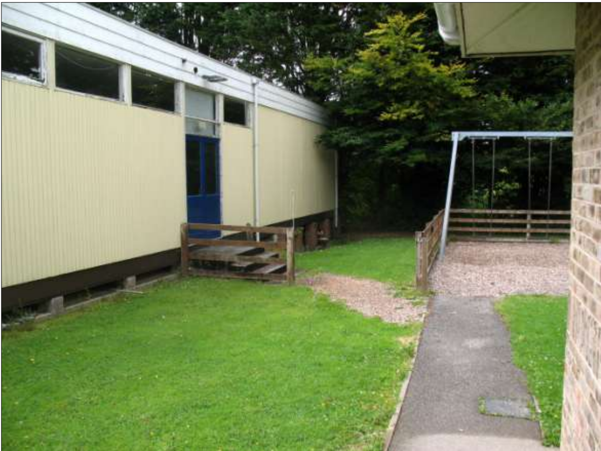
THE EAST ELEVATION OF TC#1; VIEWED FROM THE SOUTH.
