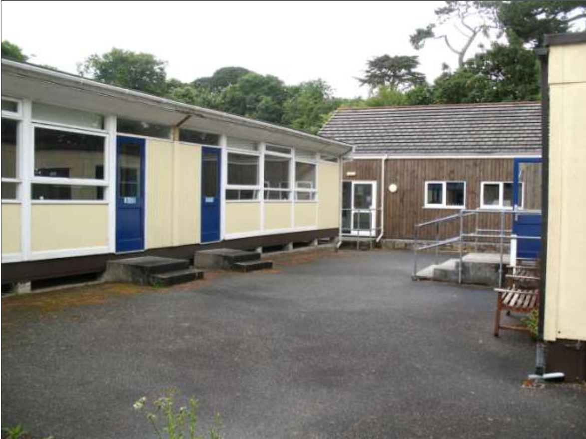
AS ABOVE, WITH TEMPORARY CLASSROOM #4 IN THE BACKGROUND; VIEWED FROM THE EAST.
