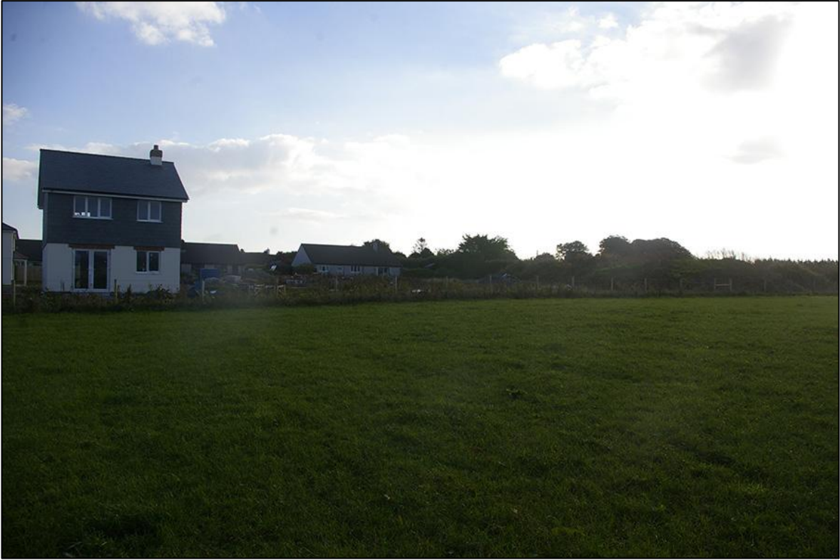
FIGURE 8: NORTH PART OF SITE WITH CURRENT AREA UNDER DEVELOPMENT; VIEWED FROM THE NORTH-WEST (NO SCALE).
