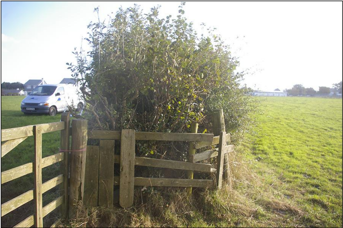
FIGURE 10: BOUNDARY DIVIDING THE SITE IN TO NORTHERN AND SOUTHERN FIELDS; VIEWED FROM THE WEST (NO SCALE).
