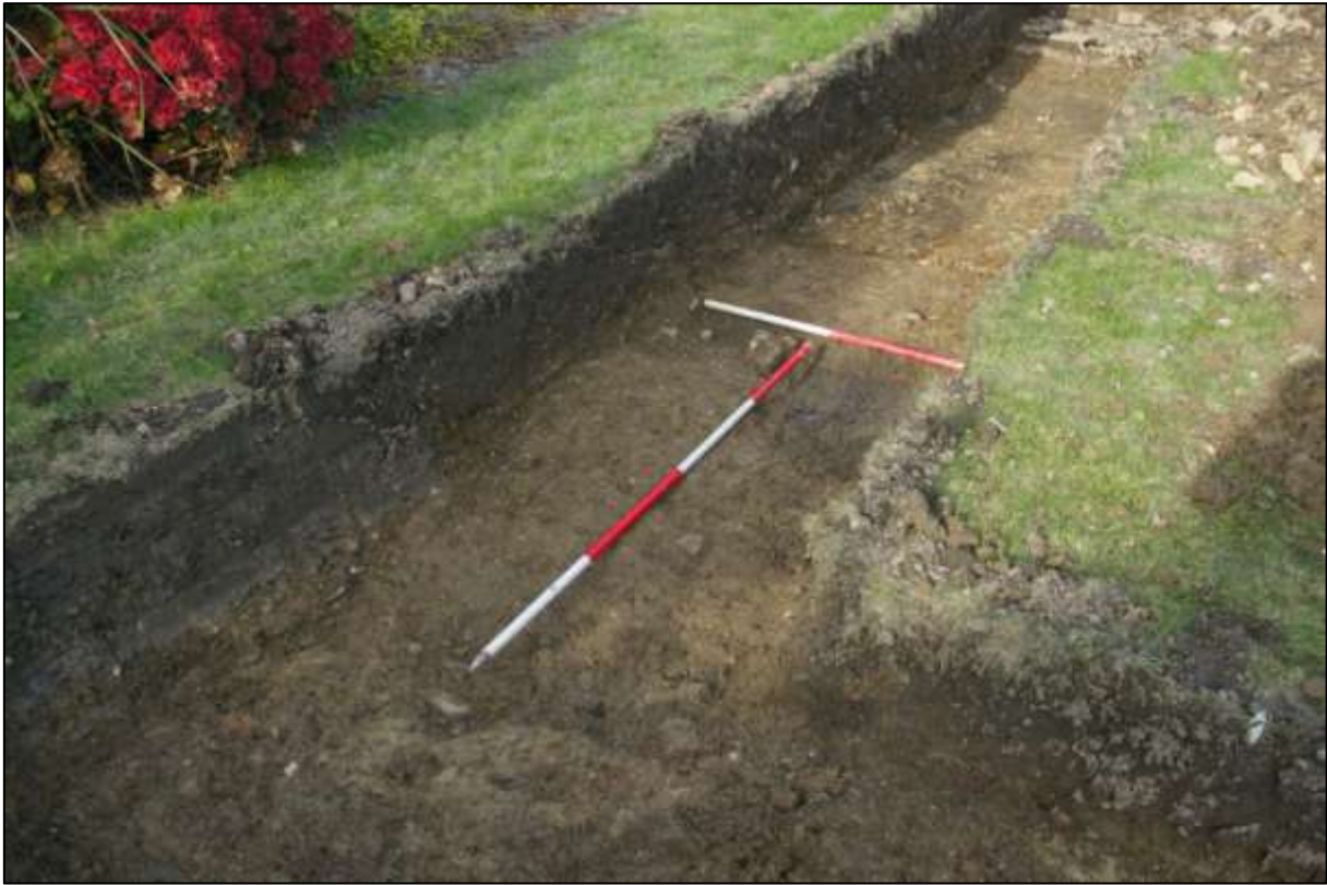
TRENCH 2, DRAINS [204] AND [206] PRE-EXCAVATION; VIEWED FROM THE SOUTH (1M & 2M SCALES).
