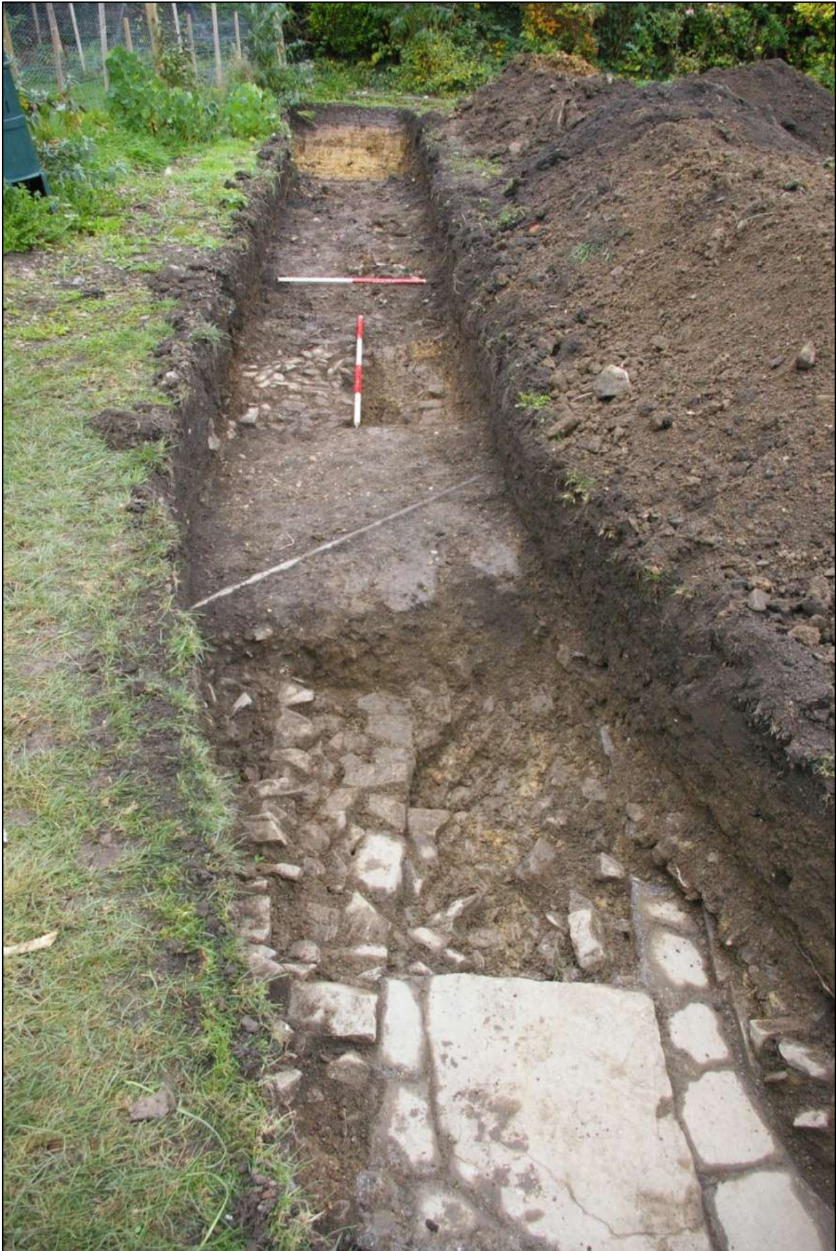
FIGURE 7: TRENCH 3 POST-EXCAVATION SHOWING WALL {314}, AND SLAB SURFACE (317) WITH COBBLE SURFACE (312) TOWARDS THE MIDDLE; VIEWED FROM THE NORTH-WEST (1M & 2M SCALES).
