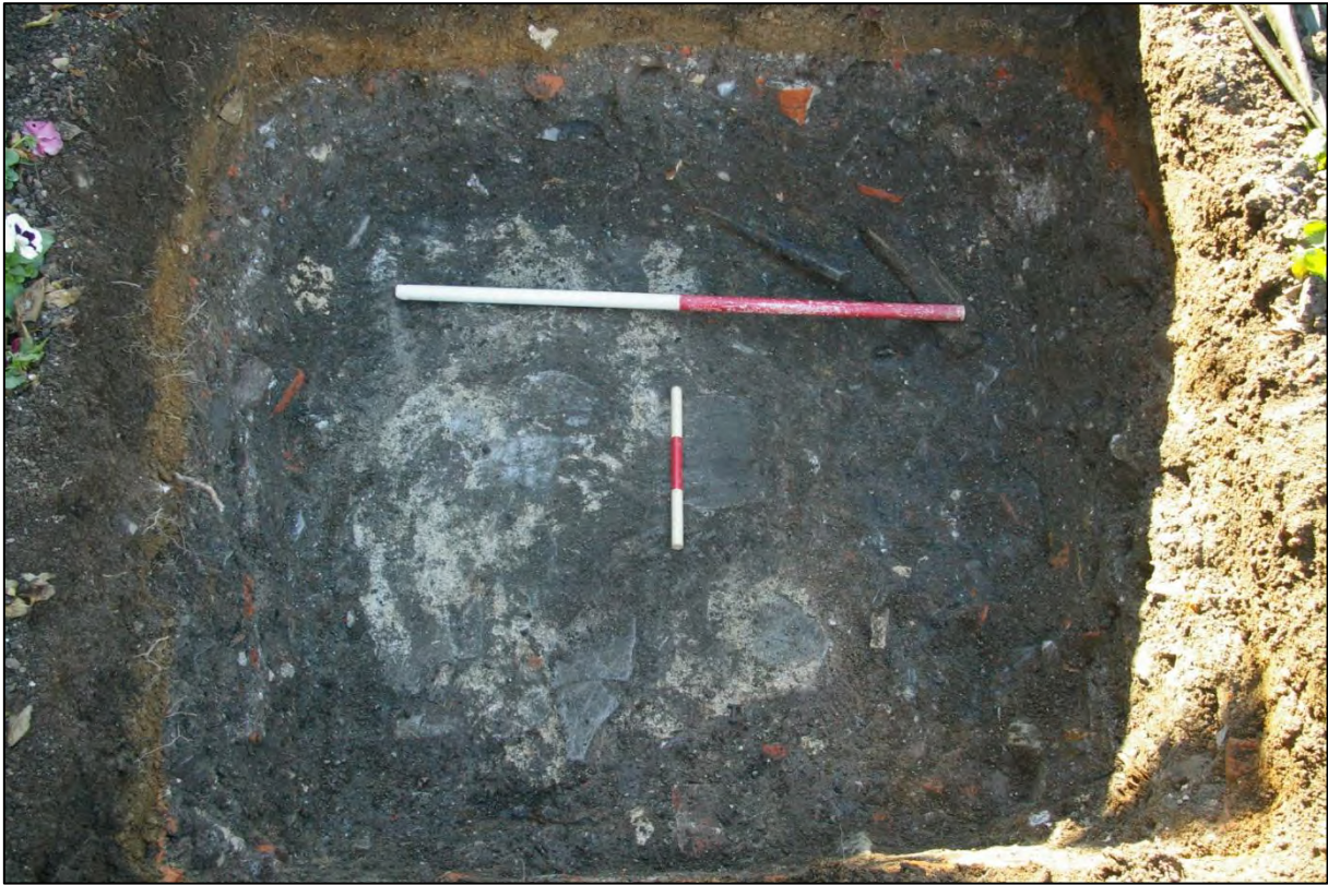
TEST PIT 2, WALL FOOTINGS {203} MID-EXCAVATION; VIEWED FROM THE NORTH-EAST (0.30M & 1M SCALES).
