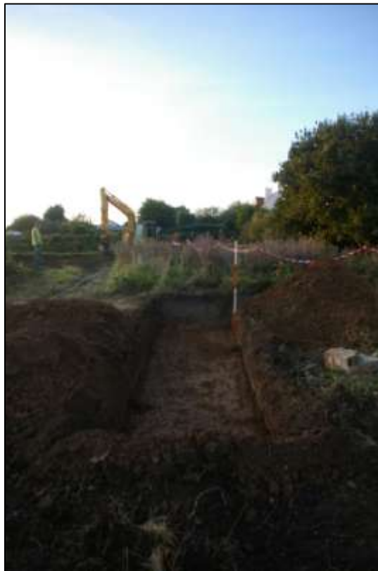
AREA 2, POST-EXCAVATION; VIEWED FROM THE SOUTH-EAST (2M SCALE).
