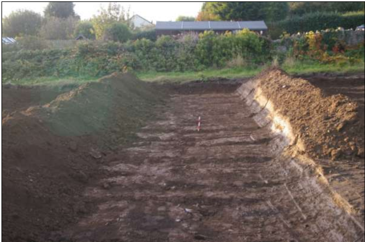
CULVERT [103]; VIEWED FROM THE SOUTH-EAST (2M SCALE).
