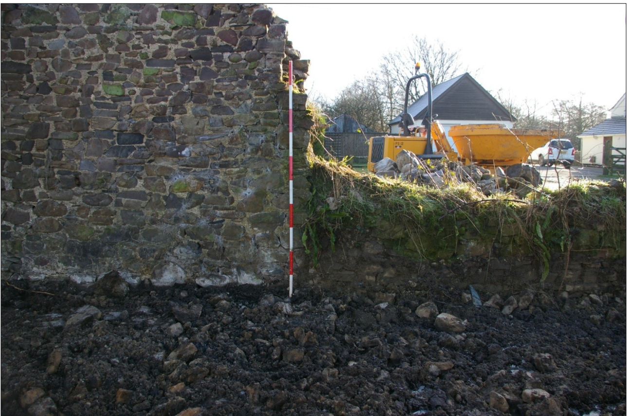
The end of the south wall with the clear build line to the west extension, now demolished; from the north (scale 2m).
