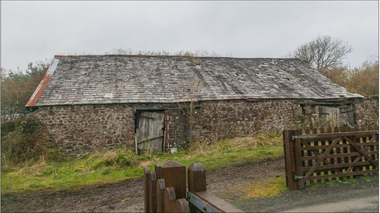
The south elevation of the warehouse; from the south-south-west (scale 2m).
