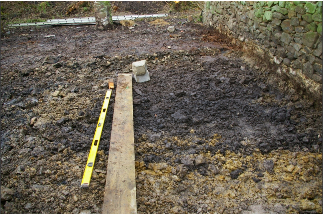
The excavated part of the floor in the west section of the barn; from the south.
