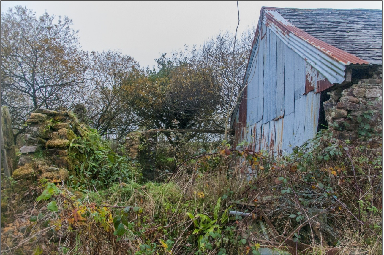
The west ruined end of the warehouse; from the south.
