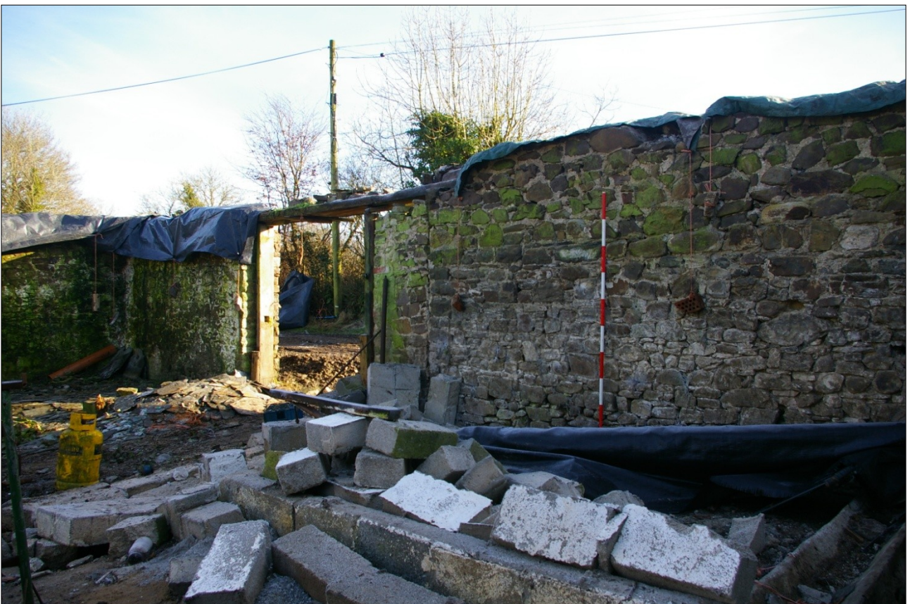
The south wall of the warehouse; from the north-west (scale 2m).
