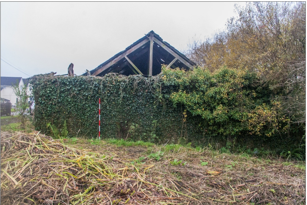
The east elevation of the warehouse; from the east (scale 2m).
