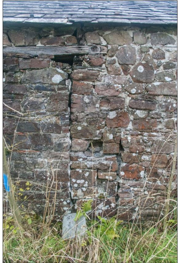
RIGHT: Detail of the blocking and two phases of build at the west doorway, south elevation; from the south.
