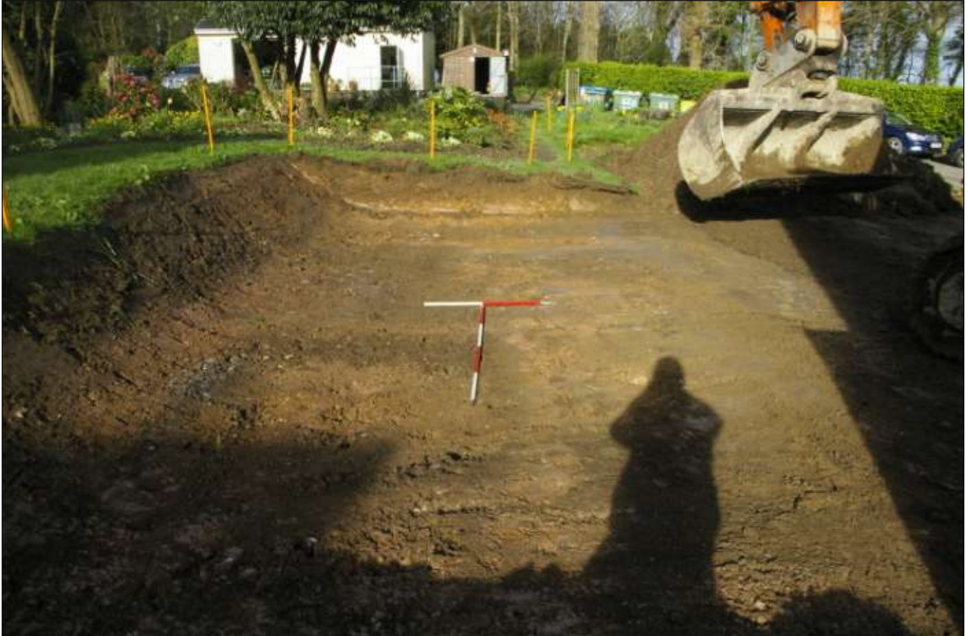
Figure 1: Area 1, post-excavation showing made-ground (to the left) over natural (right); viewed from the east (1m & 2m scales).
