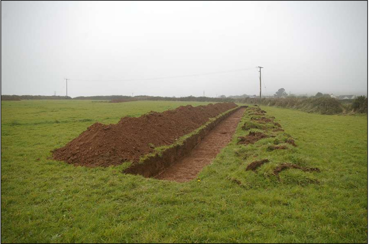
SITE SHOT SHOWING TRENCHES 1 AND 2; VIEWED FROM THE EAST (NO SCALE).
