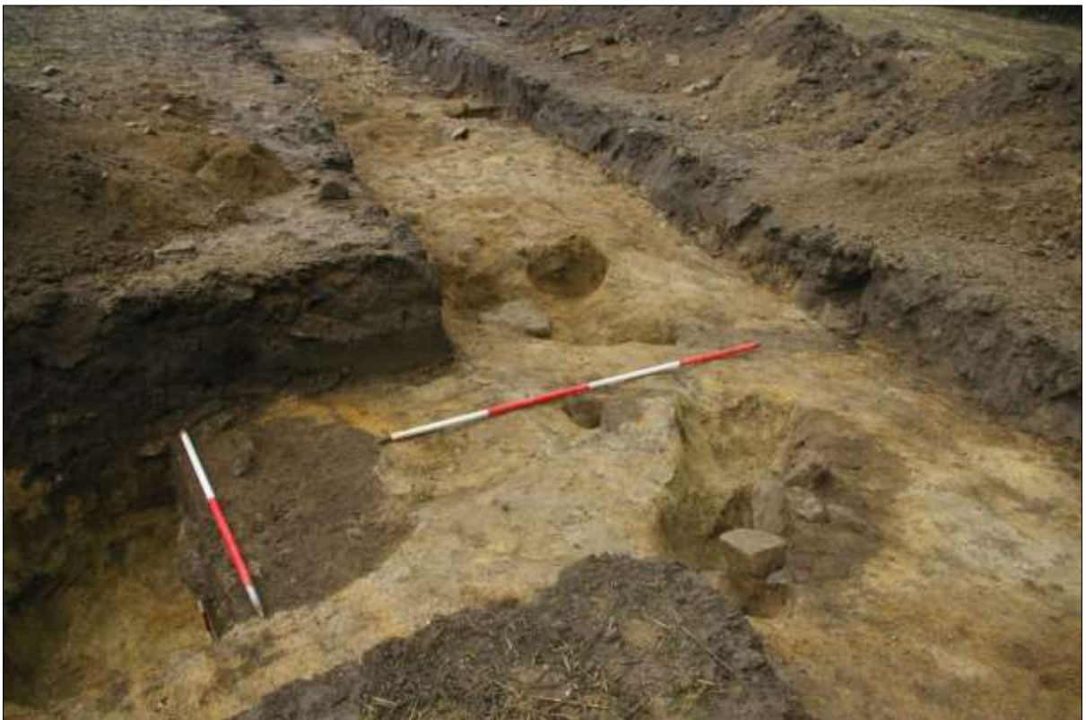
Figure 33: Postholes [1508], [1510], [1512], [1516], [1518] with pit [1615], post-excitation; viewed from the north-east (1m & 2m scales).
